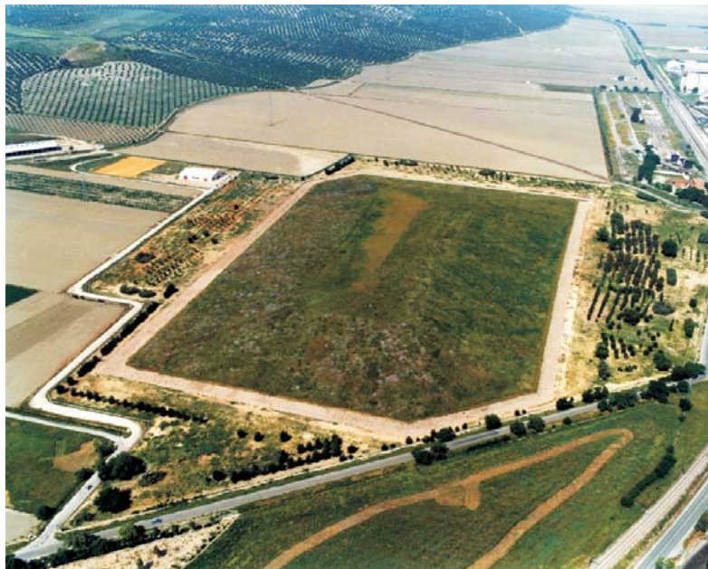
Decommissioned facilities: view of the Andújar Uranium mill.
