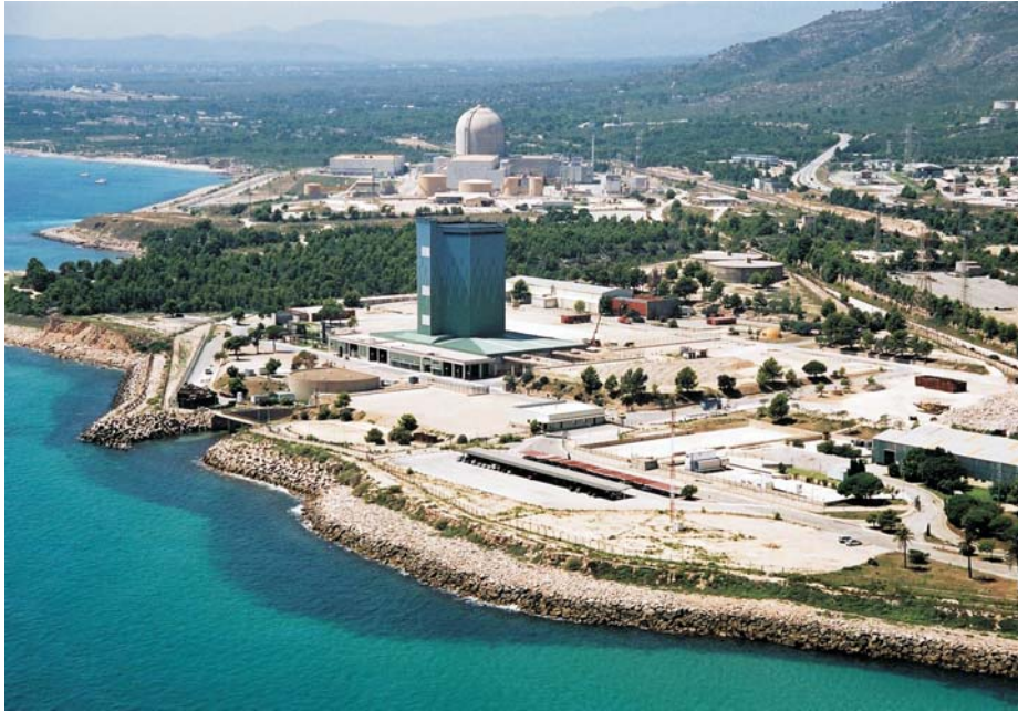
Facilities in the decommissioning phase: Vandellós I NPP.
