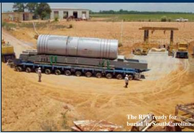
The reactor pressure vessel (RPV) was removed in May 2007 and shipped to Energy Solution's Barnwell, SC disposal facility. The shipment weighed approximately 310 tons and required a specially designed rail car.
