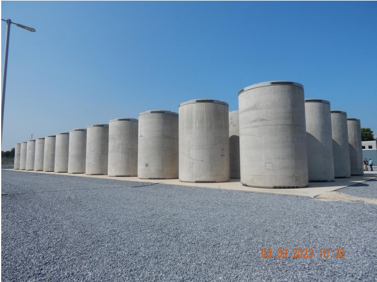
Figure 5. MAGNASTOR Dry Storage Systems at Three Mile Island Site ISFSI (Looking Southwest)
