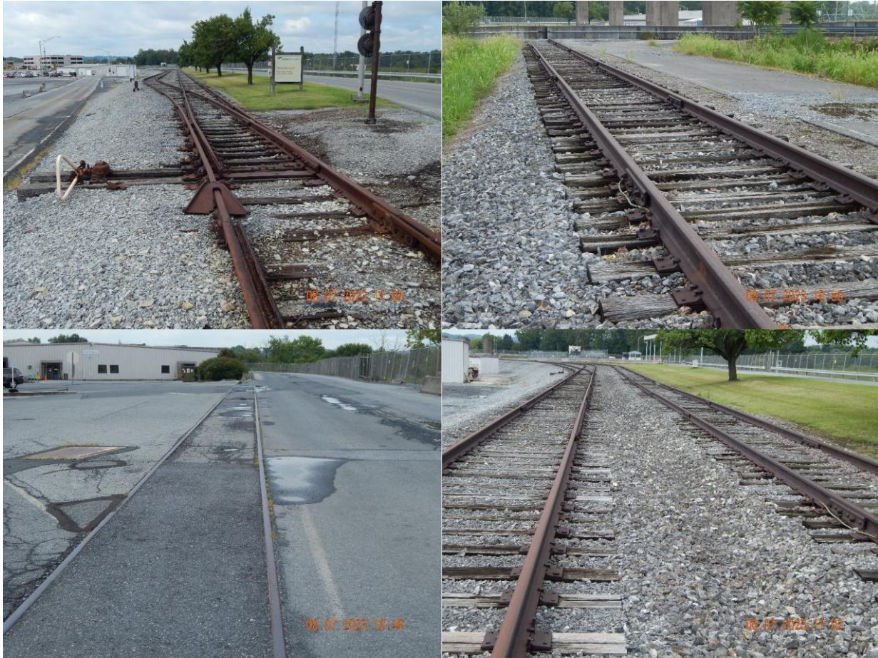
Figure 9. Views of the Three Mile Island Onsite Rail Spur
