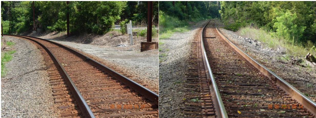
Figure 16. Norfolk Southern Rail Line at Entrance to the Three Mile Island Site Looking North (R) and South (L)
