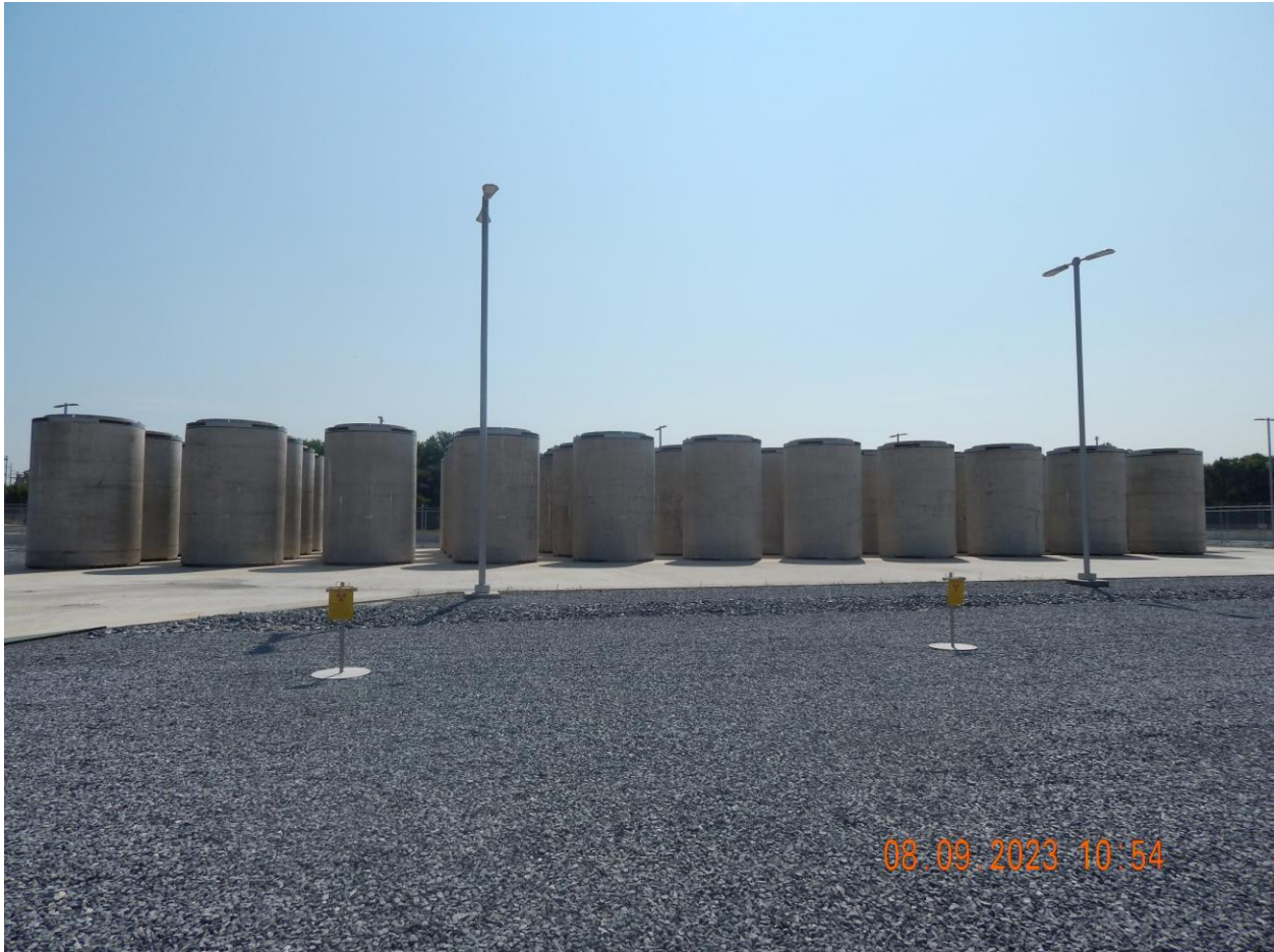
Figure 6. MAGNASTOR Dry Storage Systems at Three Mile Island Site ISFSI (Looking East)
