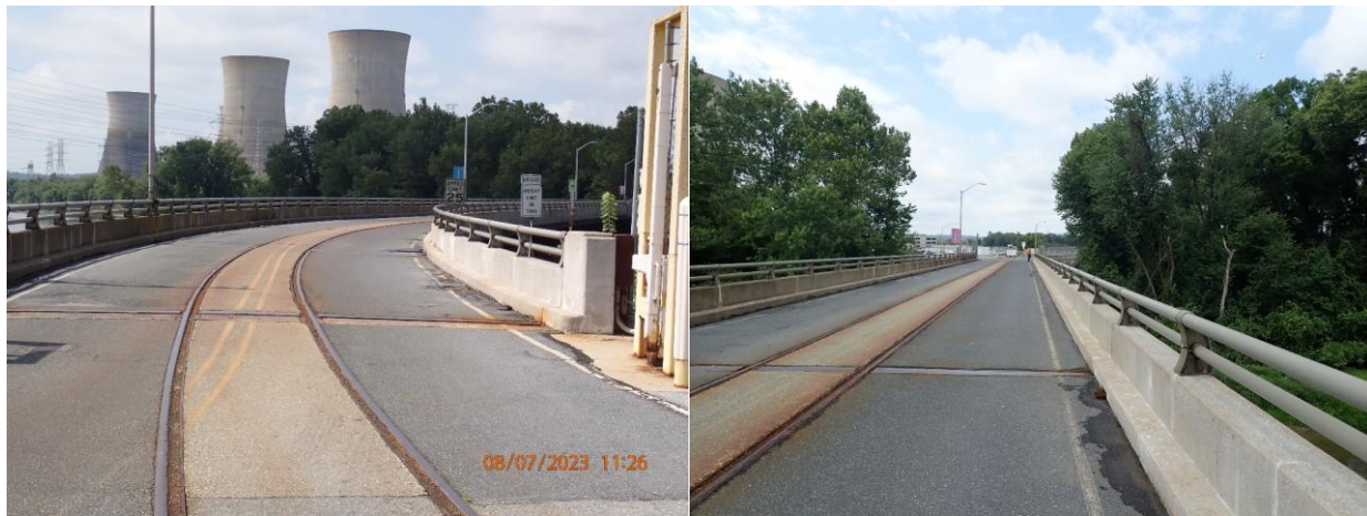
Figure 11. Three Mile Island Onsite Rail Bridge Looking Toward Site
