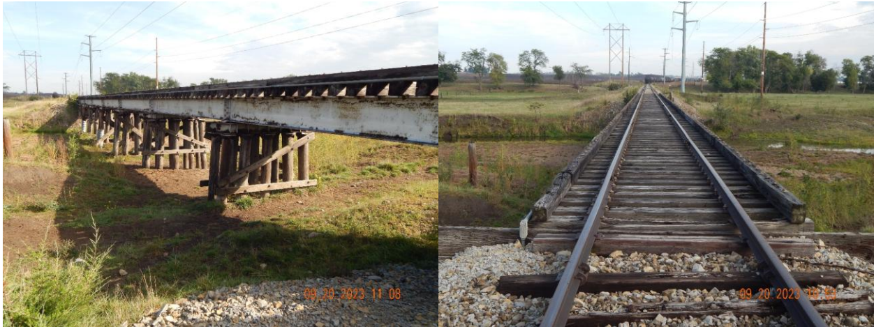
Figure 12. Trestle on Onsite Rail Spur
