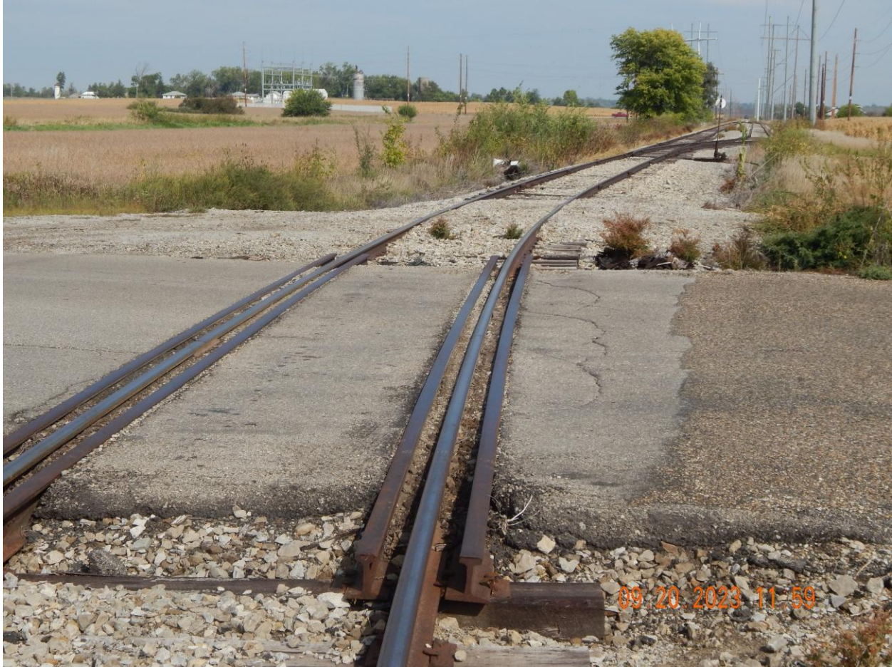
Figure 19. Duane Arnold Rail Spur at Vinton Street Grade Crossing
