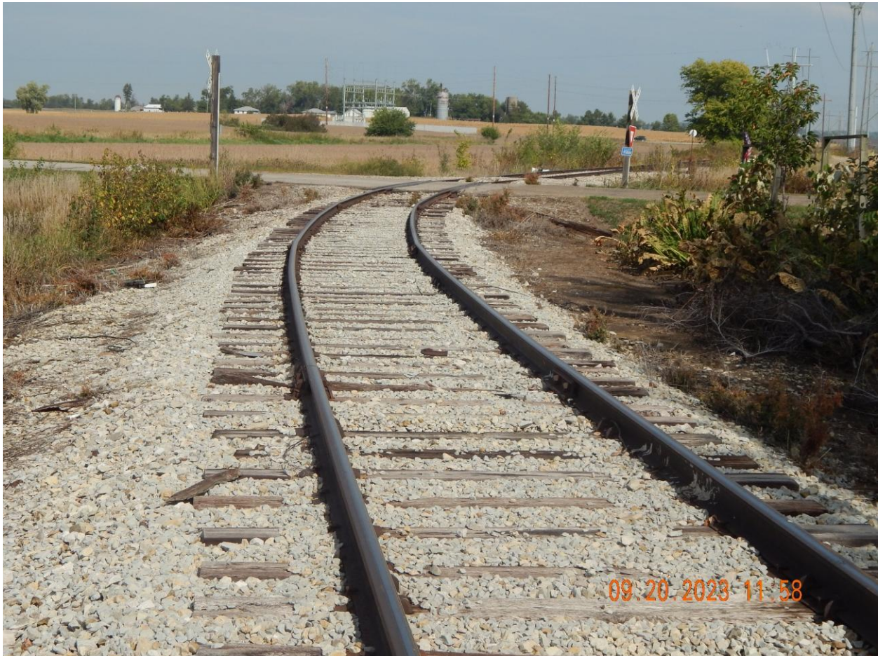
Figure 18. Duane Arnold Rail Spur Approaching Vinton Street Grade Crossing
