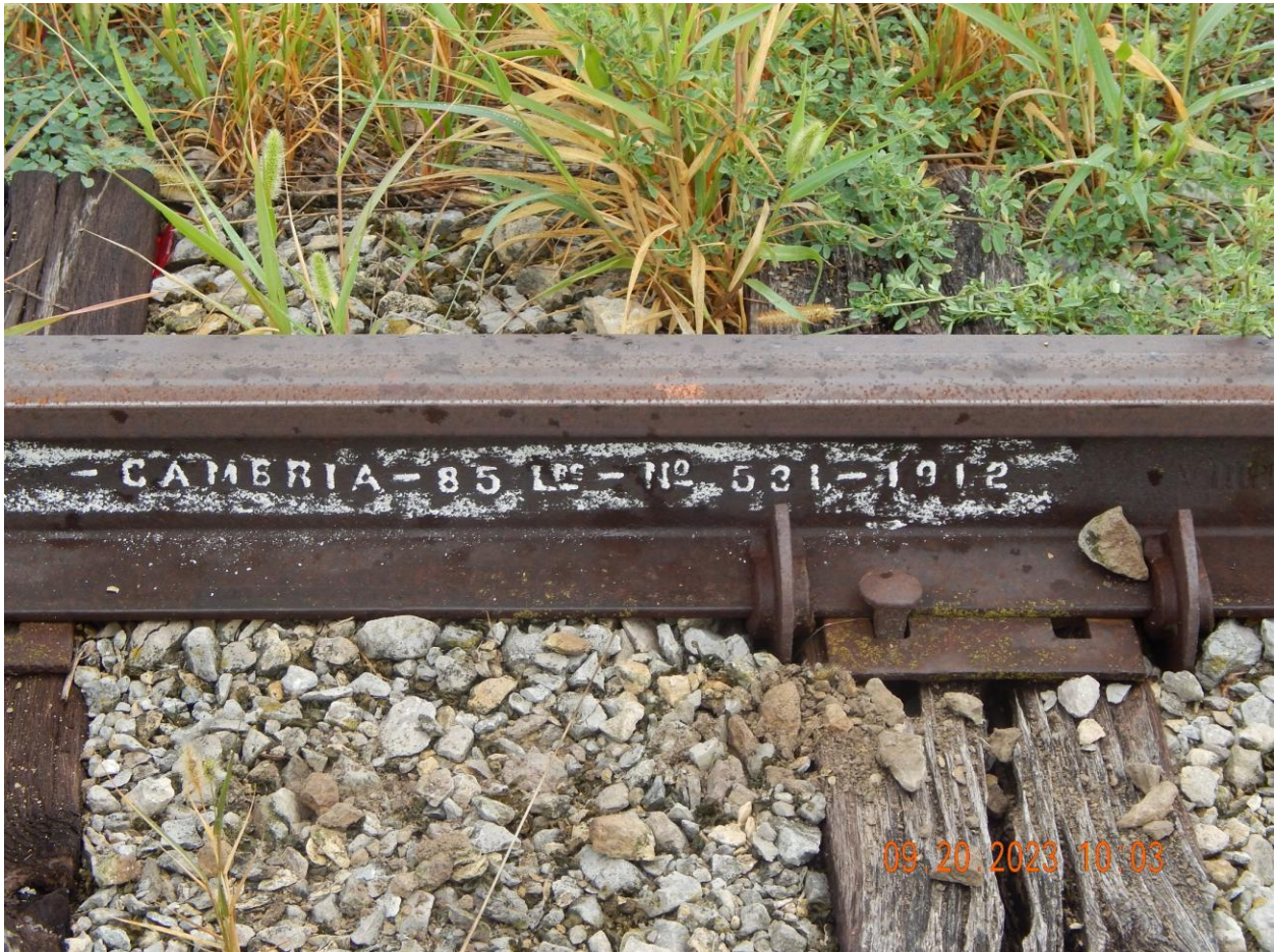
Figure 13. 85-lb Rail at Trestle on Onsite Rail Spur
