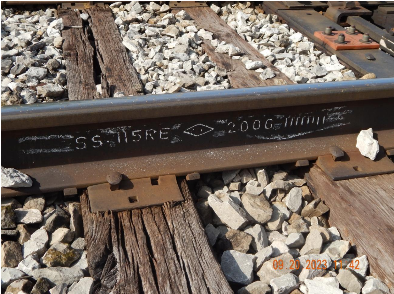
Figure 16. 115-lb Rail on CN Mainline
