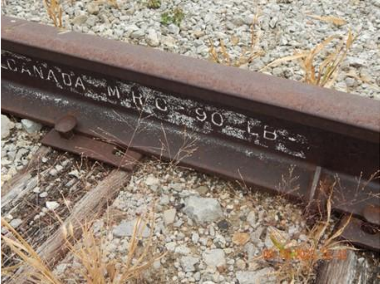
Figure 10. 90-lb Rail at Transload Locations
