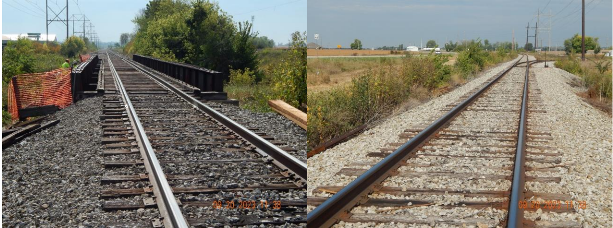
Figure 15. CN Mainline Looking Southeast (L) and Northwest (R)
