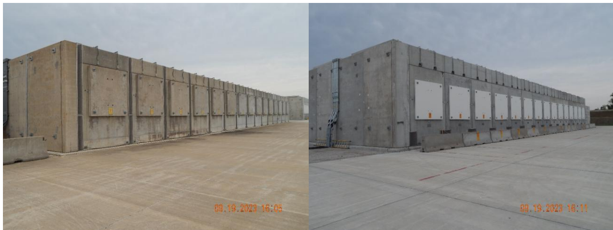
Figure 5. NUHOMS Dry Storage Systems at the Duane Arnold ISFSI
