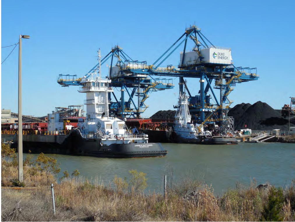
Figure 2-165. Current Barge Area Used for Unloading Coal Barges (2015)
