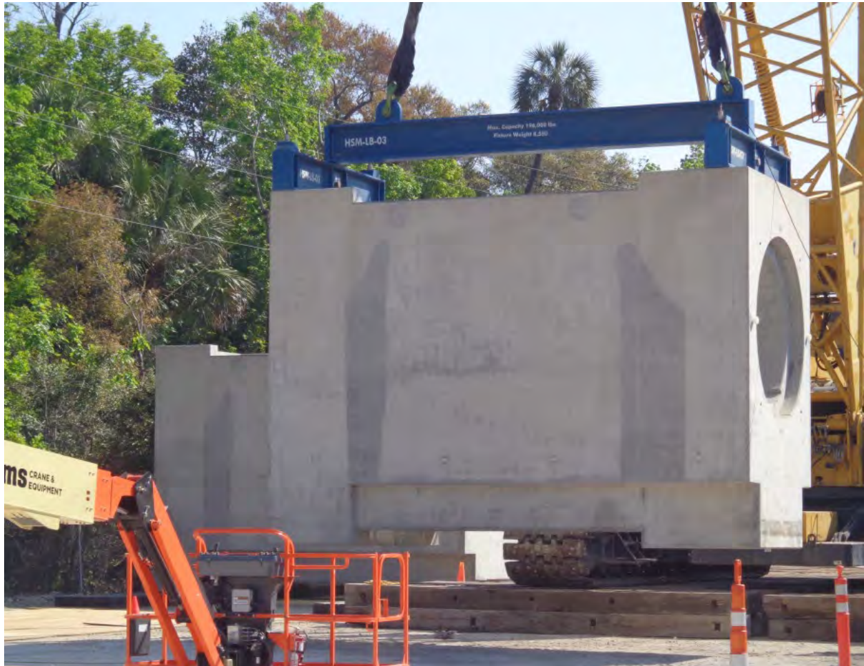
Figure 2-187. Horizontal Storage Module Being Unloaded from Railcar (2015)
