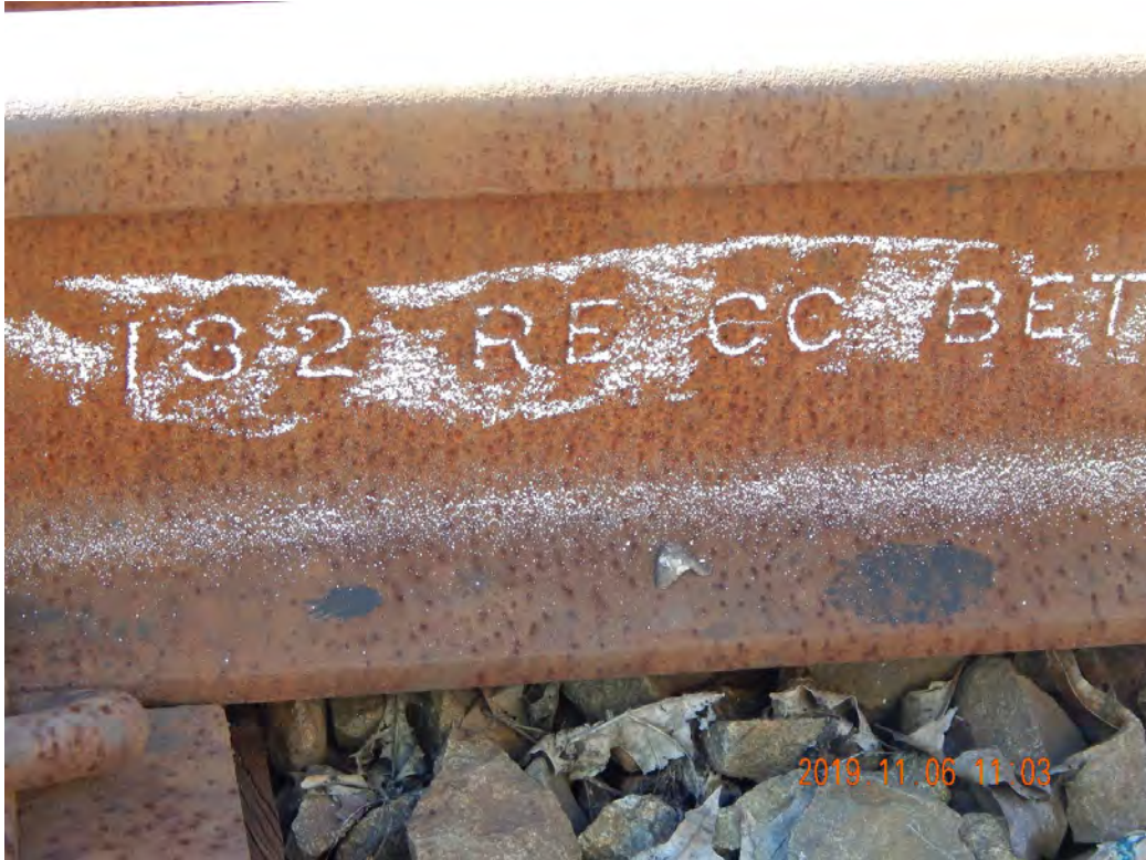
Figure 2-421. 132-lb. Rail at First Potential Rail Transload Location (2019)
