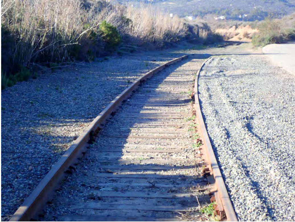
Figure 2-291. On-site Rail Spur at San Onofre Site (Looking North) (2022)
