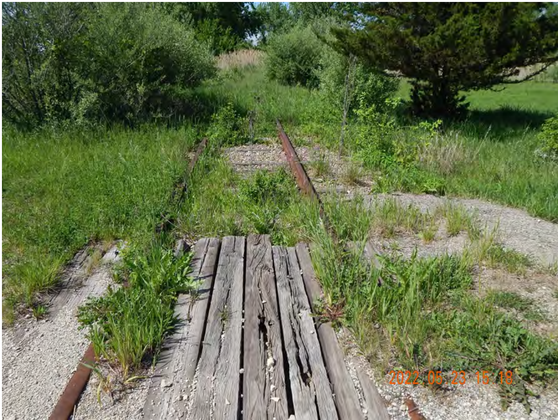
Figure 2-502. Morris Rail Spur at East Collins Road Exiting the Morris Site
