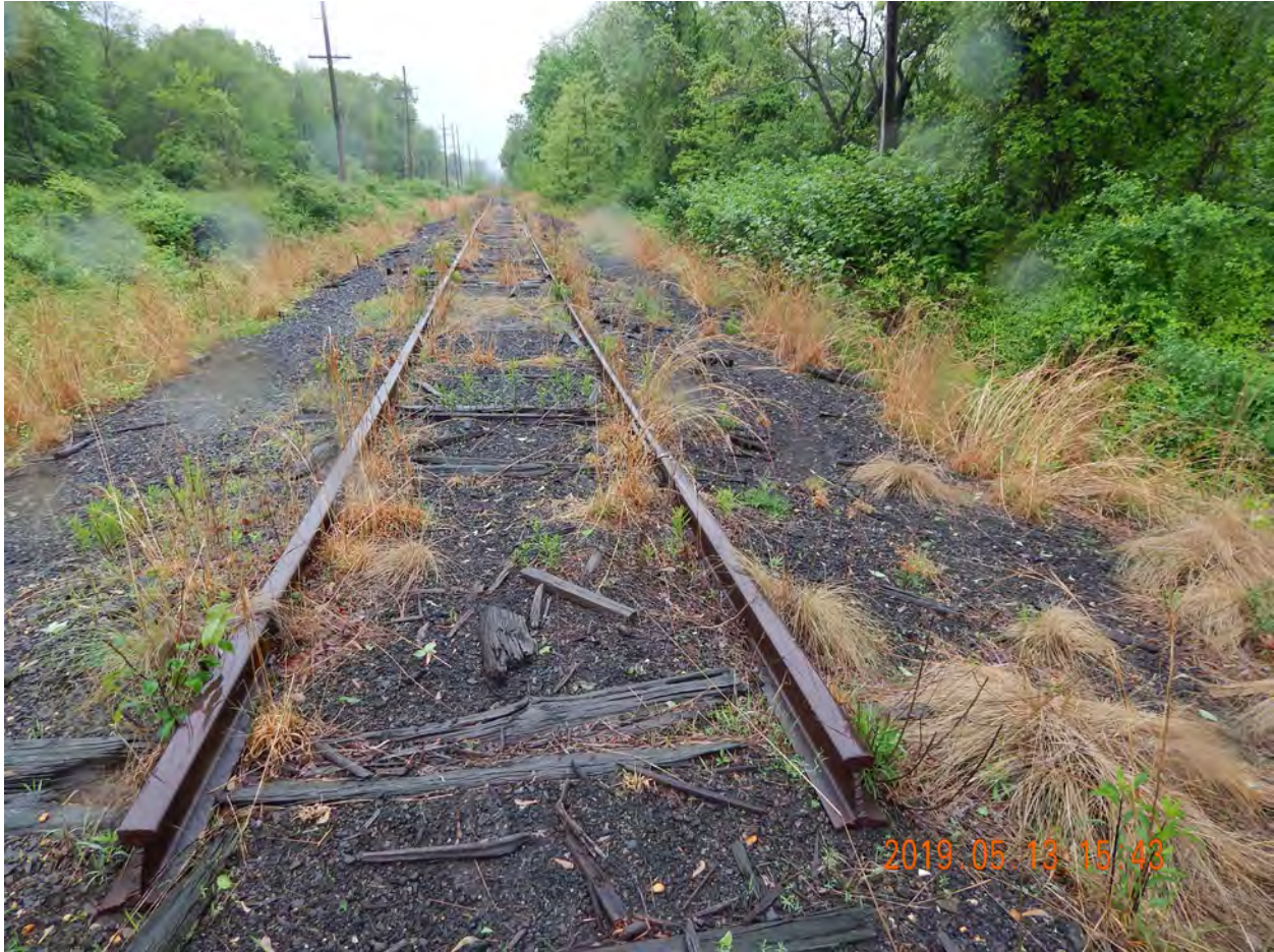
Figure 2-396. End of Rail Line in Freehold, New Jersey Looking Northwest (2019)
