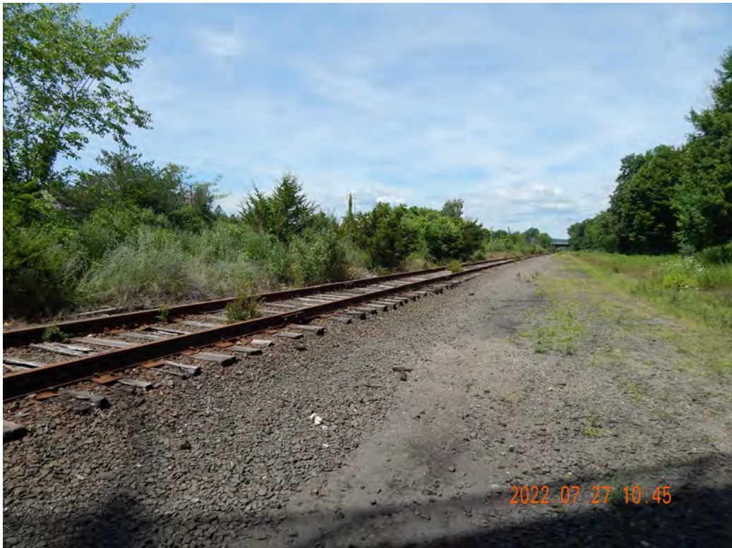
Figure 2-542. Segar Street Potential Transload Location Looking Northwest
