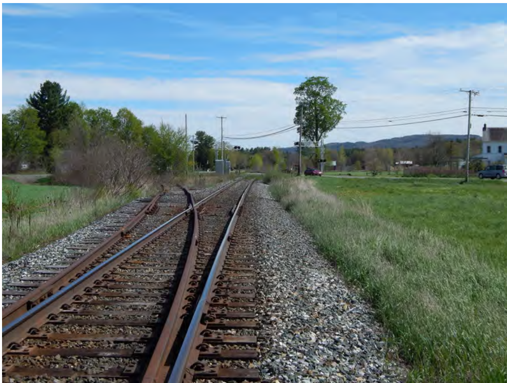
Figure 2-328. Junction of Vermont Yankee Rail Spur (Left) and New England Central Railroad Mainline (Right) Looking South (2016)
