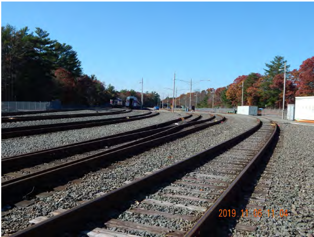
Figure 2-418. First Potential Rail Transload Location Looking West (2019)
