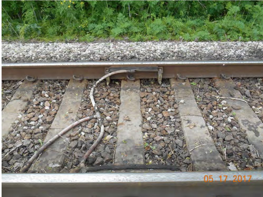
Figure 2-358. Close-up of Greaser Activators on Cargill Industrial Spur (2017)
