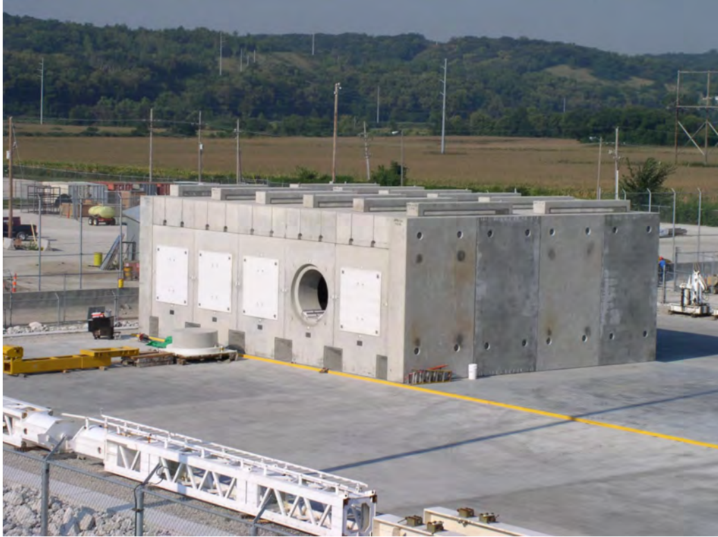
Photo courtesy of Fort Calhoun
