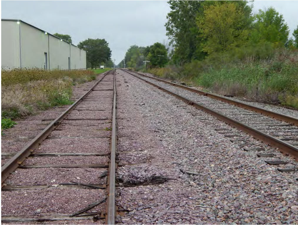
Figure 2-217. Potential Bellevue Transload Location (Looking North) (2014)
