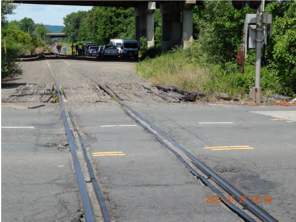
Figure 2-539. Segar Street Potential Transload Location Looking Northwest
