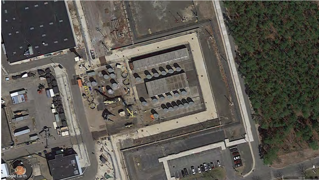
Figure 2-381. Aerial View of Oyster Creek Independent Spent Fuel Storage Installation (Google 2022)
