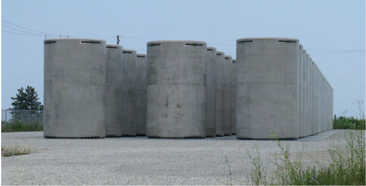
Figure 2-139. Vertical Concrete Storage Casks Staged at Zion (2013)
