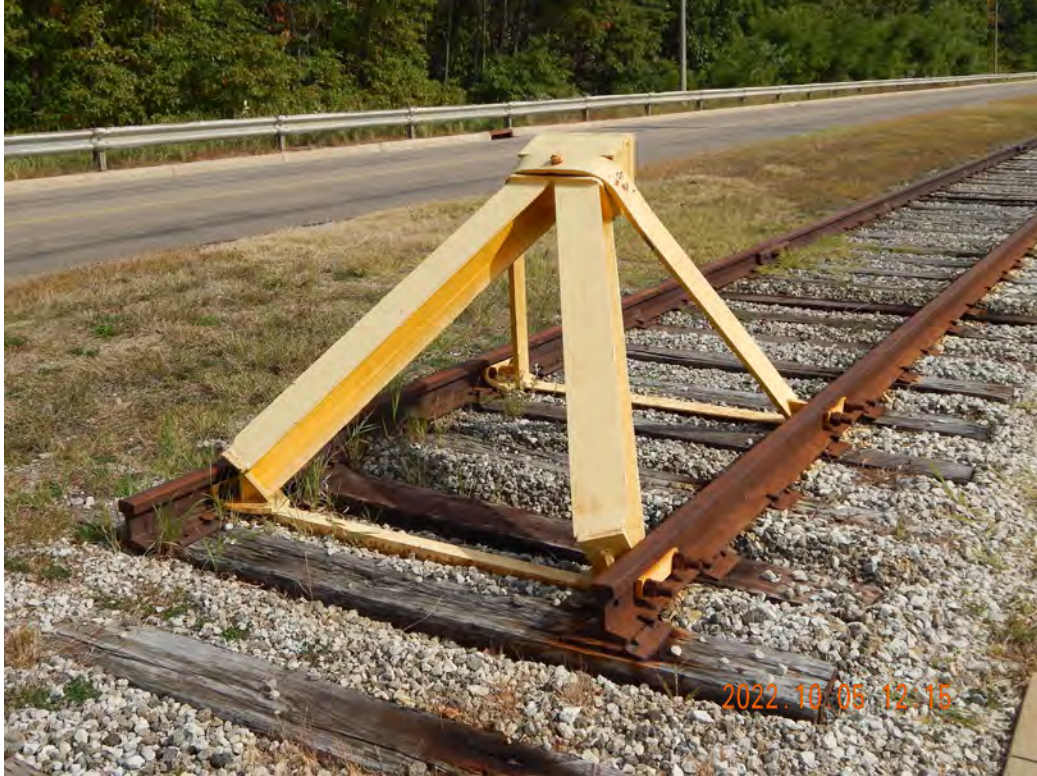
Figure 2-612. Bumping Post on DC Cook Rail Spur
