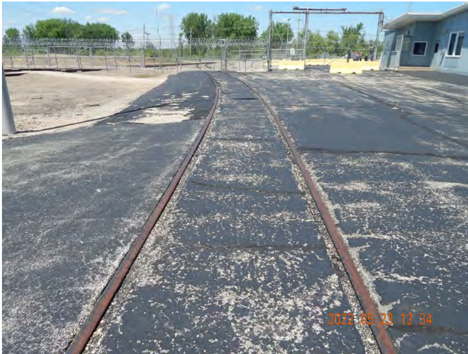
Figure 2-494. Railroad Tracks into the Cask Receiving Area (Looking North)
