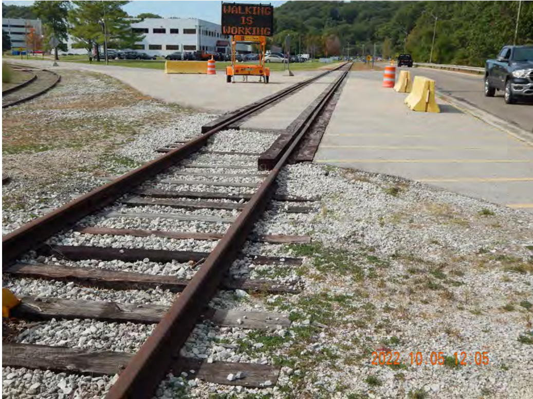
Figure 2-610. DC Cook Rail Spur Looking West
