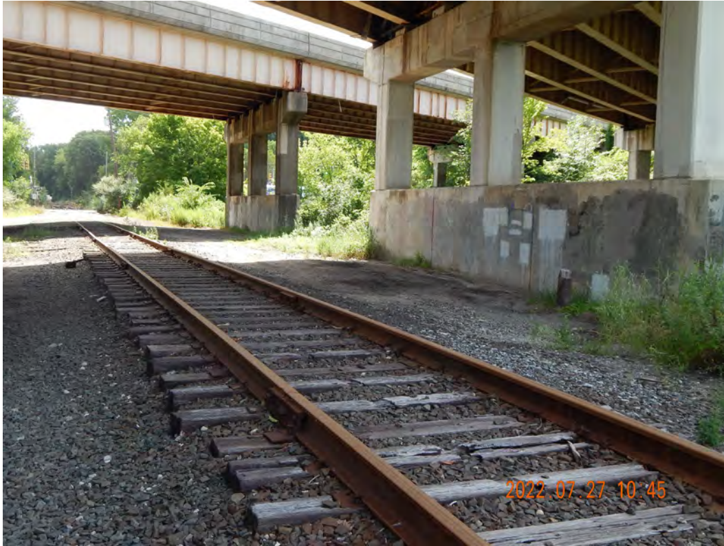
Figure 2-543. Segar Street Potential Transload Location Looking Northwest Under U.S. 7 Overpass
