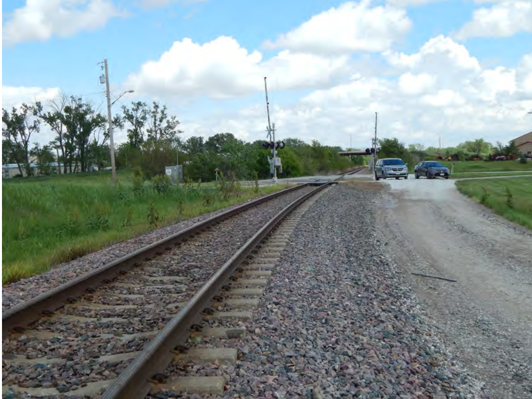
Figure 2-354. Track at Entrance to Cargill Industrial Spur (Looking North) (2017)
