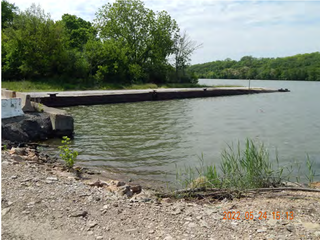
Figure 2-473. Dresden Barge Area Looking Northwest
