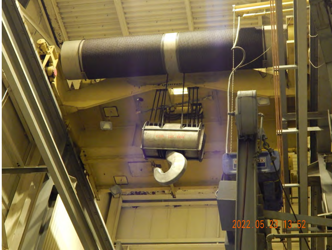
Figure 2-484. 125-Ton Crane at the Morris Site
