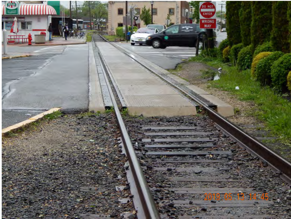
Figure 2-394. Rail Line in Freehold, New Jersey Looking Northwest (2019)
