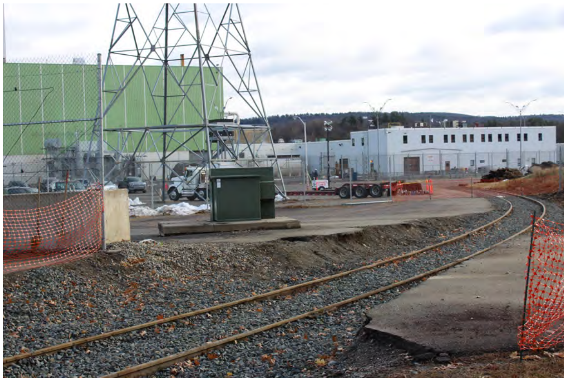
Photo courtesy of Vermont Yankee
