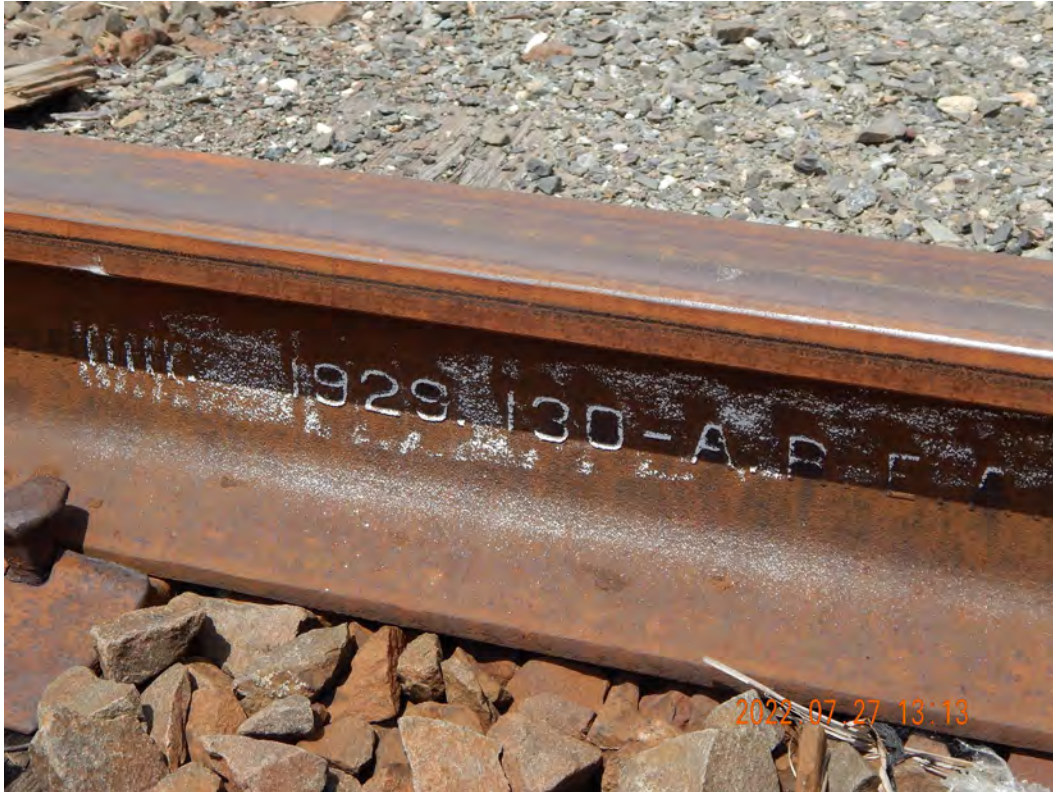
Figure 2-547. 130-lb. Rail at Agriventures Agway Potential Transload Location
