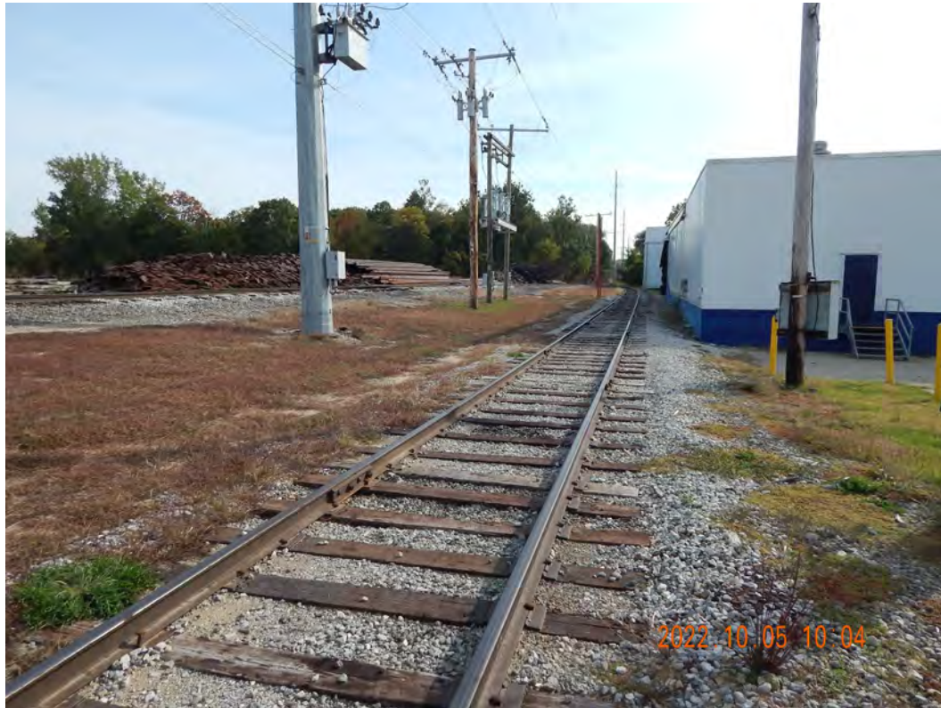
Figure 2-583. Lineage Logistics Potential Transload Location Looking East
