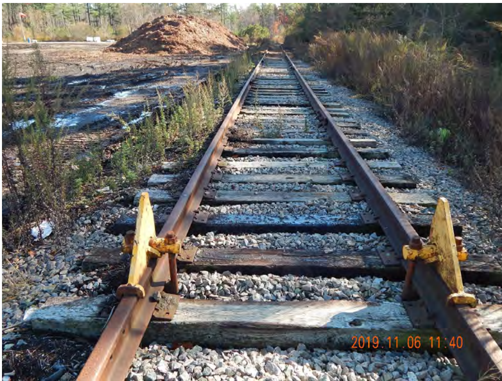
Figure 2-431. End of Industrial Spur at Second Potential Rail Transload Location (2019)
