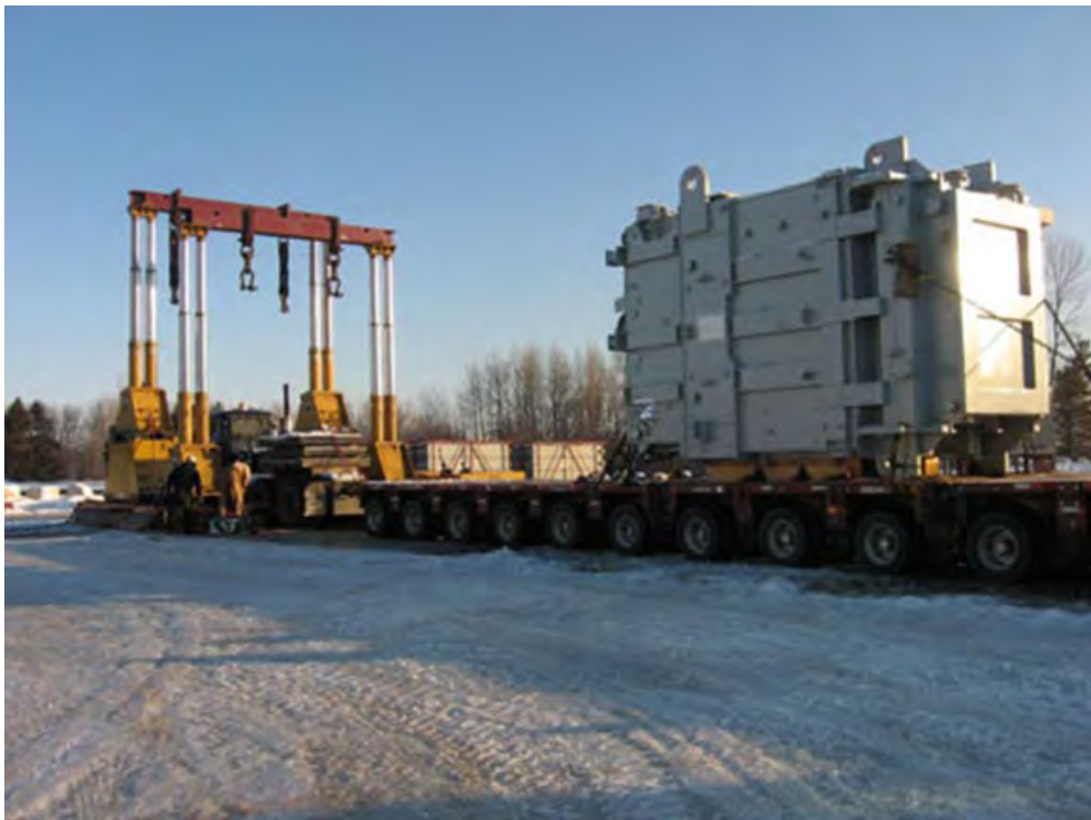
Figure 2-213. Gantry System Used to Transfer Transformers from Railcars to Goldhofer Trailers (2008)
