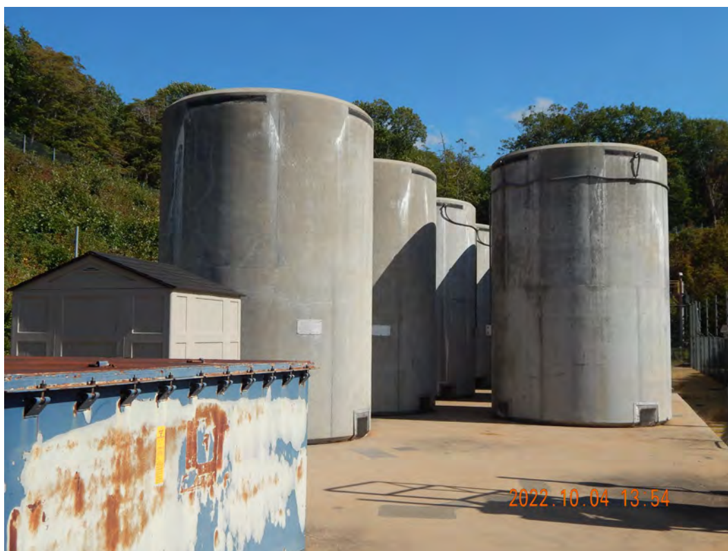
Figure 2-572. VSC-24 Dry Storage Systems at the Original ISFSI Looking East
