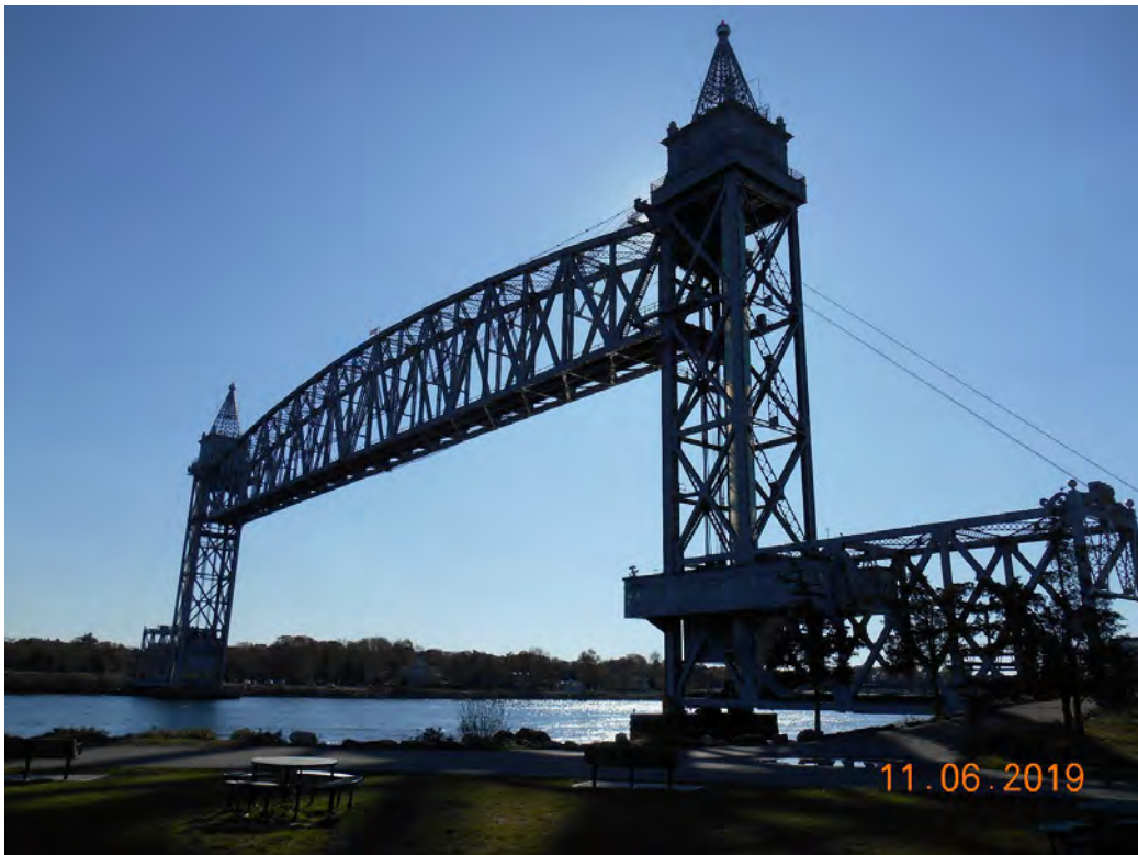
Figure 2-438. Cape Cod Canal Railroad Bridge (2019)
