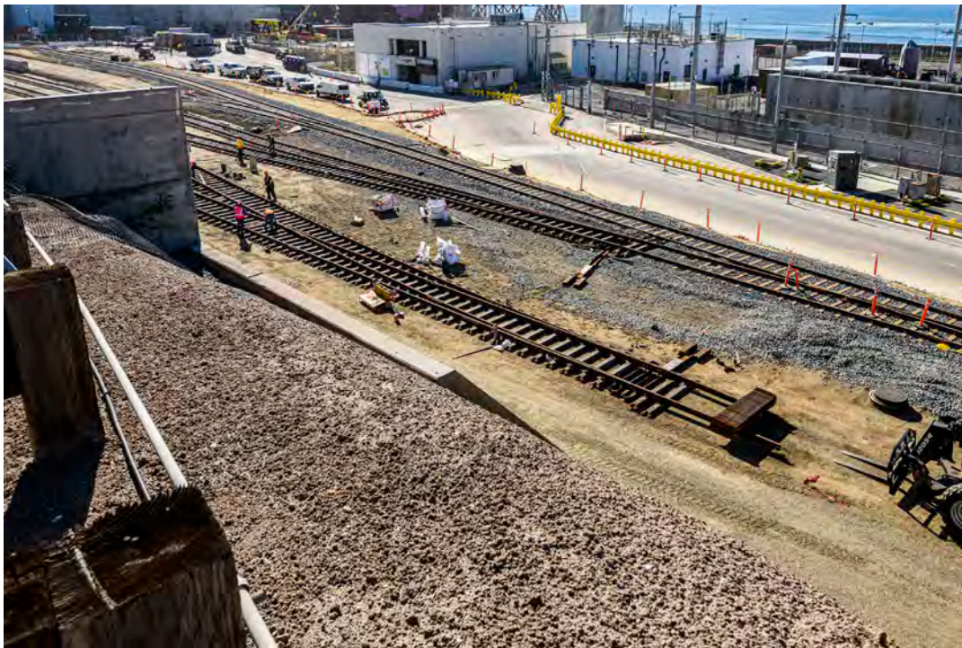
Figure 2-284. Expansion of On-site Rail Spur (Looking West) (2022)
