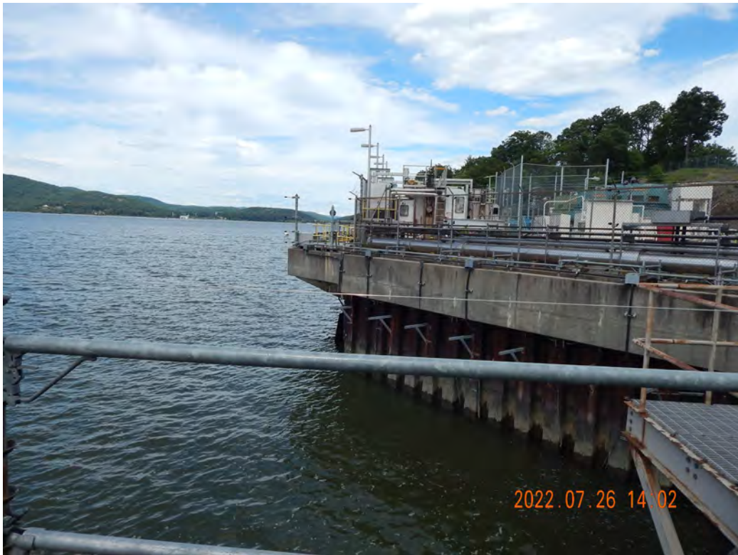
Figure 2-522. Indian Point Barge Area Looking North
