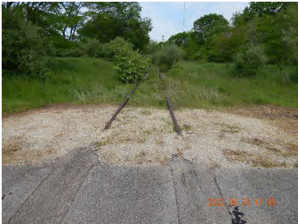
Figure 2-453. Rail Spur at Lock Road Looking East
