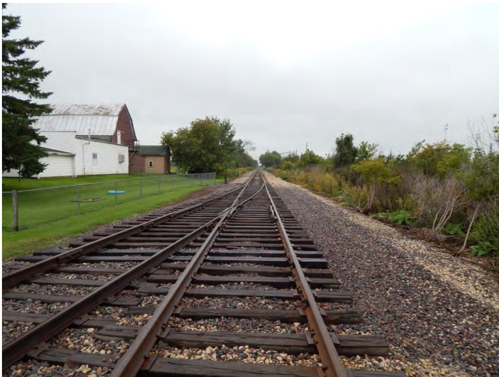
Figure 2-211. Potential Luxemburg Transload Location Further Down Track (Looking West) (2014)
