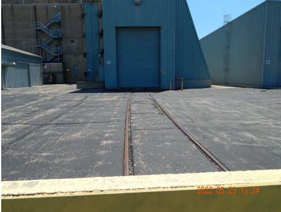
Figure 2-493. Railroad Tracks into the Cask Receiving Area (Looking South)
