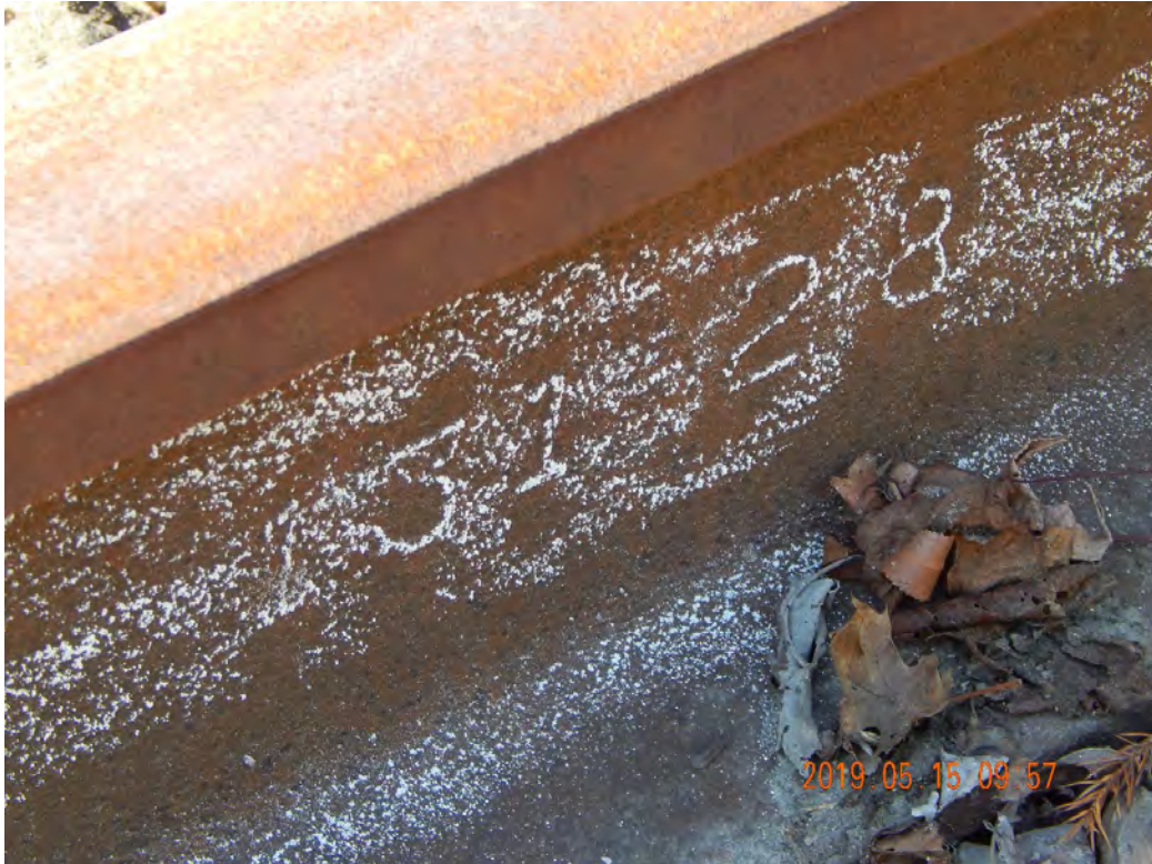
Figure 2-401. 131-lb. Rail at Morrisville Railyard (2019)
