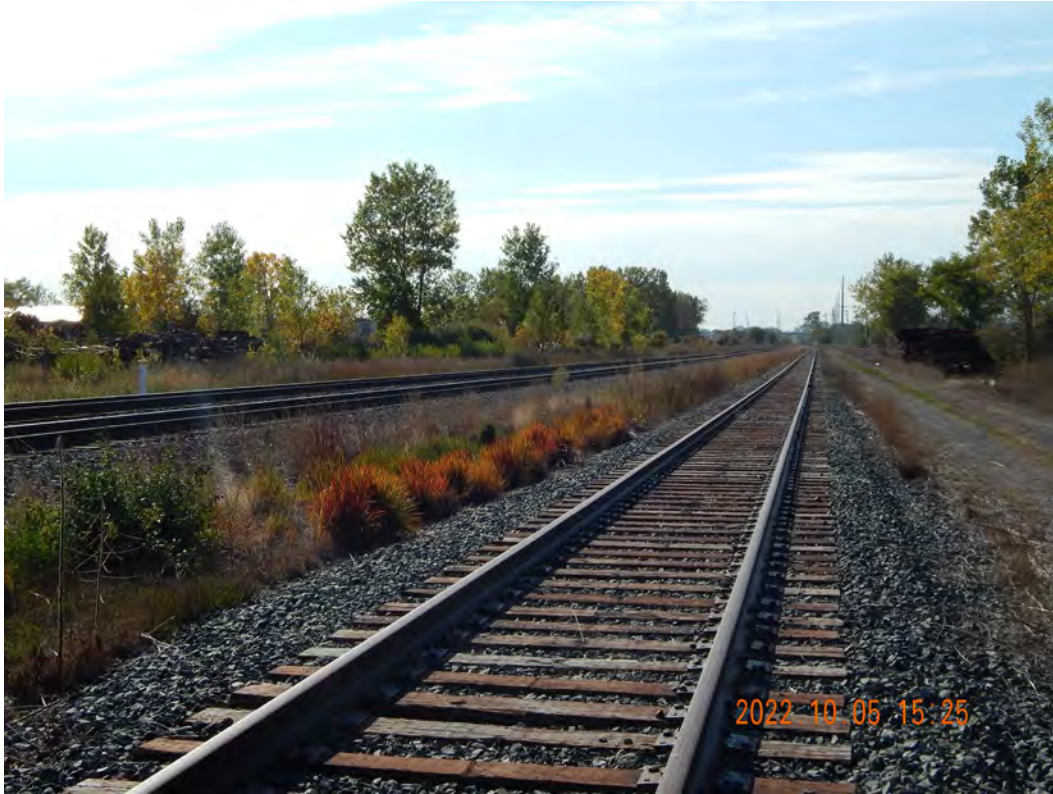
Figure 2-600. Abandoned CSX Railyard Potential Transload Location Looking West
