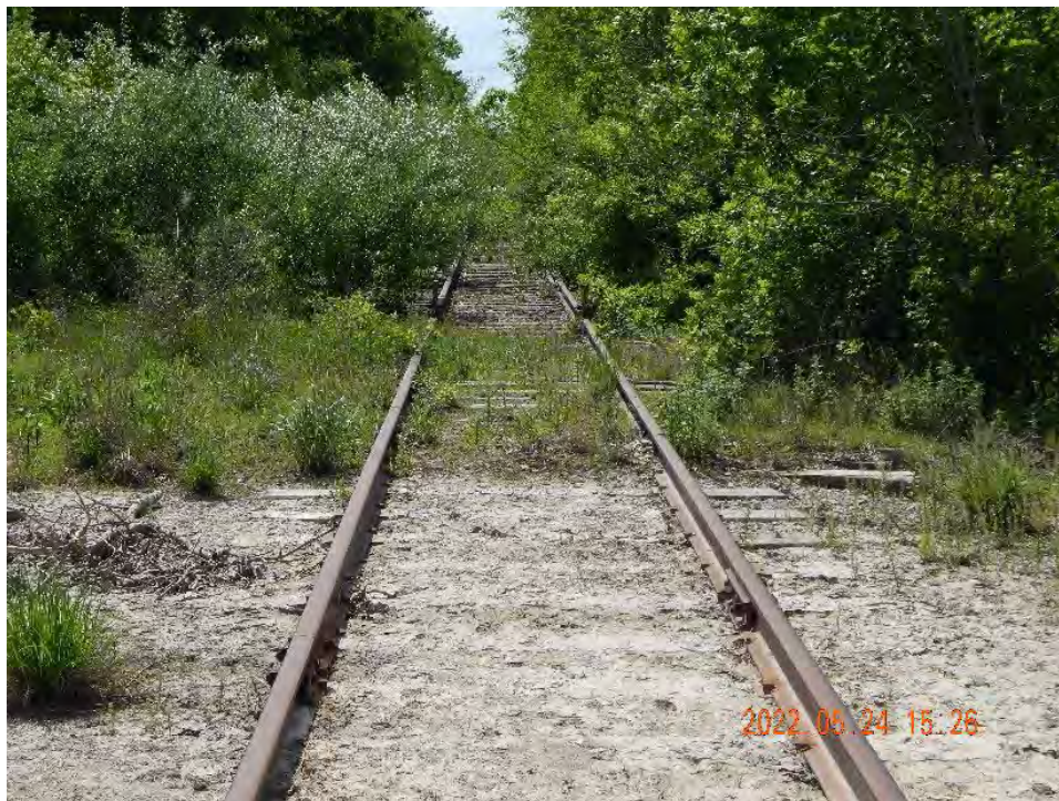
Figure 2-451. Rail Spur at the Dresden Site Looking West
