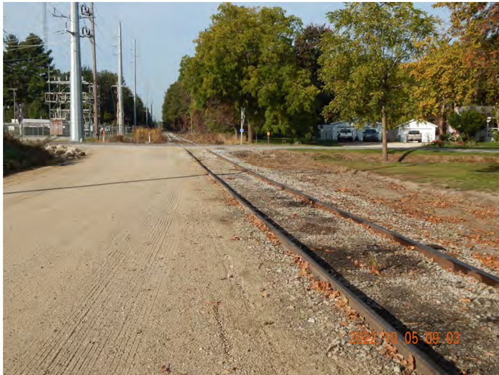
Figure 2-579. Paw Paw River Produce Potential Transload Location Looking West
