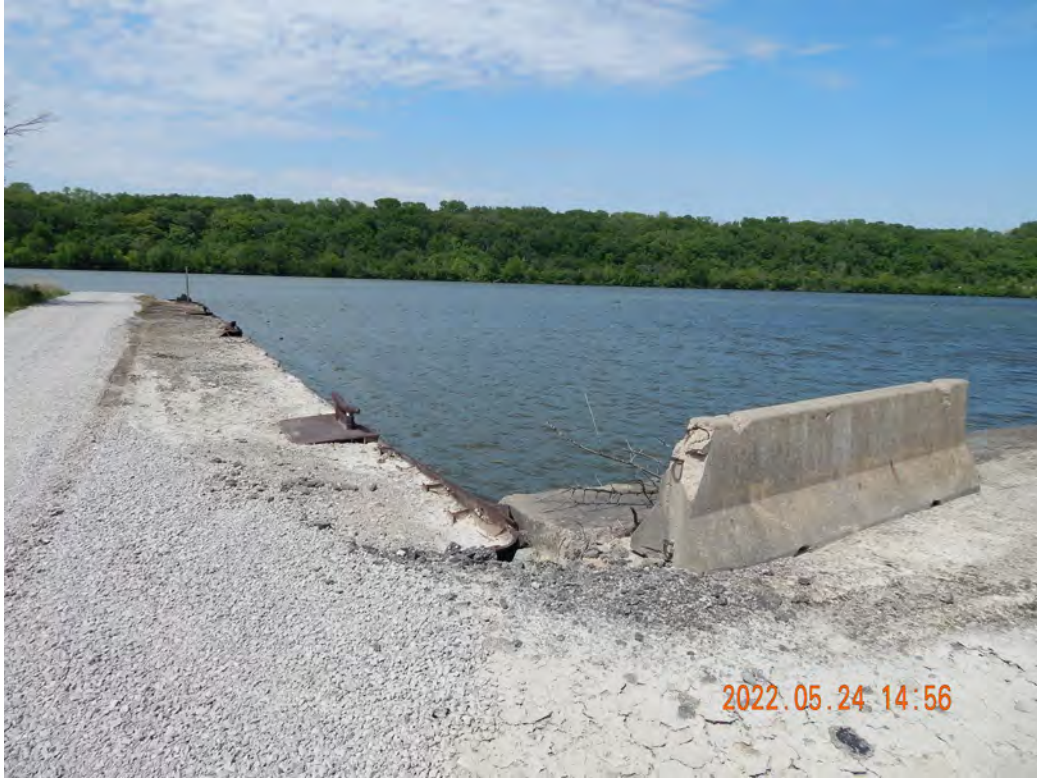
Figure 2-471. Dresden Barge Area Looking North
