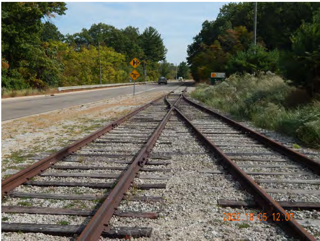
Figure 2-611. DC Cook Rail Spur Looking East
