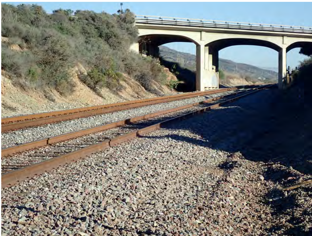
Figure 2-294. BNSF Mainline Looking South (2022)
