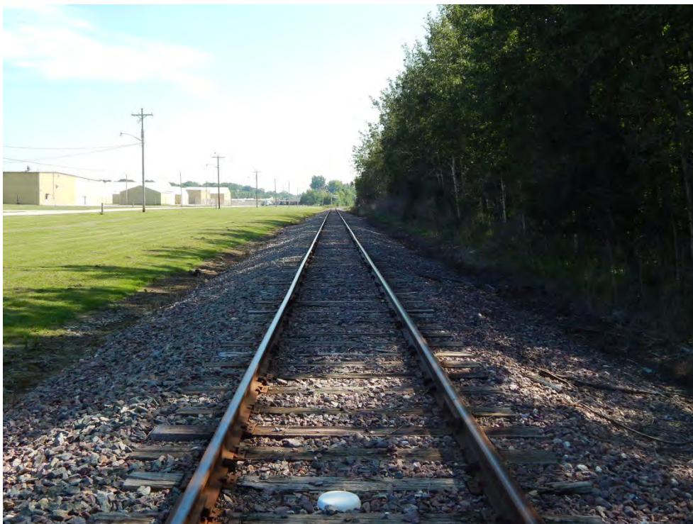
Figure 2-239. Potential Rockwood Spur at the Manitowoc Airport Transload Location (Looking South) (2014)
