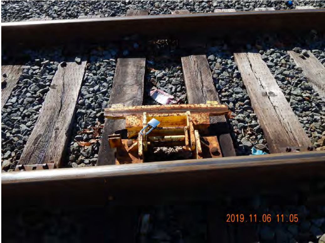
Figure 2-419. Derailer at First Potential Rail Transload Location (2019)
