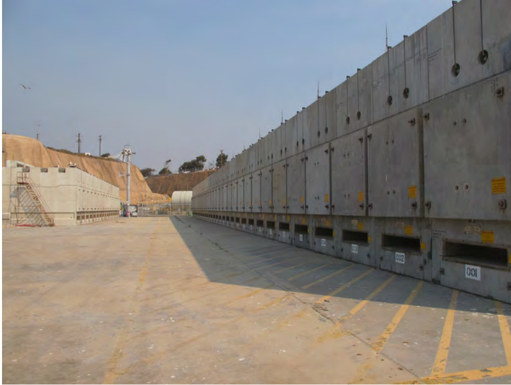
Figure 2-277. Close-up View of Original San Onofre Independent Spent Fuel Storage Installation (2018)
