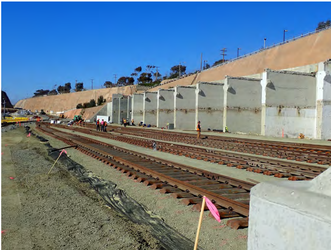
Figure 2-286. Expansion of On-site Rail Spur (Looking North) (2022)
