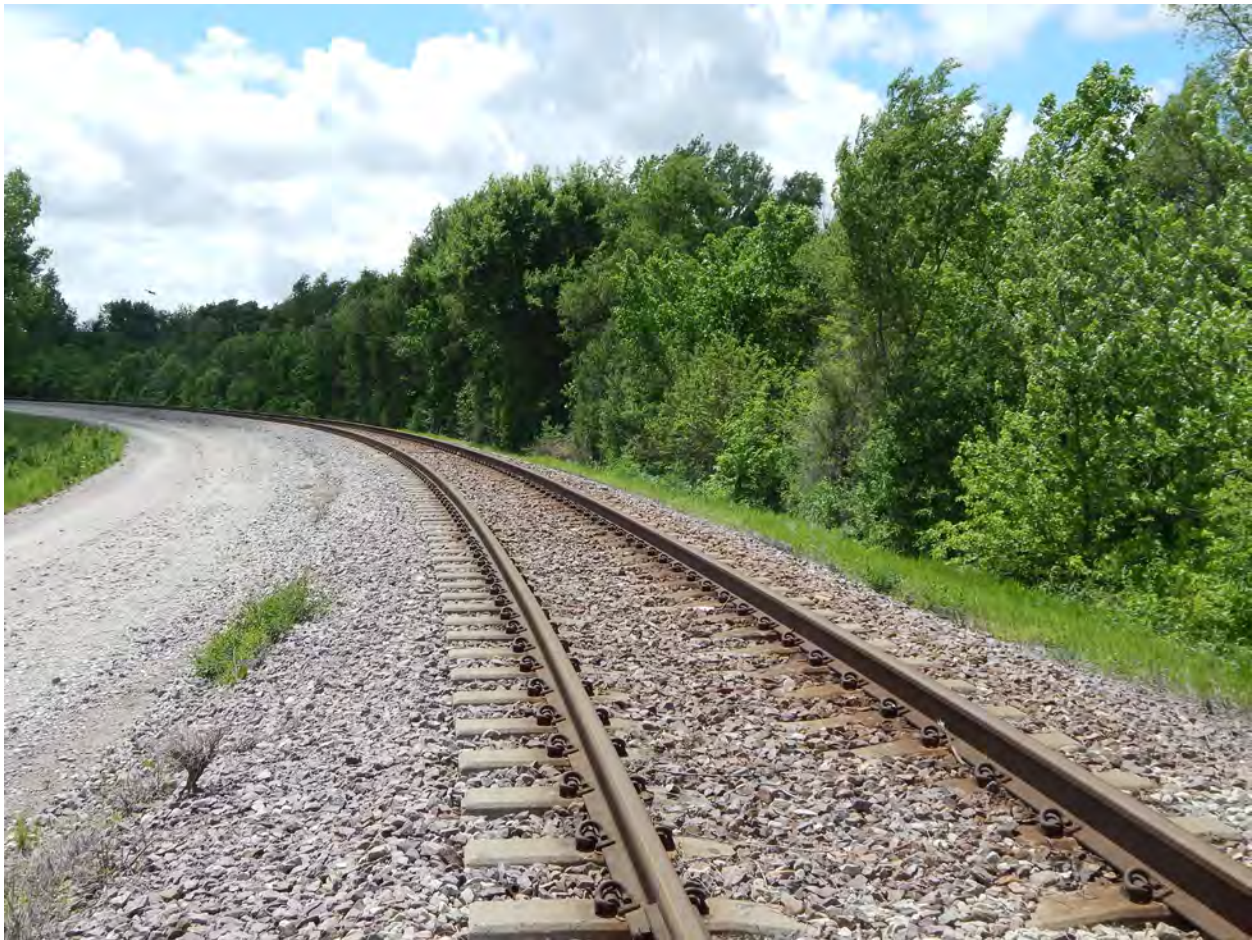
Figure 2-353. Track at Entrance to Cargill Industrial Spur (Looking South) (2017)
