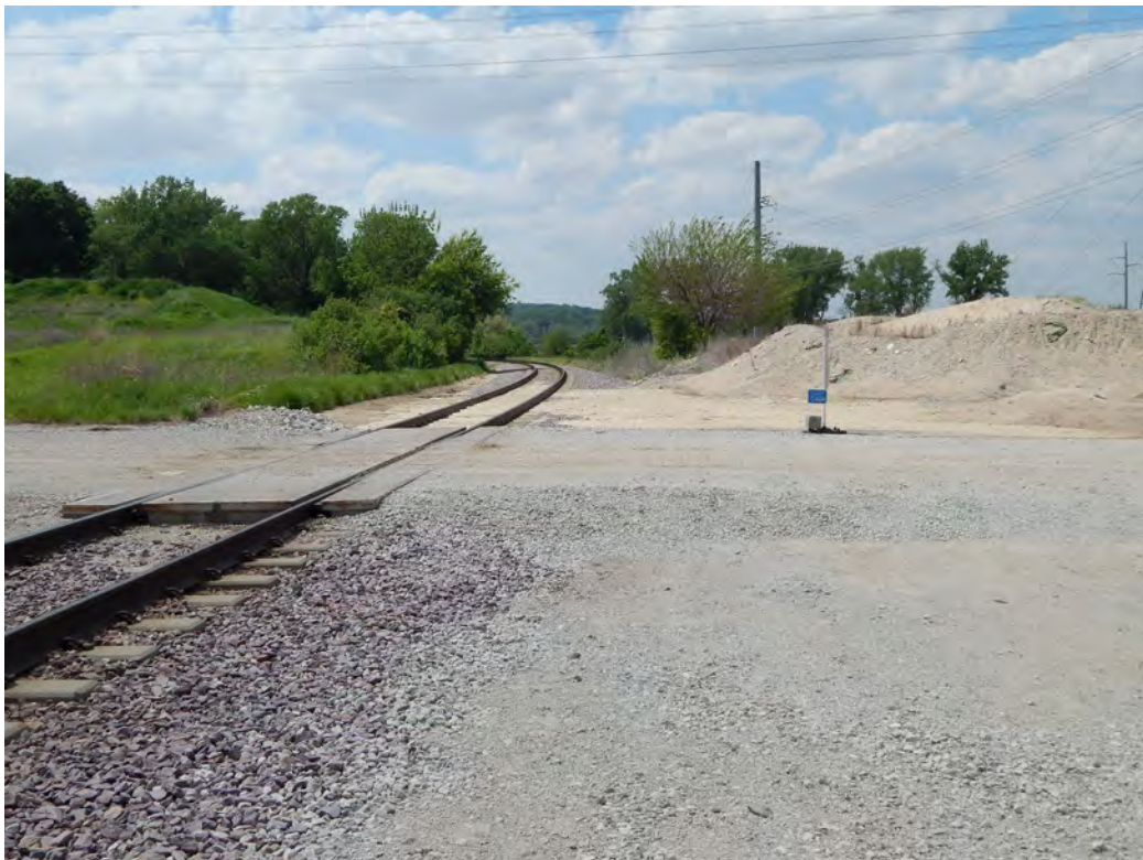
Figure 2-368. Current Condition of Transload Location (2017)
