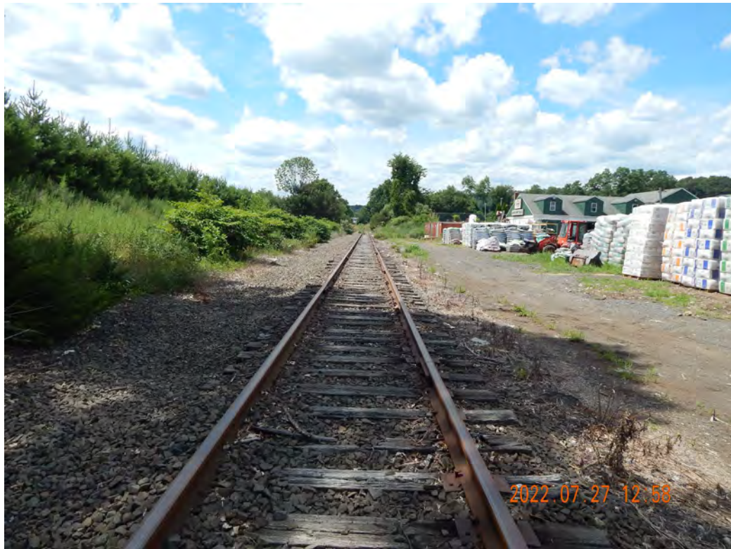
Figure 2-546. Agriventures Agway Potential Transload Location Looking Northwest
