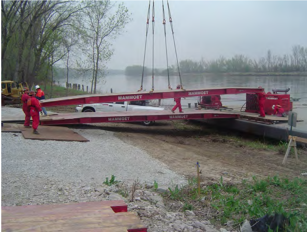
Photo courtesy of Fort Calhoun
