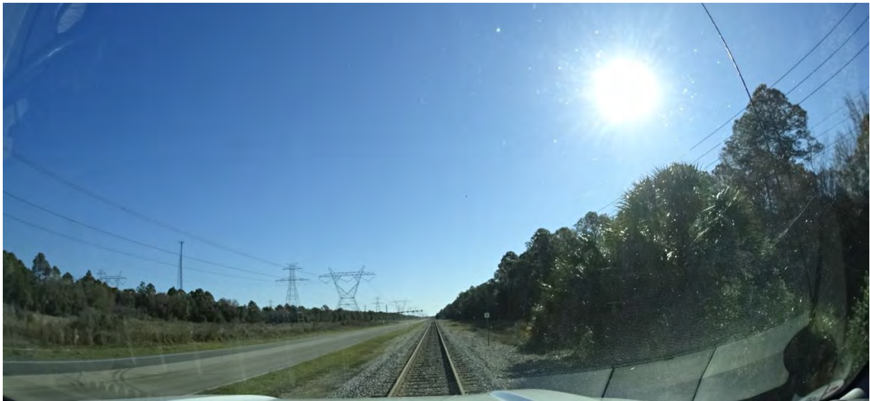
Figure 2-163. On-site Industrial Rail Spur Approaching U.S. Highway 19 from the West (2015)
