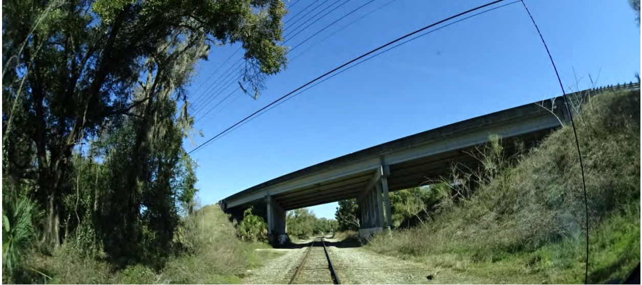
Figure 2-171. Highway Bridge over Florida Northern Railroad (2015)
