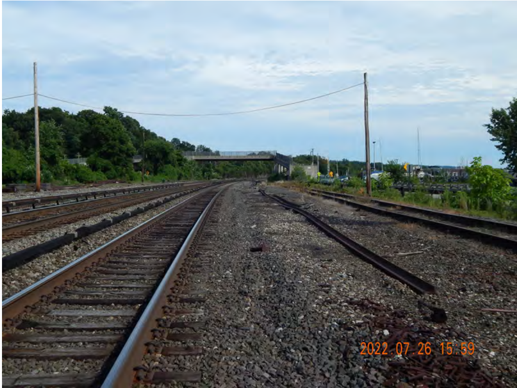
Figure 2-557. Croton Railyard Potential Transload Location Looking Southeast
