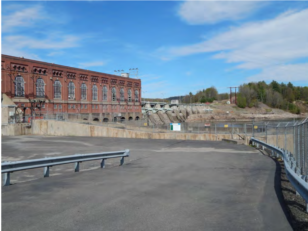
Figure 2-316. Vernon Dam and Hydroelectric Station (2016)
