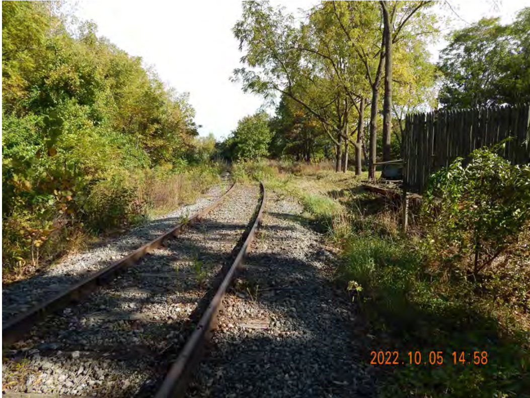
Figure 2-591. Rail Spur Near NoBo Marijuana Cultivation Facility Potential Transload Location Further Down Spur Looking Towards CSX Mainline
