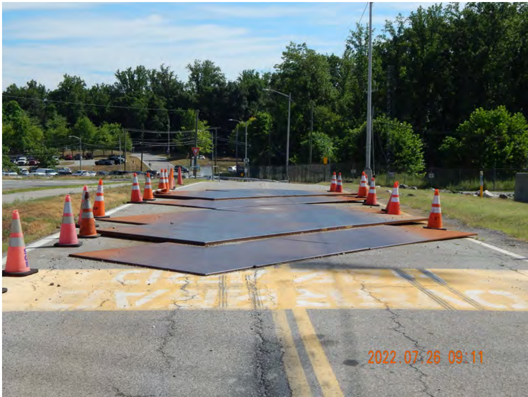
Figure 2-526. Air Bridge Over 26-inch and 30-inch Gas Lines Looking North
