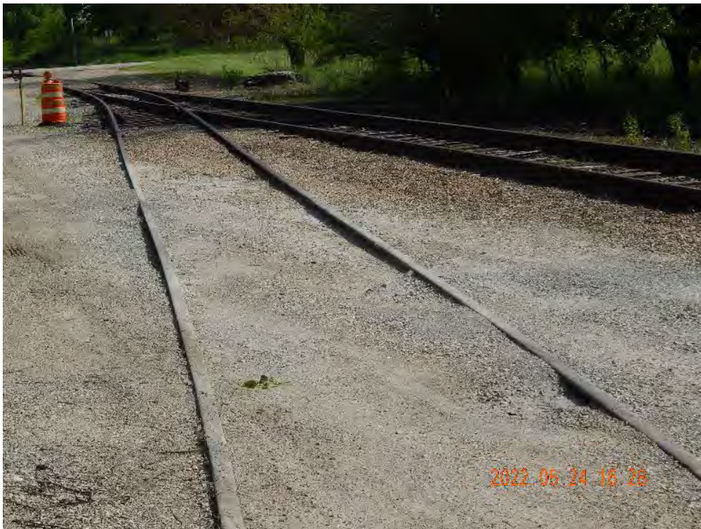
Figure 2-455. Rail Spur and Canadian National Illinois Subdivision Rail Line (Looking Southwest)
