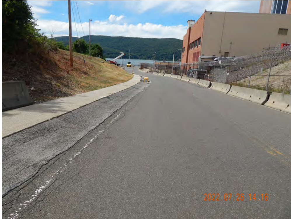
Figure 2-523. Indian Point Barge Area Access Road
