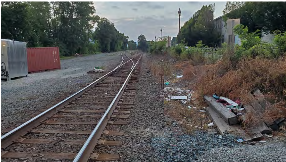
Figure 2-564. West Bank of the Hudson River Potential Transload Location Looking South
