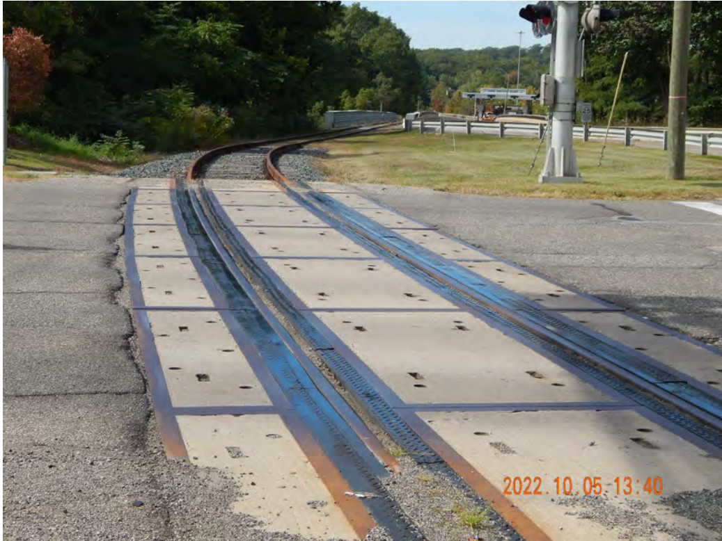
Figure 2-614. Grade Crossing on DC Cook Rail Spur Looking East
