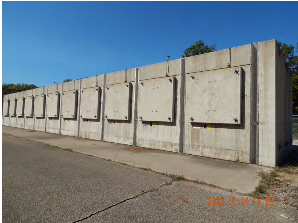
Figure 2-575. NUHOMS Dry Storage Systems at the East ISFSI at the Palisades Site
