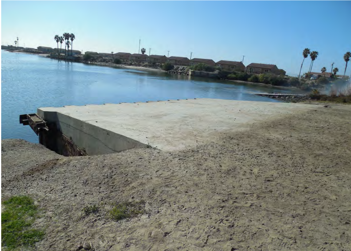
Figure 2-311. Del Mar Boat Basin Bulkhead (2016)
