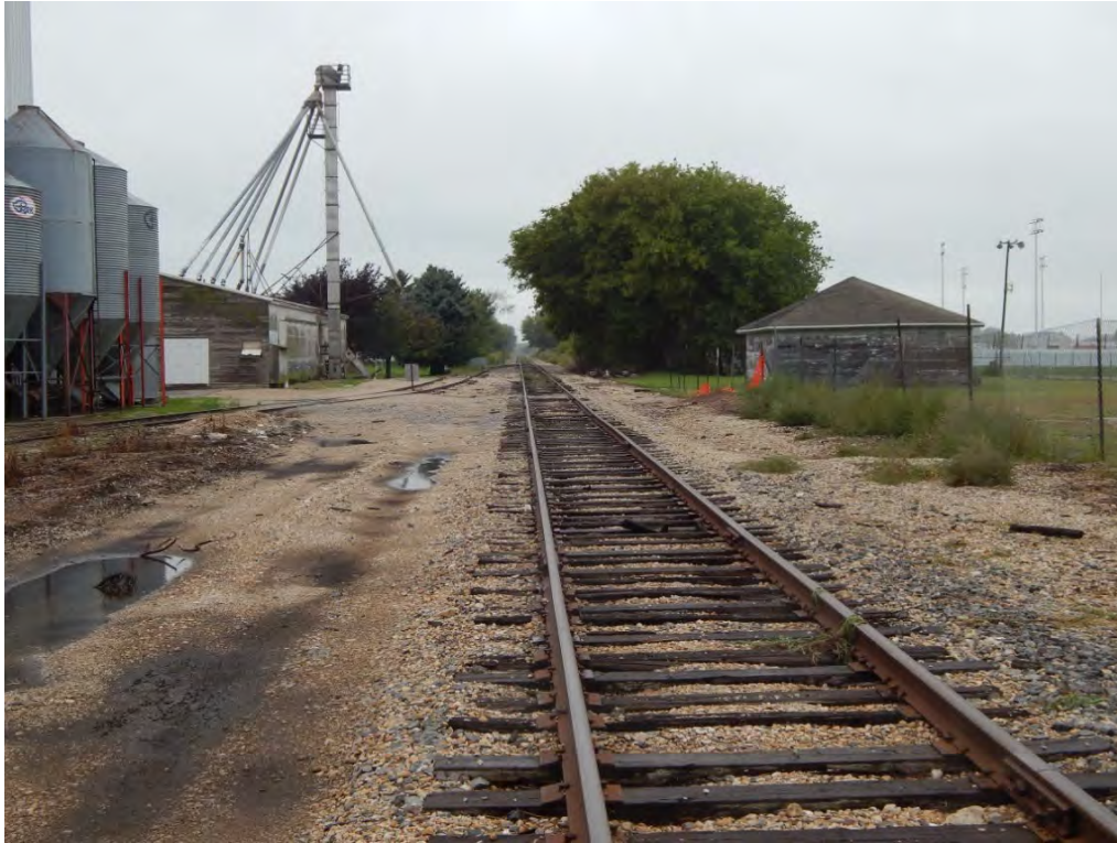
Figure 2-210. Potential Luxemburg Transload Location (Looking West) (2014)
