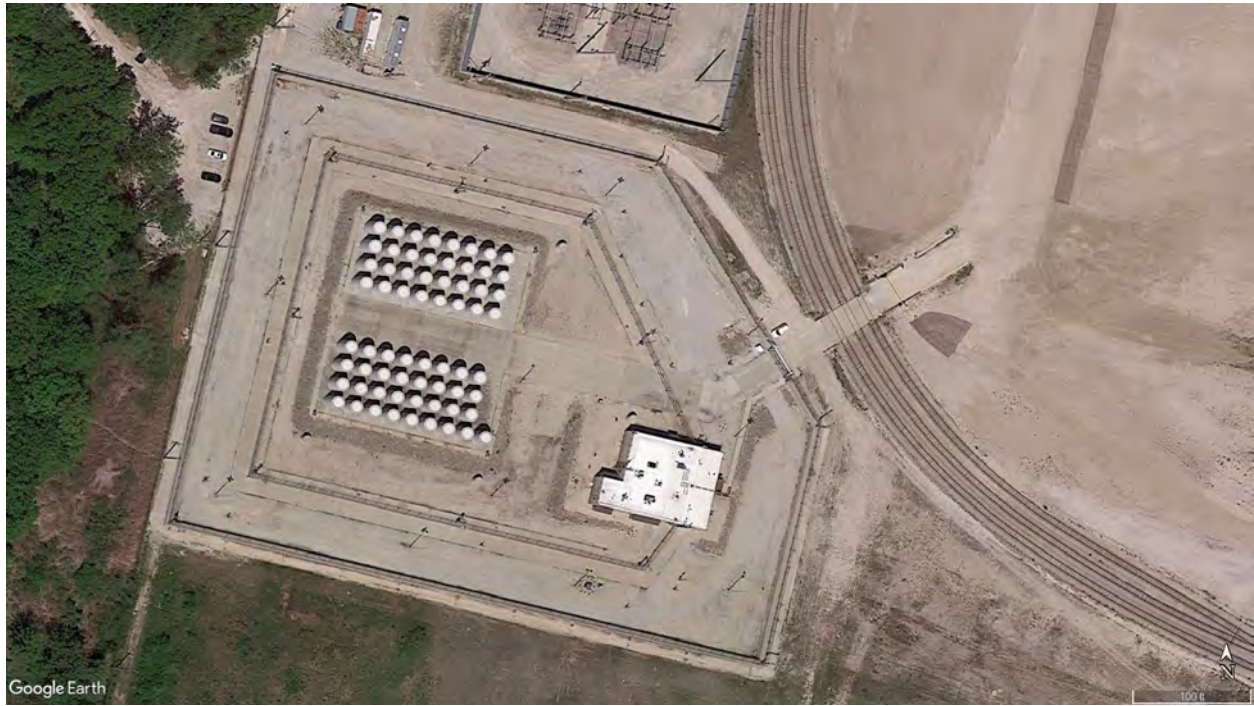
Figure 2-138. Aerial View of Zion Independent Spent Fuel Storage Installation (Google 2022)
