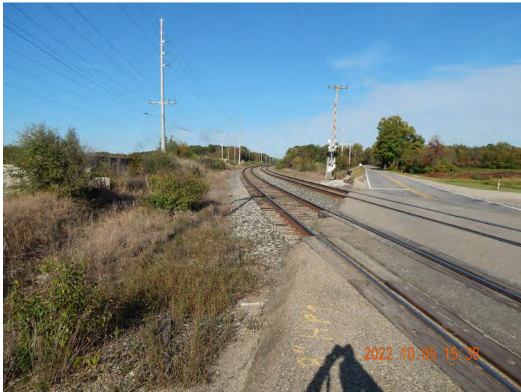
Figure 2-596. Quarry Potential Transload Location Looking North
