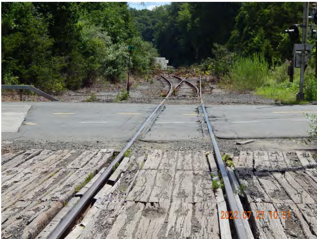
Figure 2-540. Segar Street Potential Transload Location Looking Southeast
