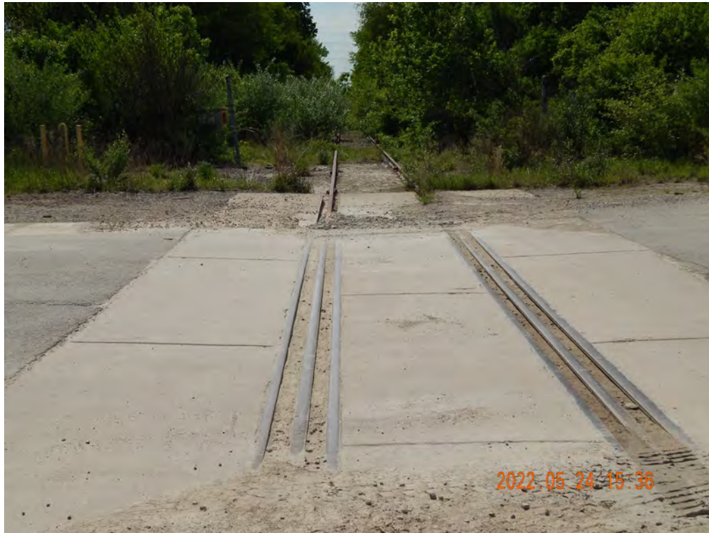
Figure 2-452. Grade Crossing at the Dresden Site Looking West
