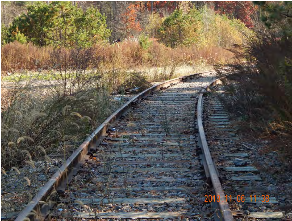
Figure 2-429. Industrial Spur at Second Potential Rail Transload Location Looking East (2019)
