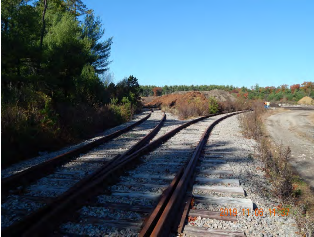
Figure 2-428. Industrial Spur at Second Potential Rail Transload Location Looking Northwest (2019)
