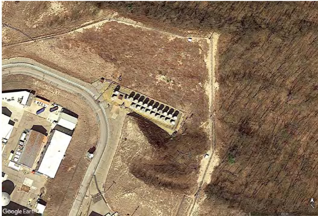
Figure 2-571. Aerial View of the Original ISFSI Containing VSC-24 Dry Storage Systems (Google 2022)
