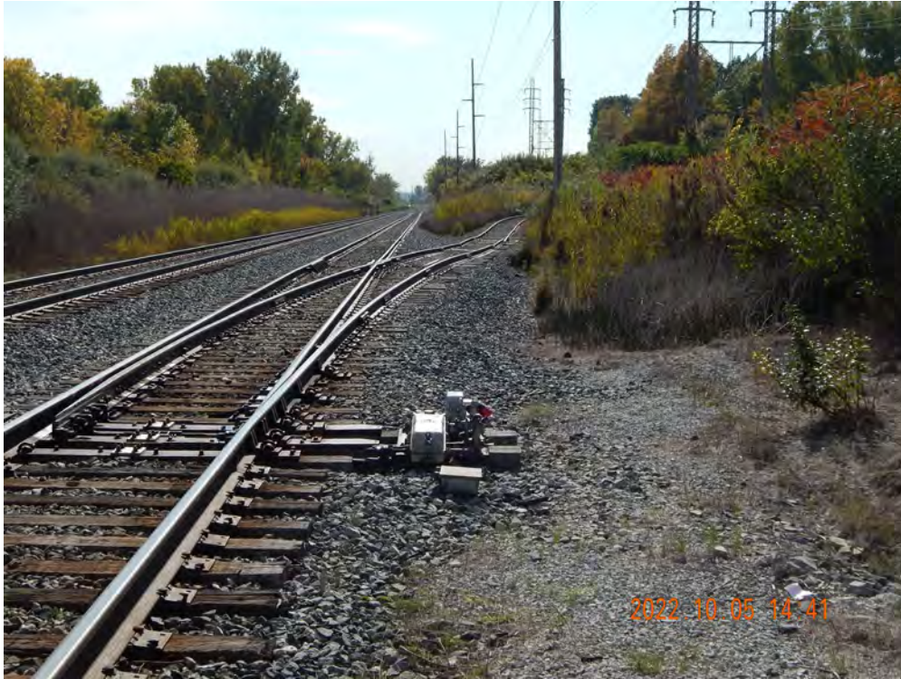
Figure 2-589. Rail Spur Near NoBo Marijuana Cultivation Facility Potential Transload Location Looking South
