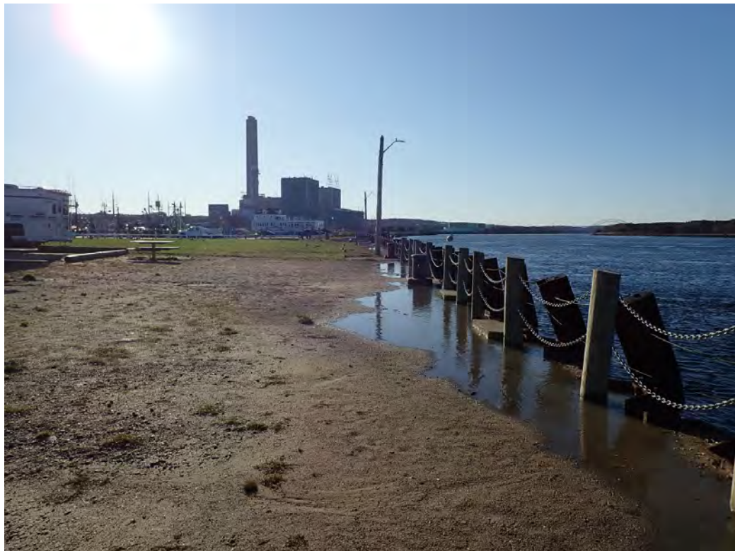
Figure 2-436. East Barge Transload Location Looking West (2019)
