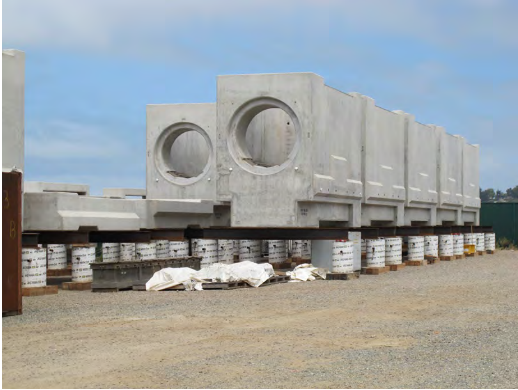
Figure 2-267. Horizontal Storage Modules (2015)
