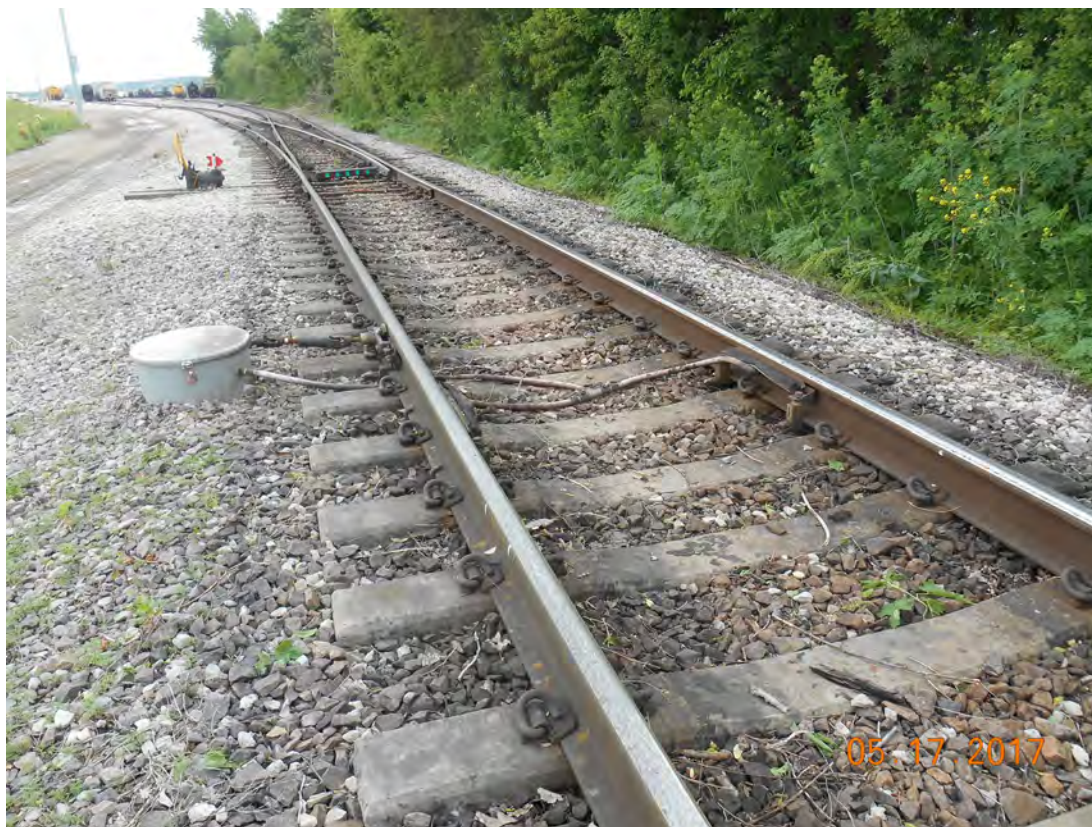
Figure 2-357. Derailer and Greaser on Cargill Industrial Spur (2017)
