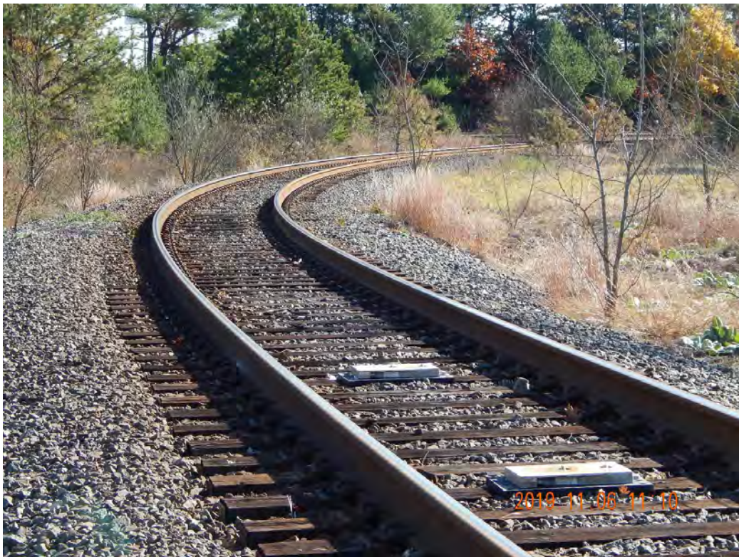
Figure 2-420. Positive Train Control Sensors at First Potential Rail Transload Location (2019)
