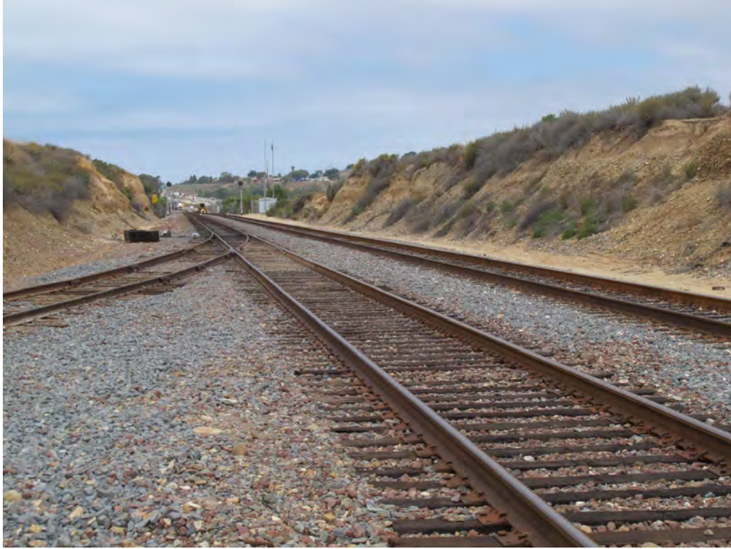
Figure 2-301. Mainline at San Onofre Site (Looking North) (2015)
