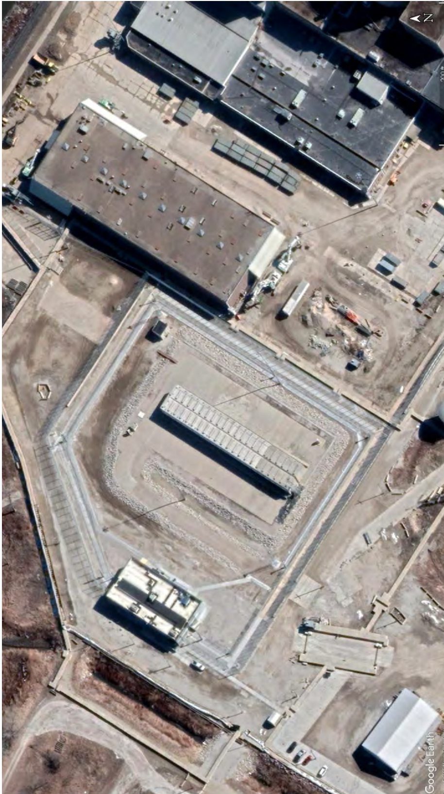
Figure 2-346. Aerial View of Fort Calhoun Independent Spent Fuel Storage Installation (Google 2022)
