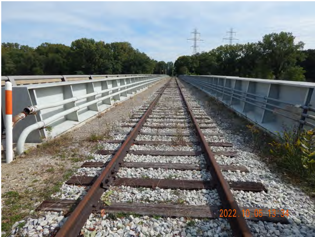
Figure 2-613. Rail Bridge on DC Cook Rail Spur Looking West
