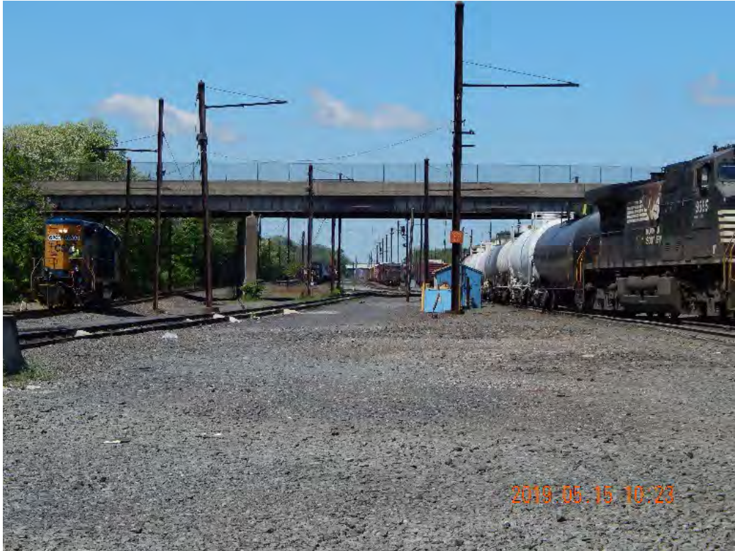
Figure 2-399. Morrisville Railyard Looking East (2019)
