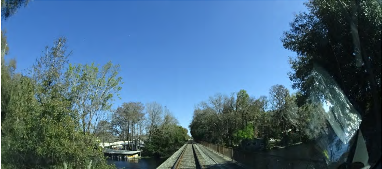
Figure 2-173. Florida Northern Railroad Bridge (2015)
