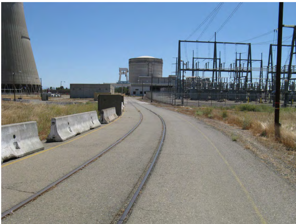
Figure 2-92. On-site Rail Spur Running into Rancho Seco Site (2013)
