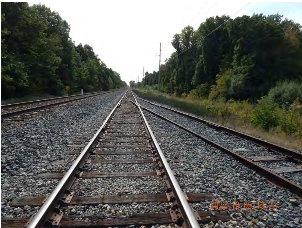
Figure 2-615. CSX Mainline at DC Cook Looking South
