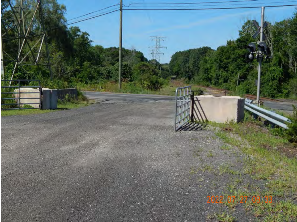
Figure 2-533. Hawleyville Road Entrance Looking Southwest
