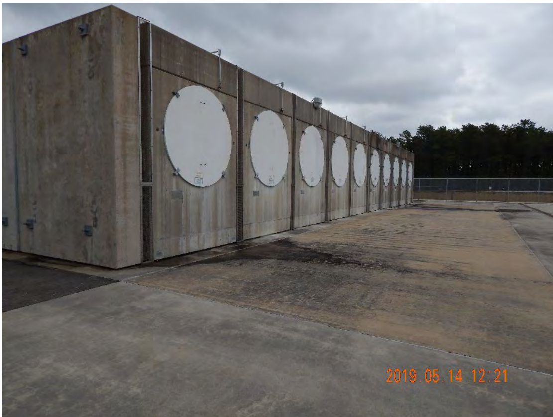
Figure 2-382. Ground-Level View of Oyster Creek Independent Spent Fuel Storage Installation (2019)
