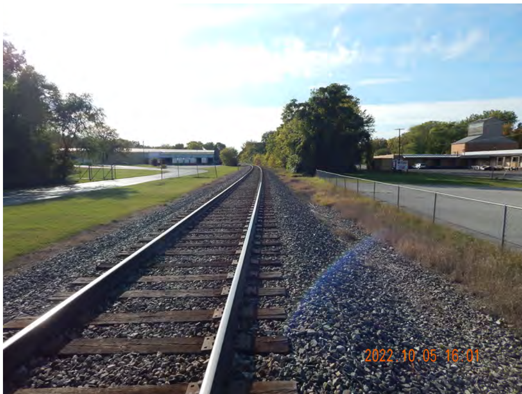
Figure 2-605. Menasha Packaging Potential Transload Location Looking West
