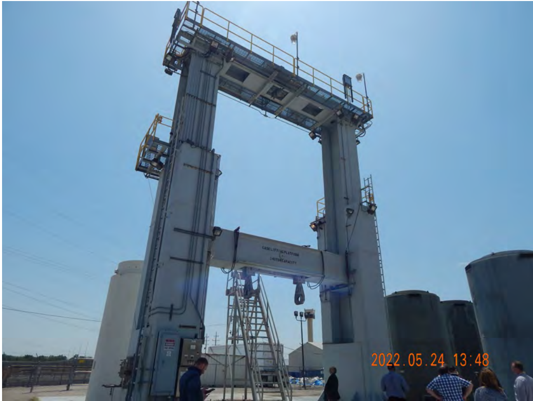
Figure 2-448. Cask Lifting Platform at Dresden Site
