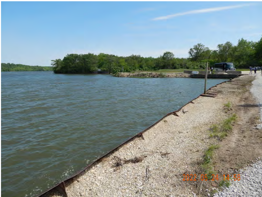
Figure 2-472. Dresden Barge Area Looking South
