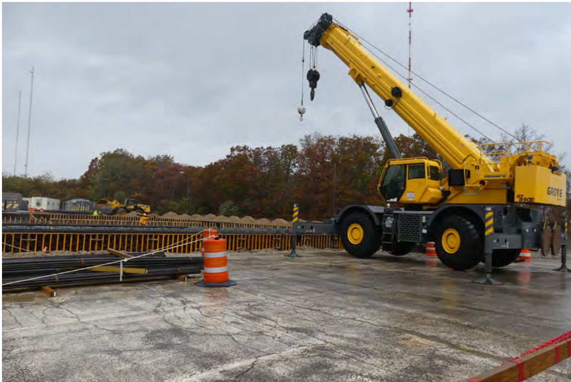
Figure 2-412. Construction of New Pilgrim Independent Spent Fuel Storage Installation (2019)
