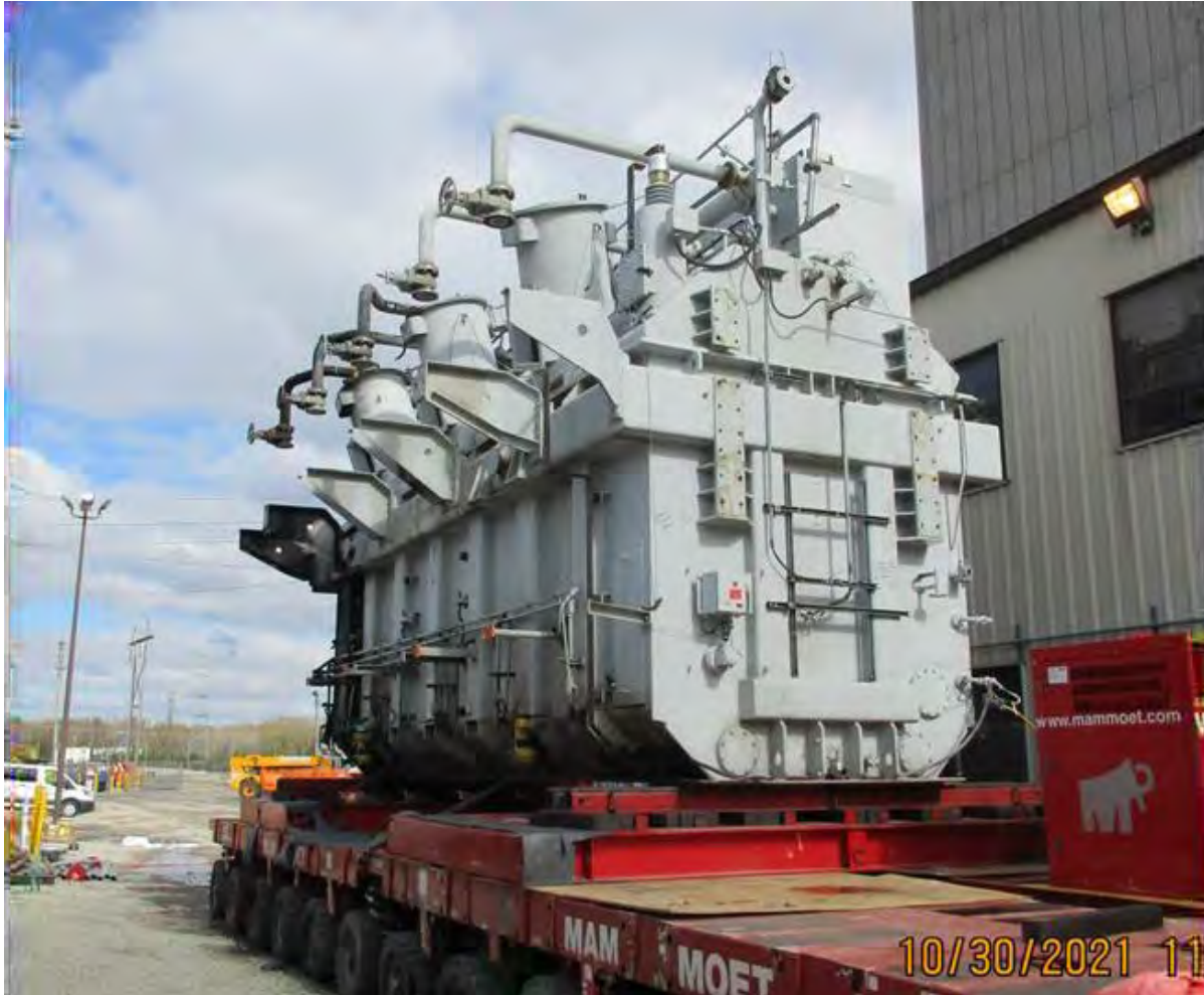
Figure 2-481. Transformer Being Shipped to Dresden Site
