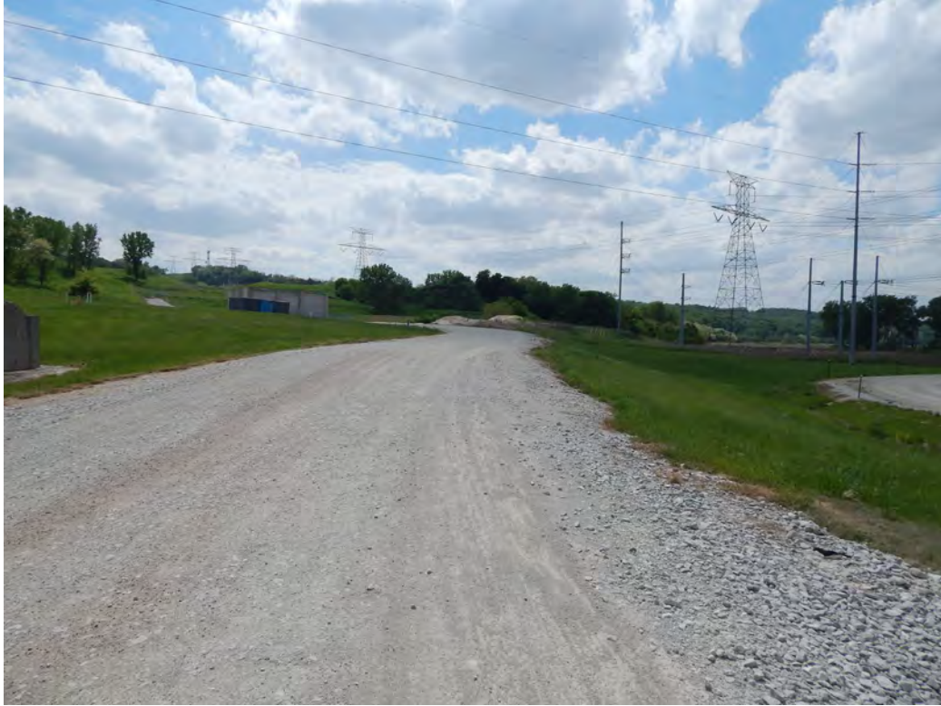
Figure 2-369. Current Condition of Haul Road (2017)
