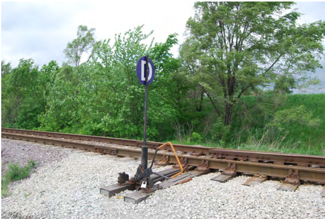
Figure 2-355. Derailer at Entrance to Cargill Industrial Spur (2017)
