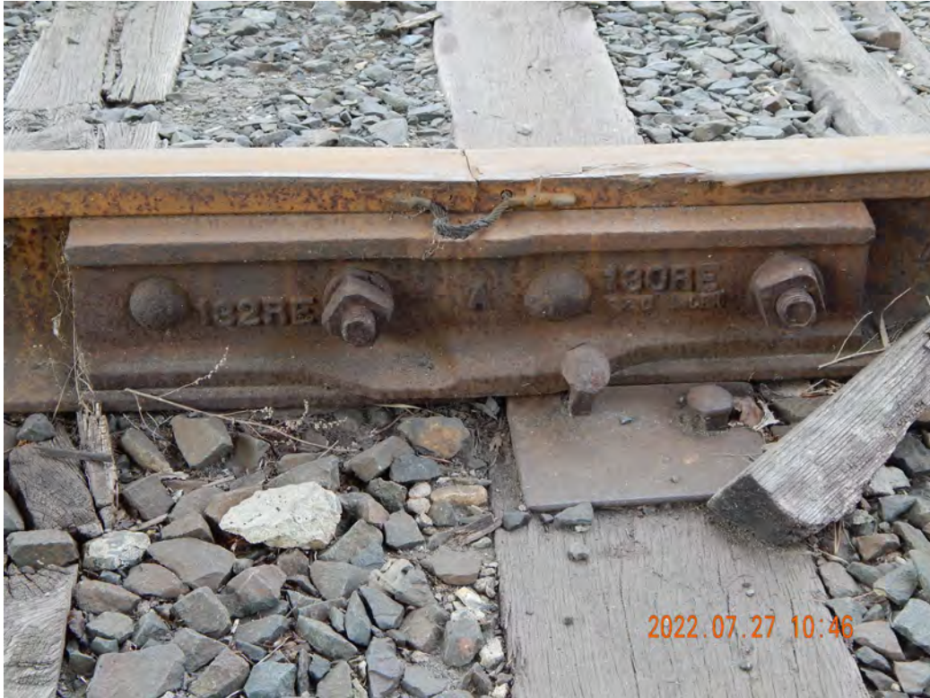
Figure 2-541. 132 lb. to 130 lb. Rail Joint at Segar Street Potential Transload Location
