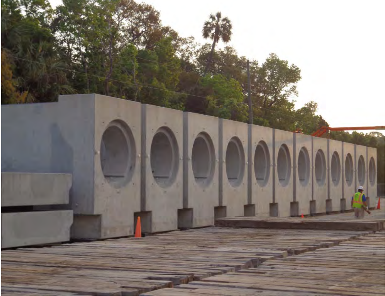
Figure 2-188. Horizontal Storage Modules at Nuclear Spur after Unloading (2015)
