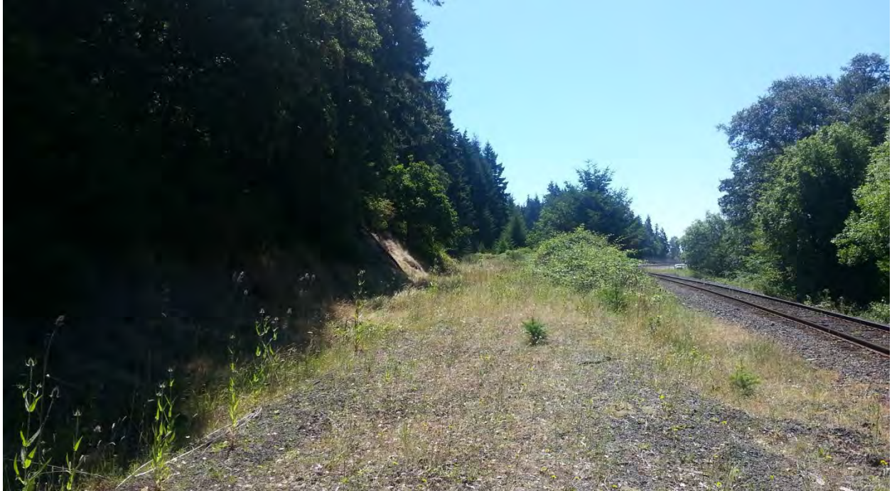
Figure 2-109. Former Trojan Rail Spur Railbed (2013)
