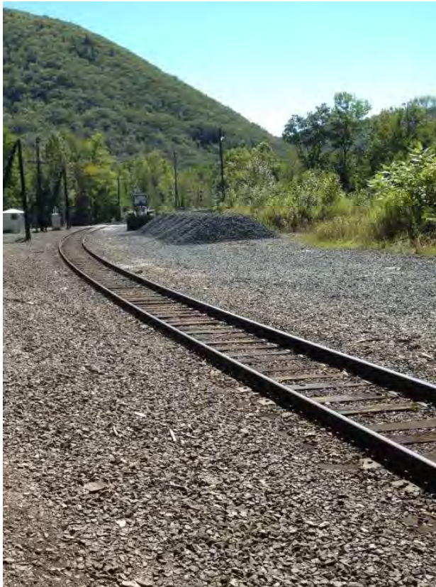
Figure 2-27. Rail Line at East Portal of the Hoosac Tunnel (2012)
