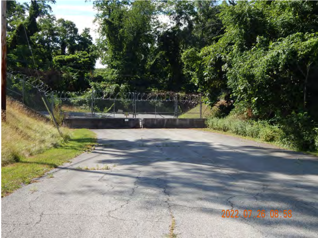
Figure 2-513. Indian Point South Entrance Looking East Towards Broadway
