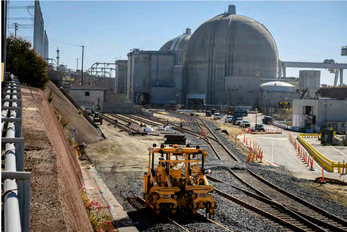
Figure 2-285. Expansion of On-site Rail Spur (Looking South) (2022)
