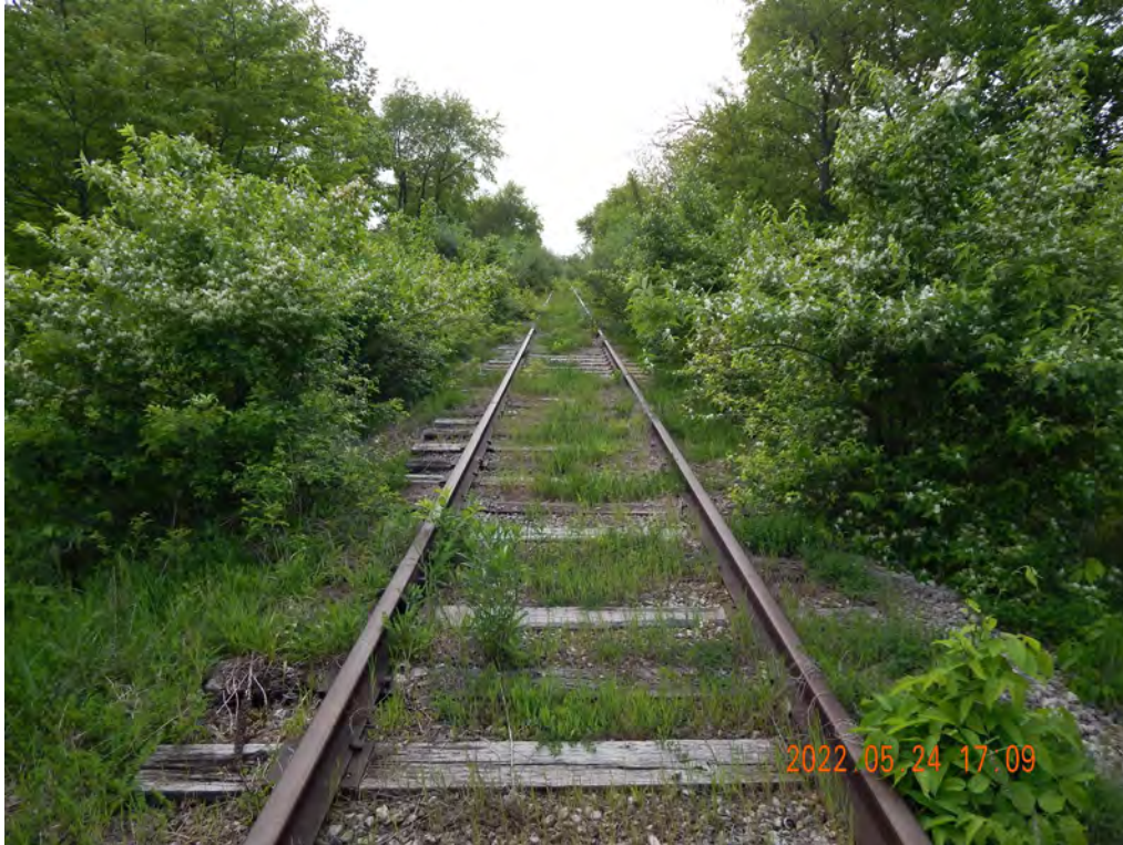
Figure 2-454. Rail Spur at Lock Road Looking West
