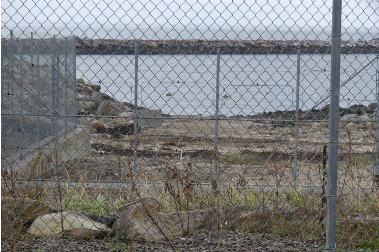
Figure 2-414. Barge Access at Pilgrim Site (2019)
