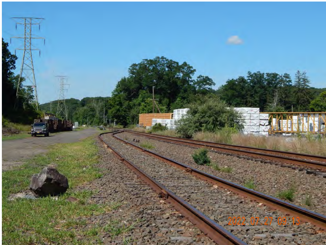
Figure 2-532. Hawleyville Road Potential Transload Location Looking Southwest
