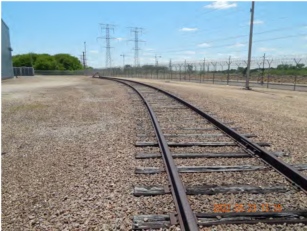
Figure 2-496. Western Rail Spur (Looking South)
