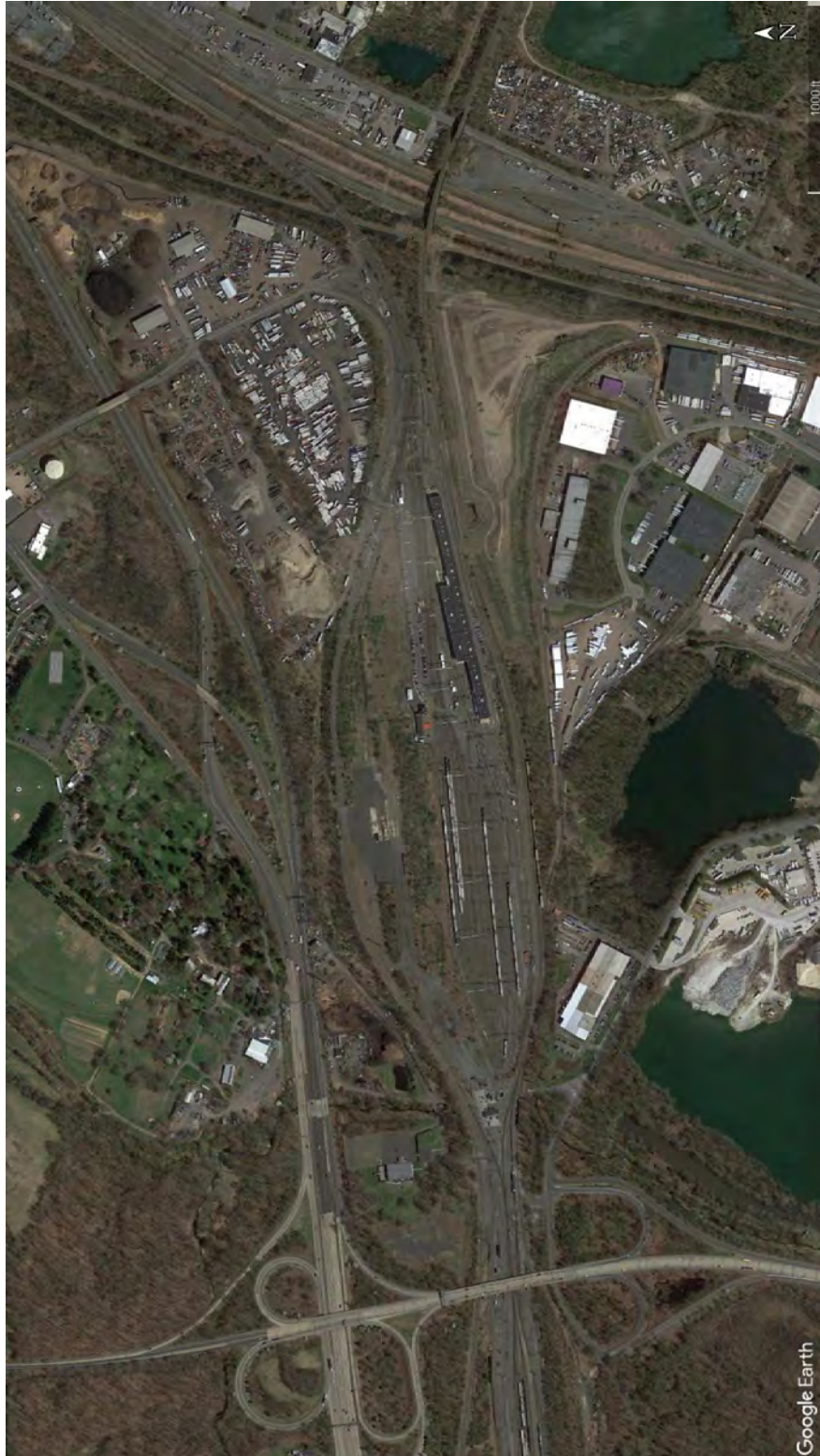
Figure 2-398. Aerial View of the Morrisville, Pennsylvania Railyard (Google 2022)
