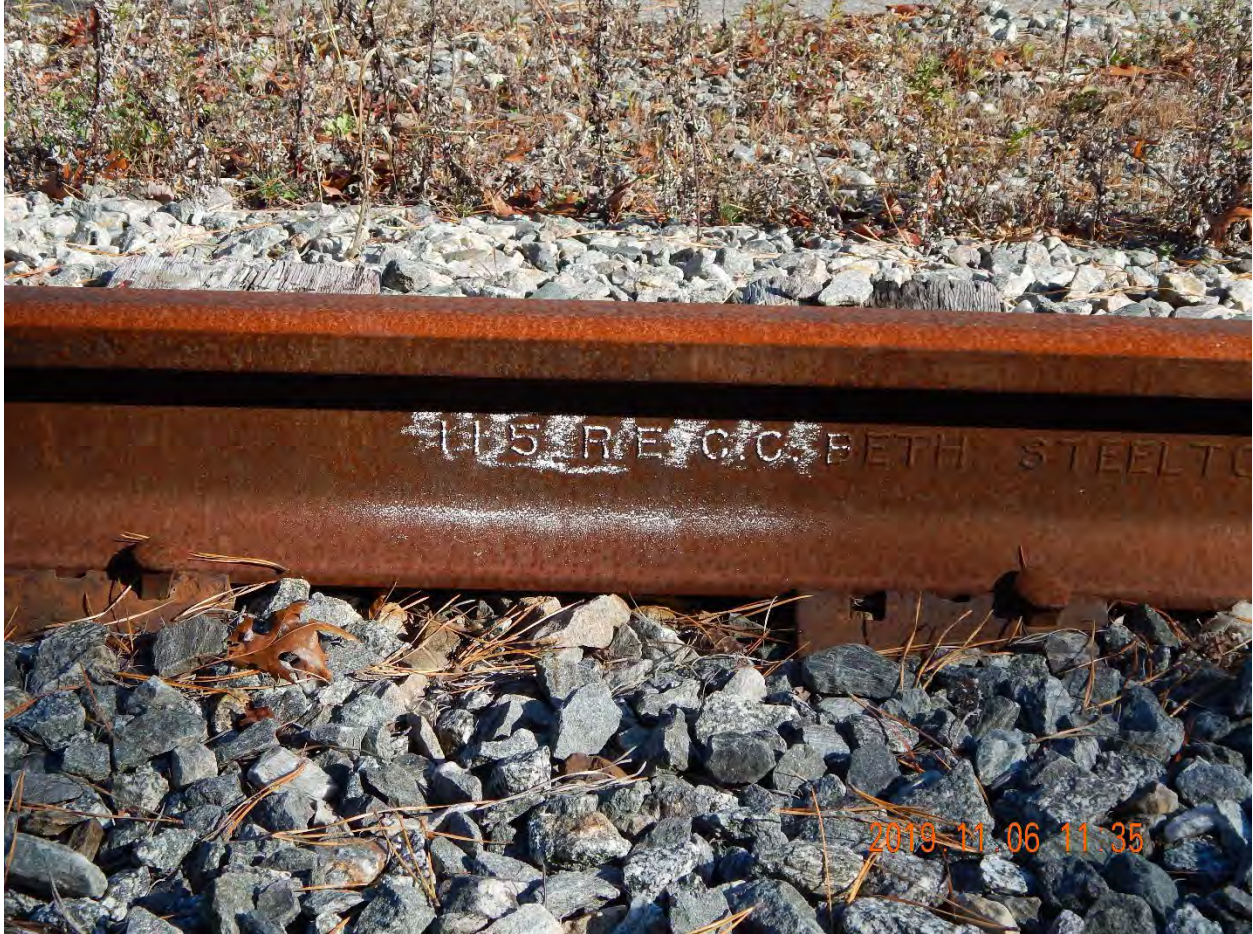
Figure 2-432. 115-lb. Rail at Industrial Spur at Second Potential Rail Transload Location (2019)
