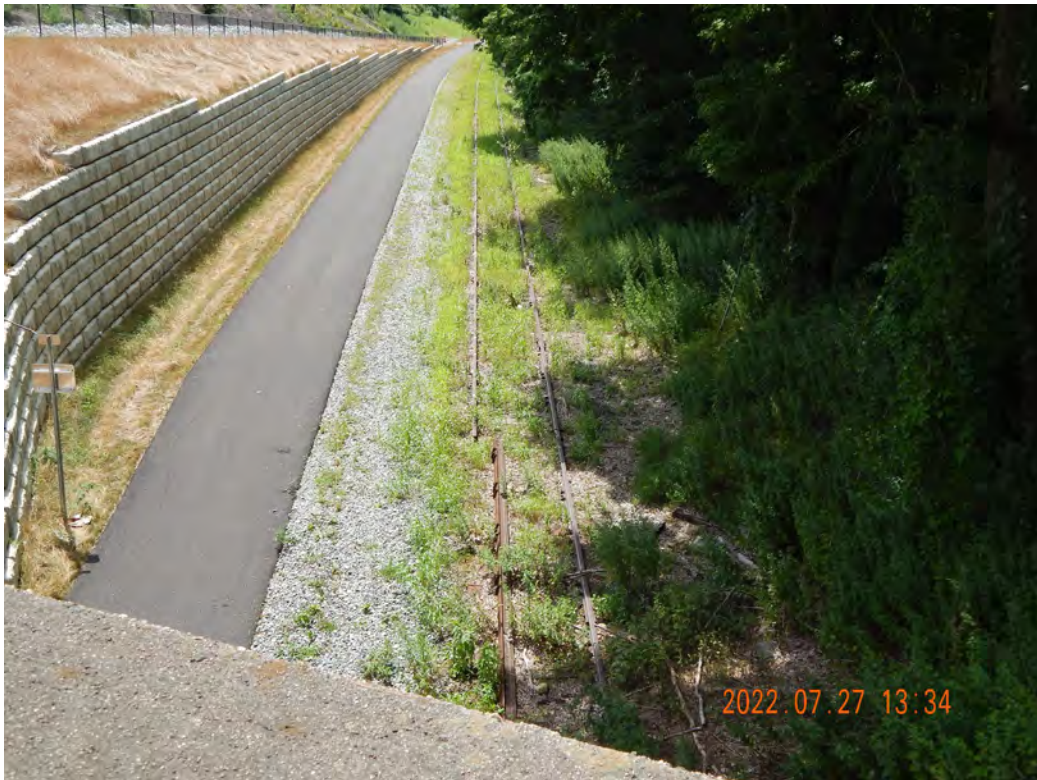
Figure 2-550. State Line Potential Transload Location Looking Southwest Towards New York
