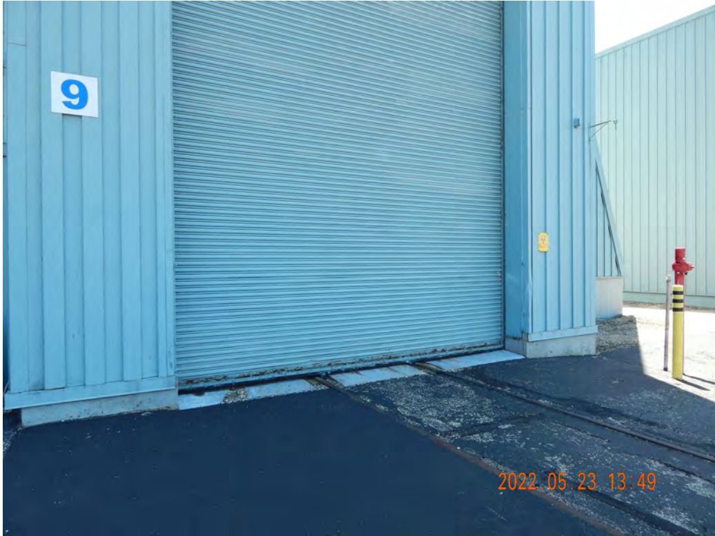
Figure 2-495. Railroad Tracks into the Cask Service Facility
