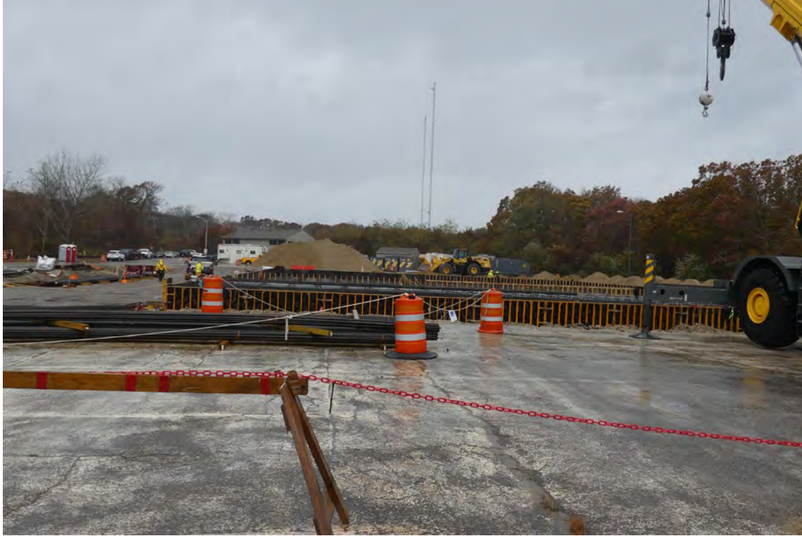
Figure 2-411. Construction of New Pilgrim Independent Spent Fuel Storage Installation (2019)
