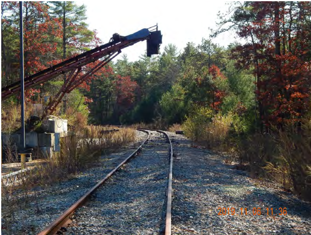
Figure 2-427. Industrial Spur at Second Potential Rail Transload Location Looking South (2019)
