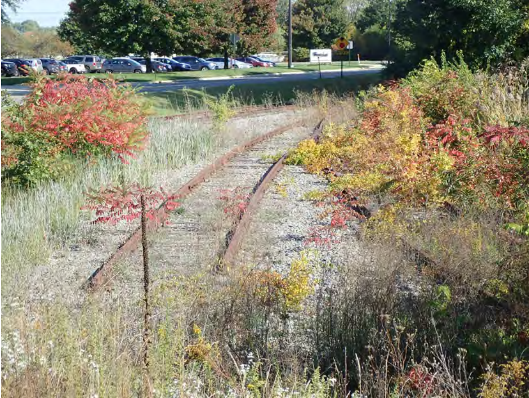
Figure 2-594. Aludyne Potential Transload Location Looking North Showing Spur
