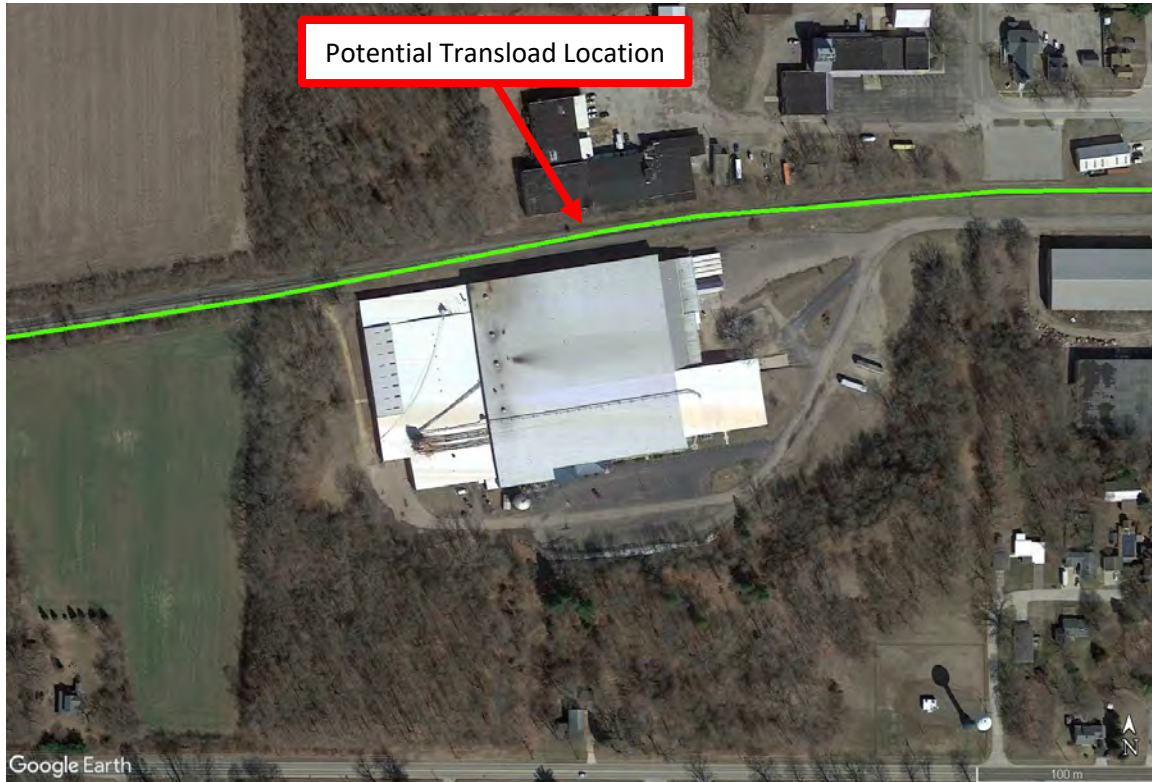
Figure 2-604. Aerial View of Menasha Packaging Potential Transload Location (Google 2022)
