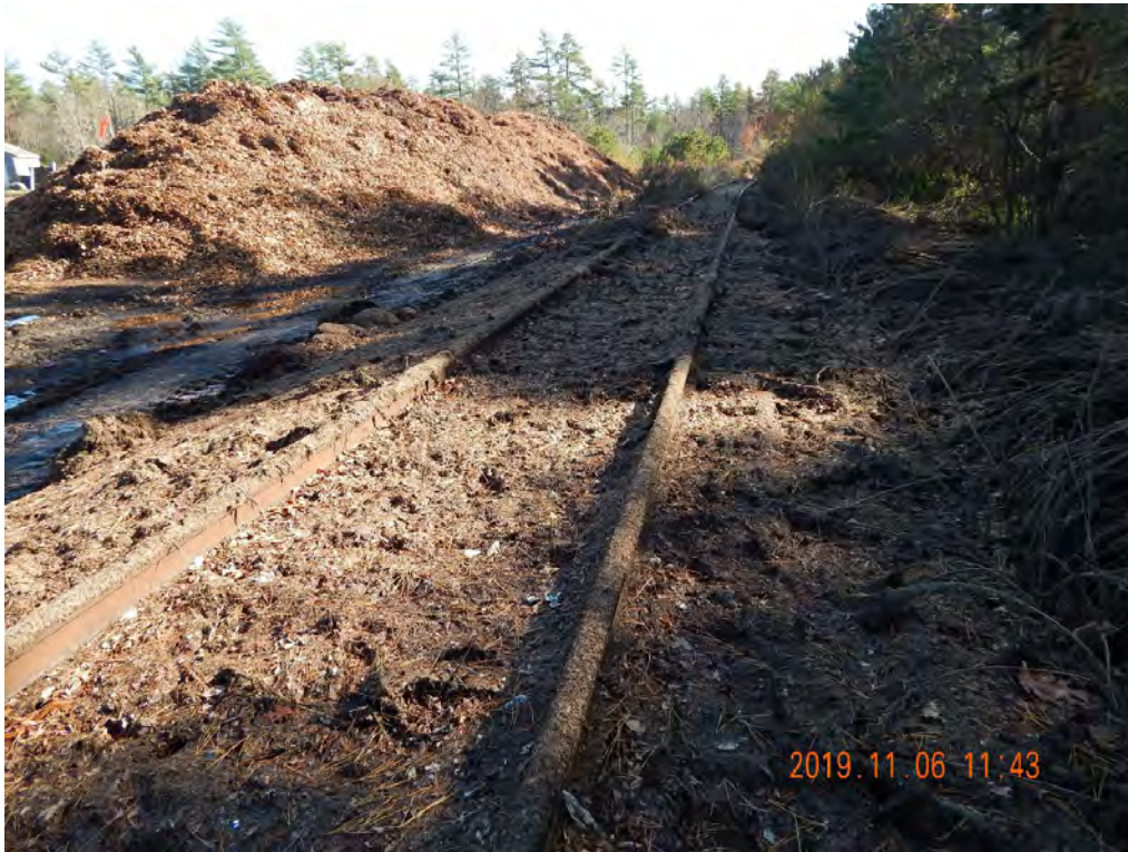
Figure 2-430. Industrial Spur at Second Potential Rail Transload Location Covered with Mulch (2019)
