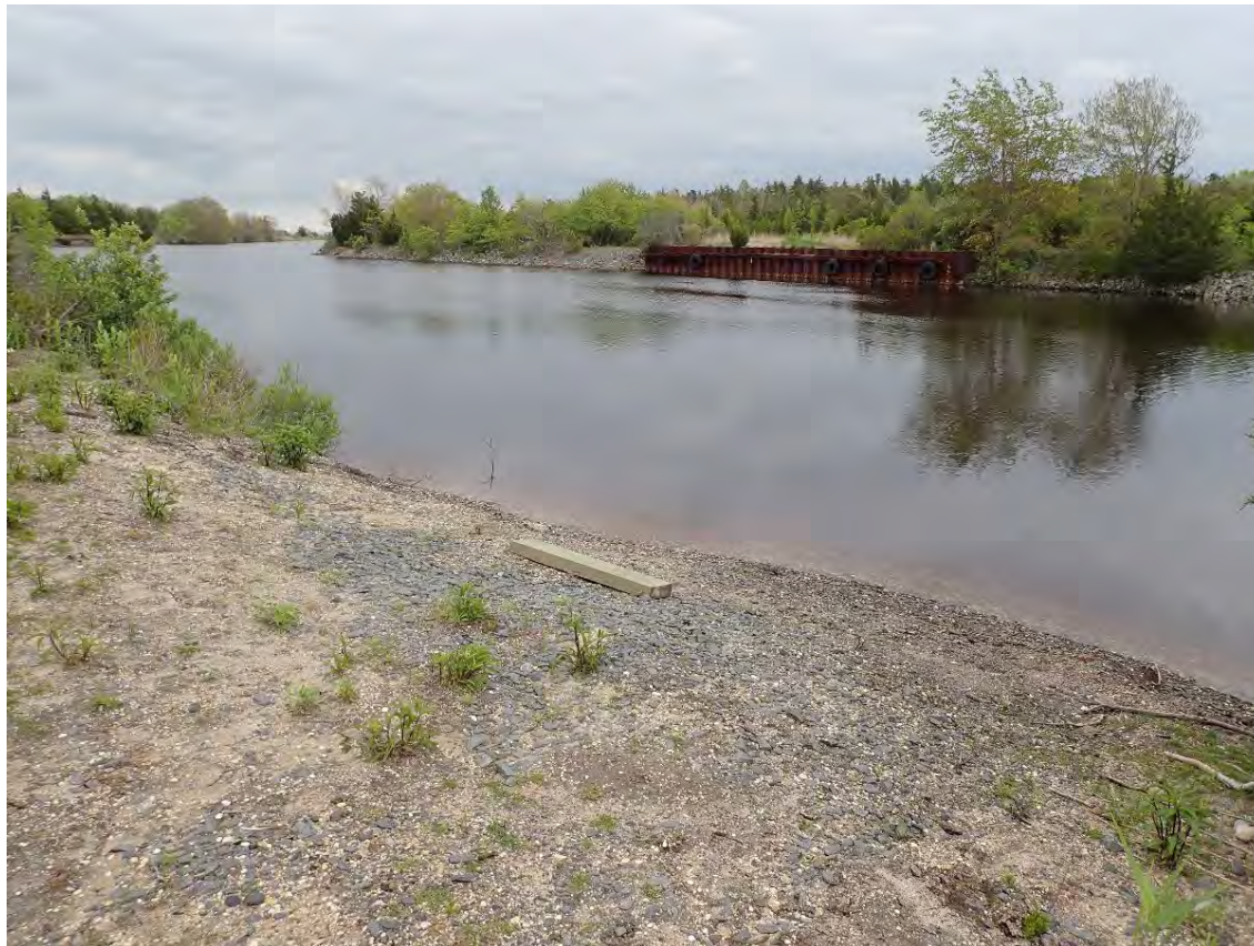
Figure 2-384. Oyster Creek Barge Access (North Bank of Oyster Creek) (2019)
