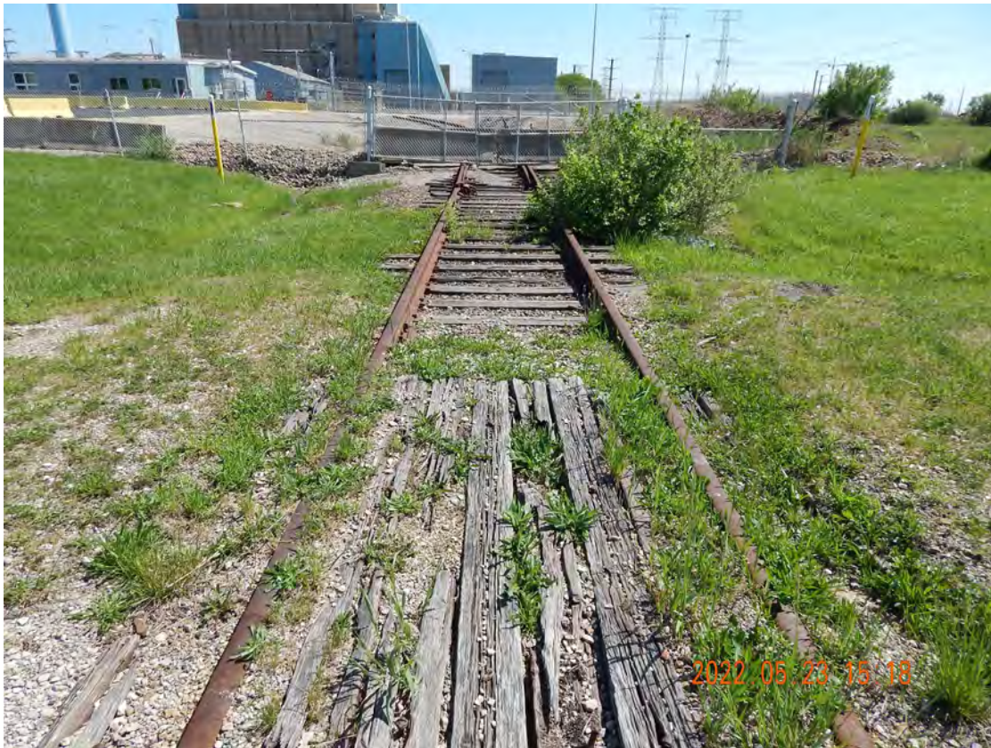
Figure 2-500. Morris Rail Spur Approaching the Morris Site
