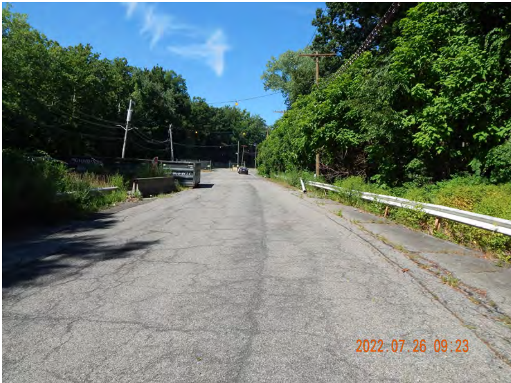
Figure 2-516. Indian Point North Entrance Looking West Towards Hudson River
