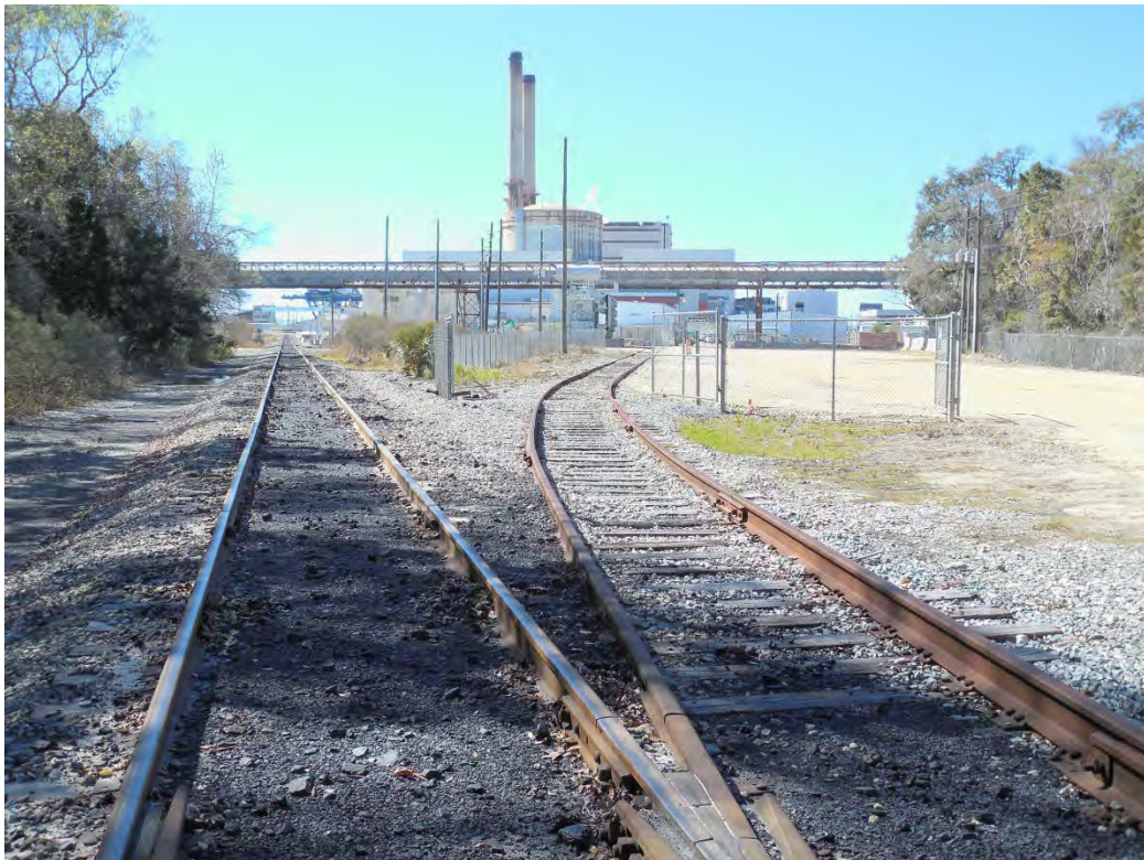
Figure 2-159. Junction of On-site Industrial Spur (Left) and Nuclear Spur (Right) (2015)
