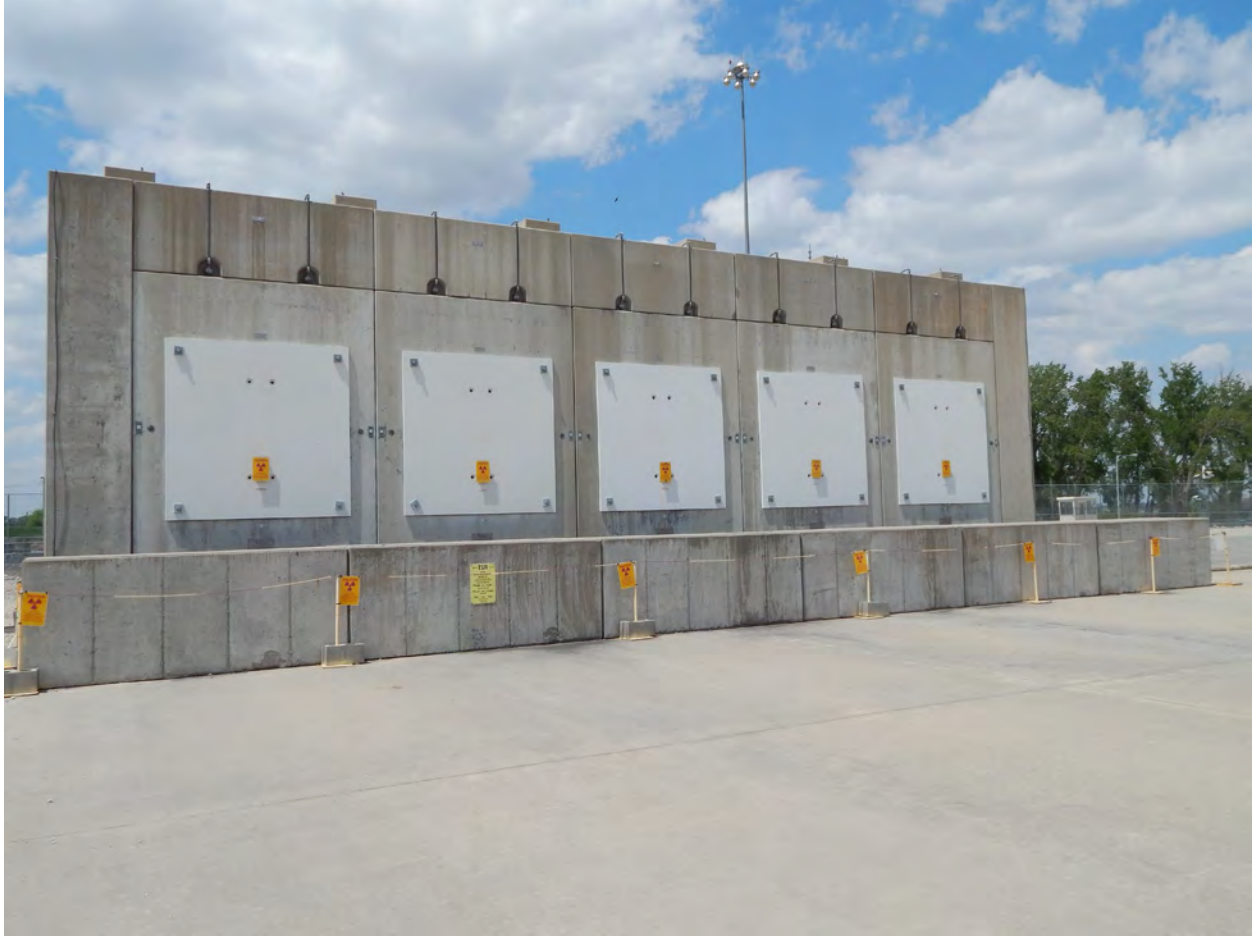
Figure 2-345. Fort Calhoun Independent Spent Fuel Storage Installation (2017)
