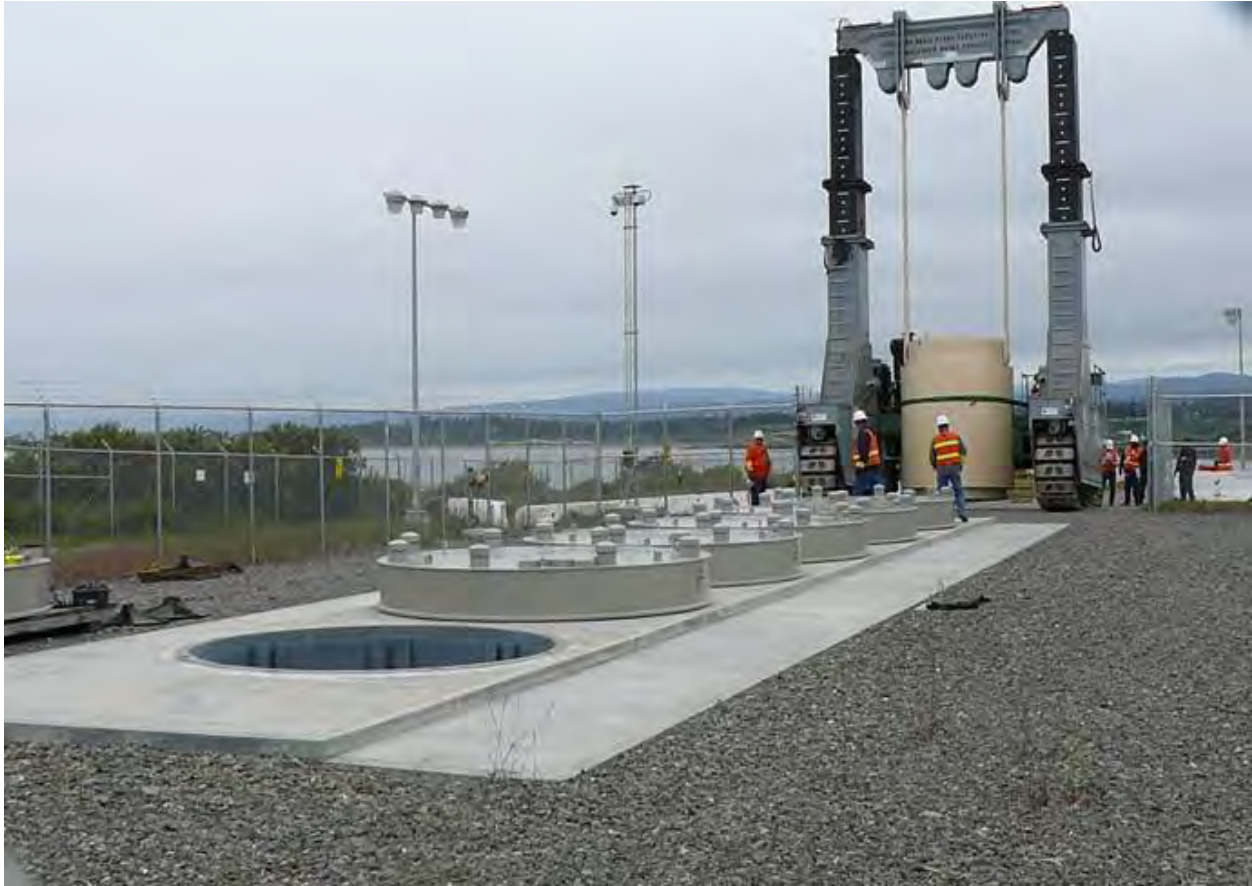
Photo courtesy of Humboldt Bay
