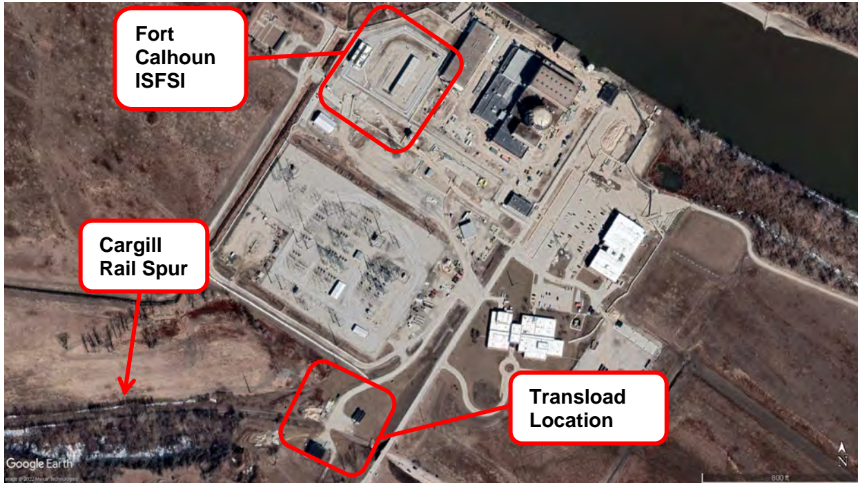
Figure 2-363. Aerial View of Transload Location (Google 2022)
