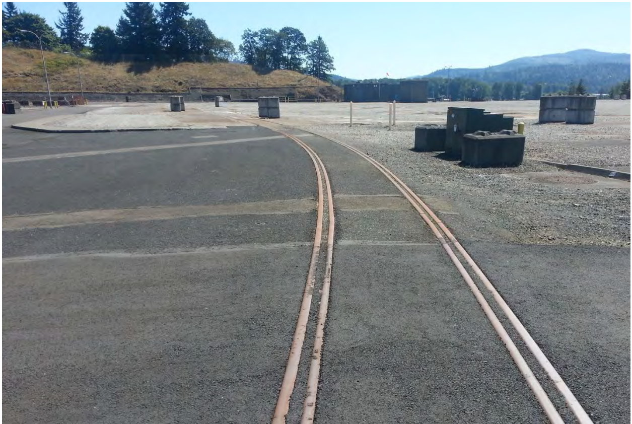
Figure 2-110. Remnants of On-site Rail Spur at Trojan (2013)
