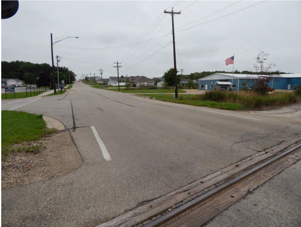
Figure 2-227. Potential Denmark Transload Location (Looking West) (2014)
