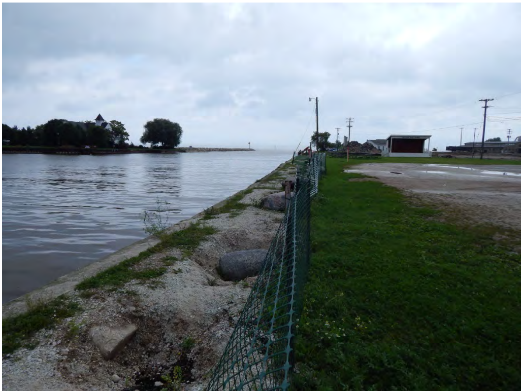
Figure 2-249. Potential Kewaunee Barge Transload Location Water Front (2014)
