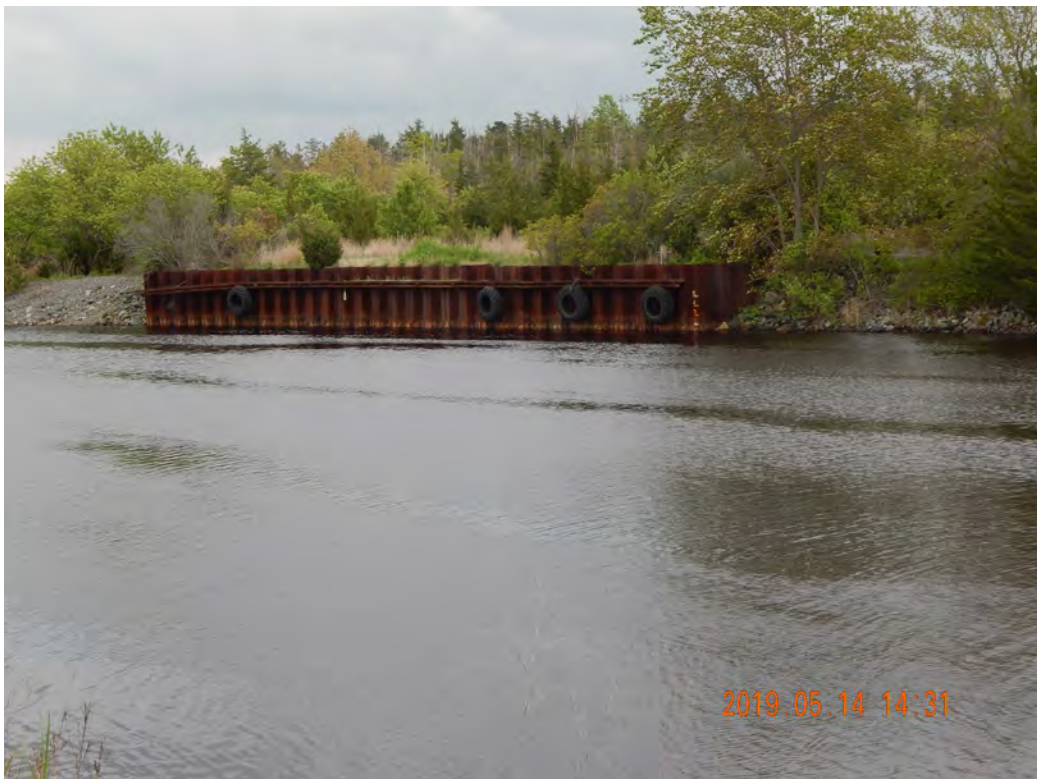
Figure 2-386. Oyster Creek Barge Access Road (South Bank of Oyster Creek) (2019)
