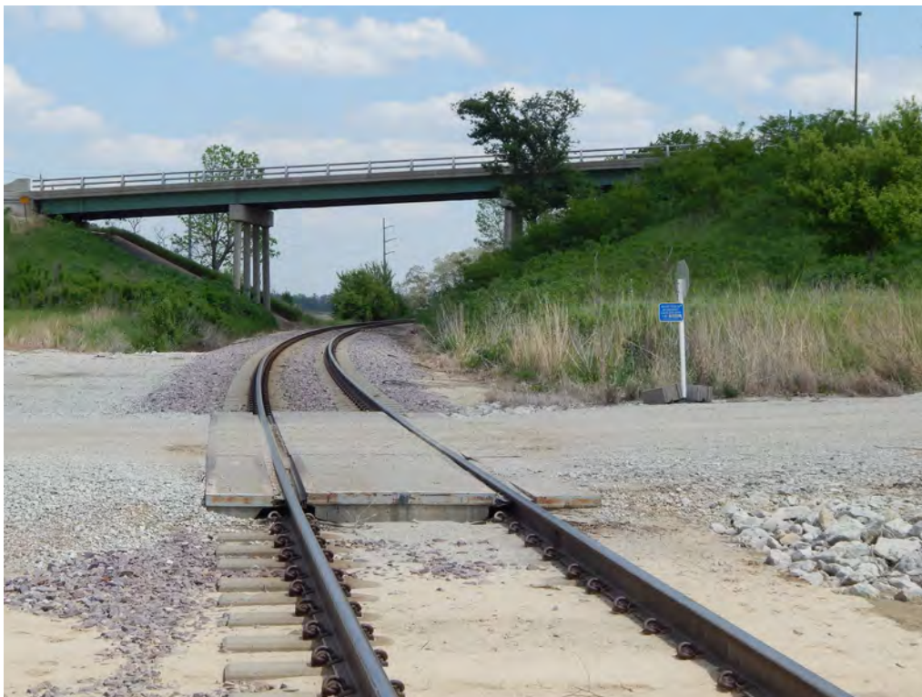
Figure 2-349. Cargill Industrial Spur (Looking Southeast) (2017)
