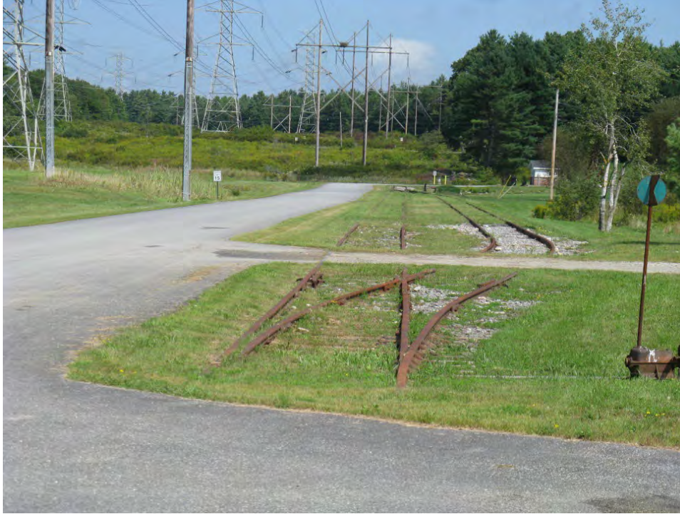
Figure 2-13. Paved-over Railroad Tracks at the Maine Yankee Site (2012)
