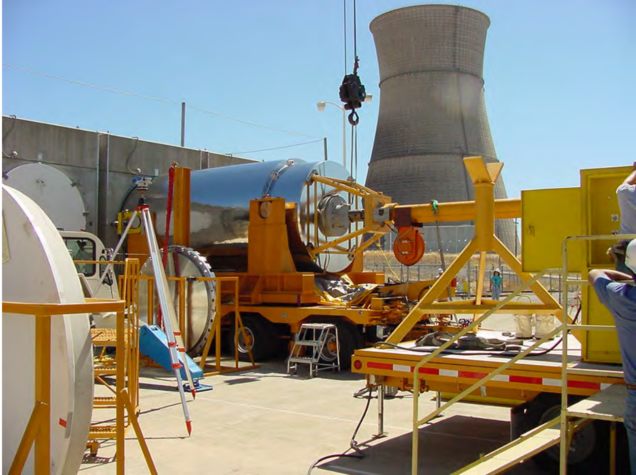
Figure 2-87. MP187 Transportation Cask and Hydraulic Ram Being Used to Load a Canister into a Horizontal Storage Module at Rancho Seco
