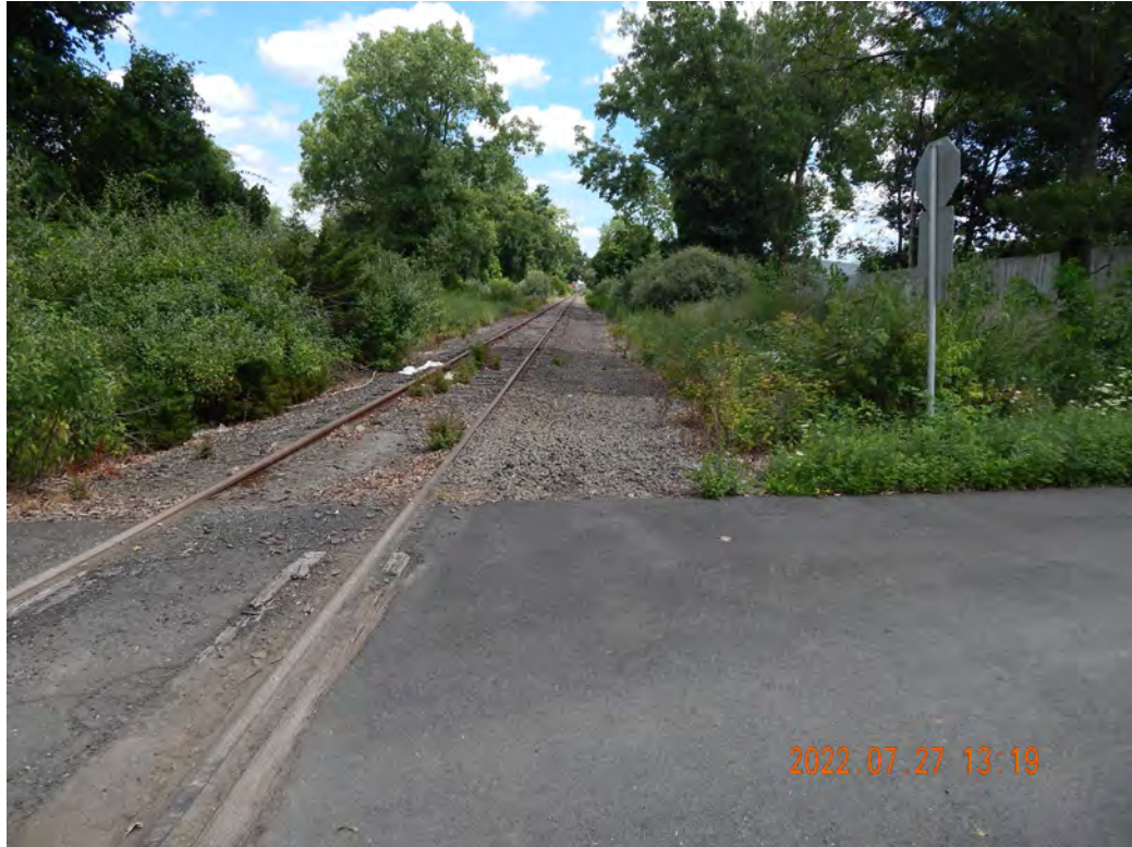
Figure 2-545. Agriventures Agway Potential Transload Location Looking Southeast
