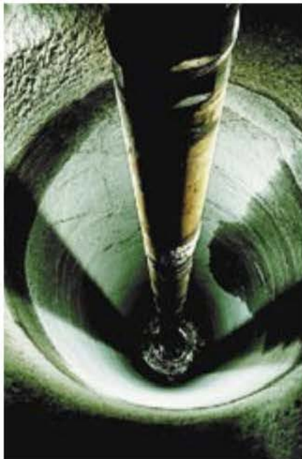
Drilling of a canister hole.
