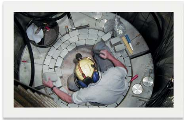
Installation of bentonite in a test deposition hole.
