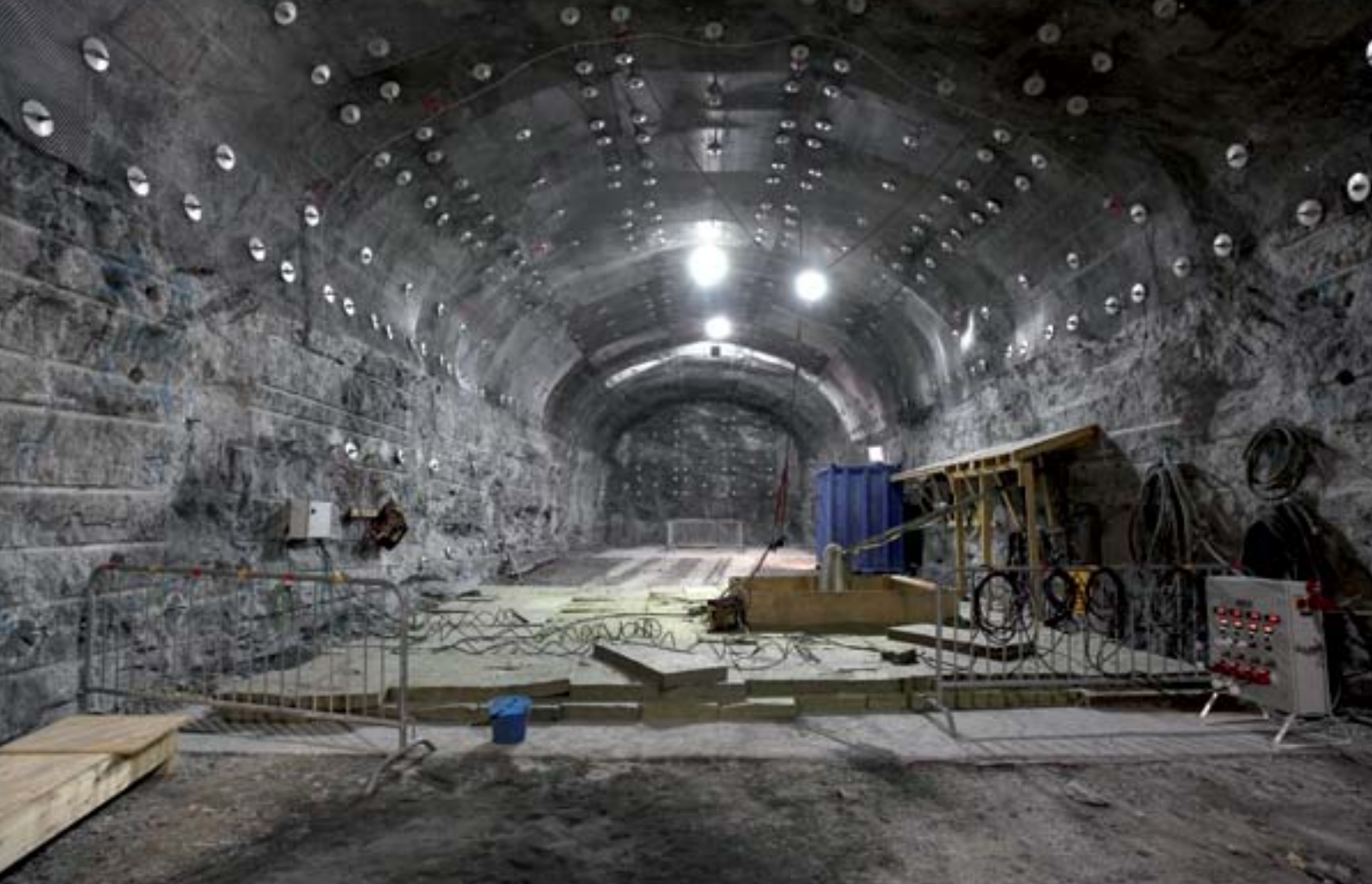
ONKALO's research facility 3 ("Pose" niche) studies the effect of heat on rock spalling in the test holes drilled in the floor of the facility.
