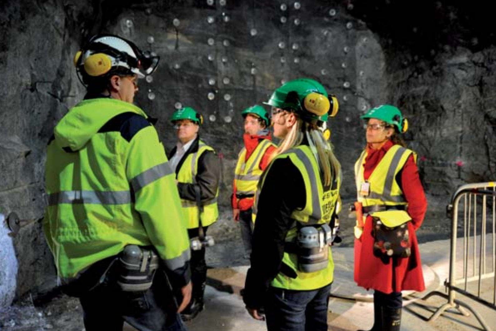
Janne Laihonen presents tunnel reinforcements in ONKALO's research facility 3 ("Pose" niche).
