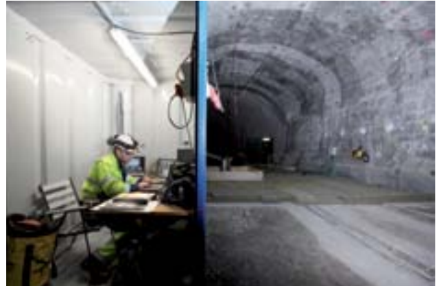
Collection of measurement data in ONKALO's research facility 3.
