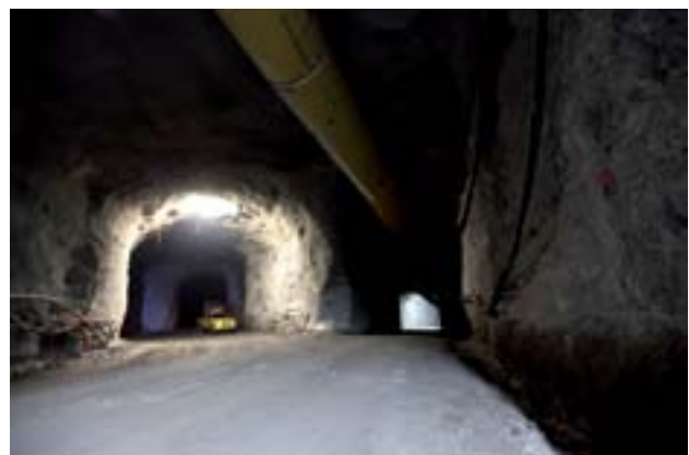
View of ONKALO at final disposal depth.
