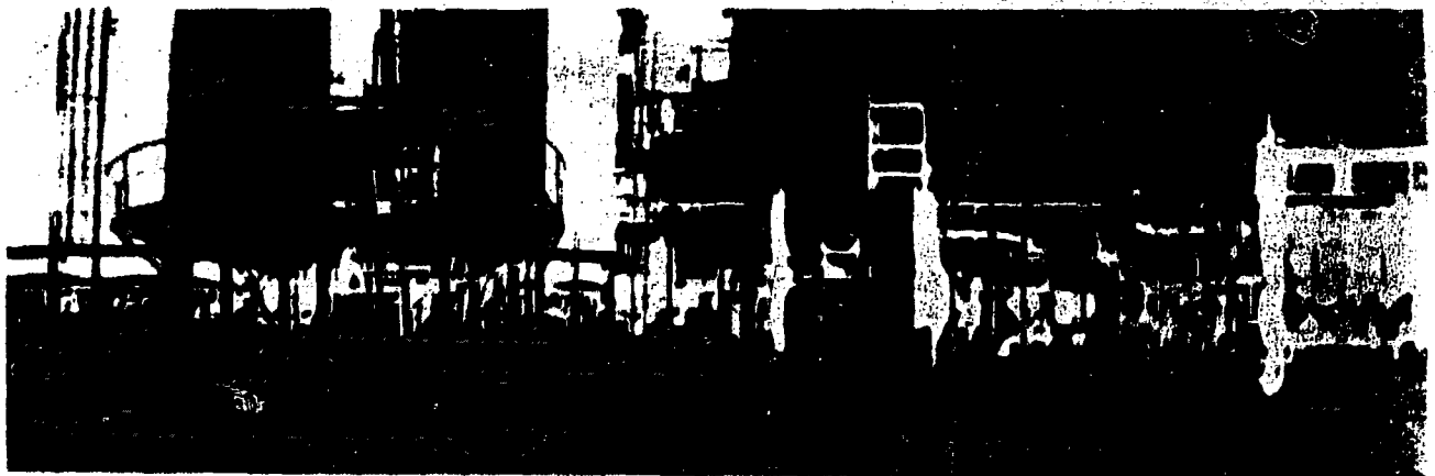
Heat paints a portrait of an energy-leaking chemical plant in this "thermograph" made by an infrared scanner, increasingly used these days to spot such
