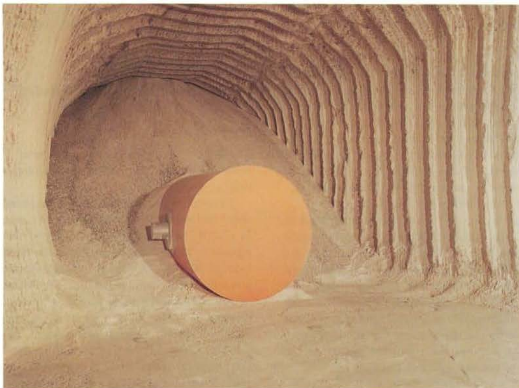
Figure 6-3. Demonstration of horizontal emplacement of a German Custos canister in a salt formation.
