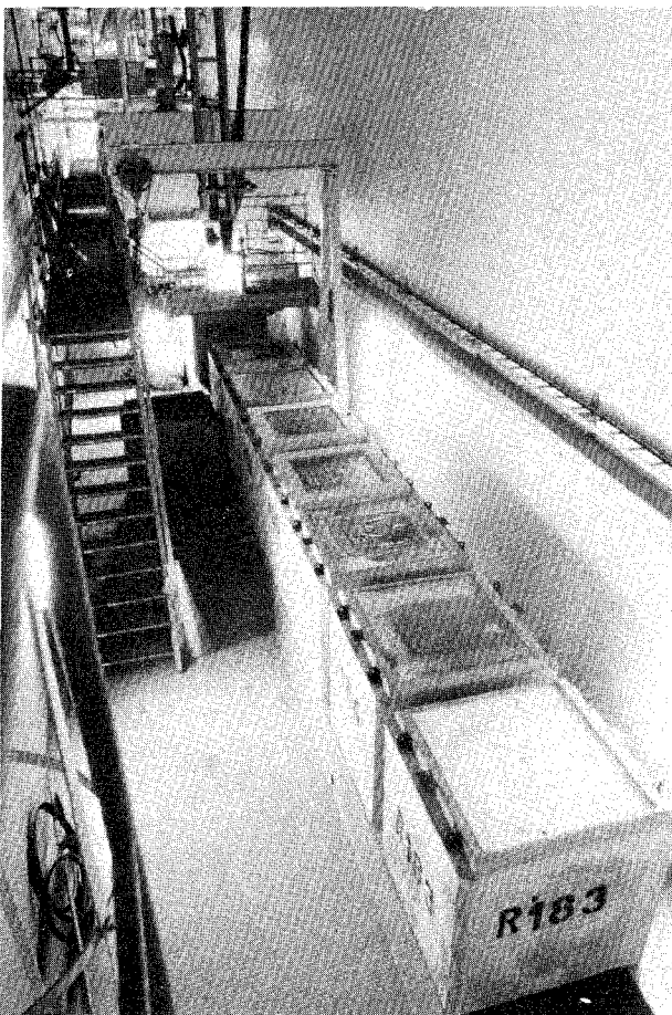
Figure 2-3. Solidification of ion exchange resin in concrete moulds at Ringhals nuclear power station.
