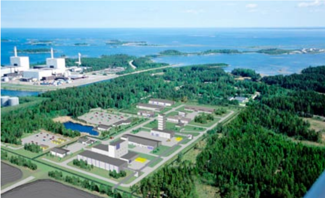
Figure 4-4. Photomontage showing the final repository's surface facilities located on the southern part of the industrial area in Forsmark (Layout D1).
