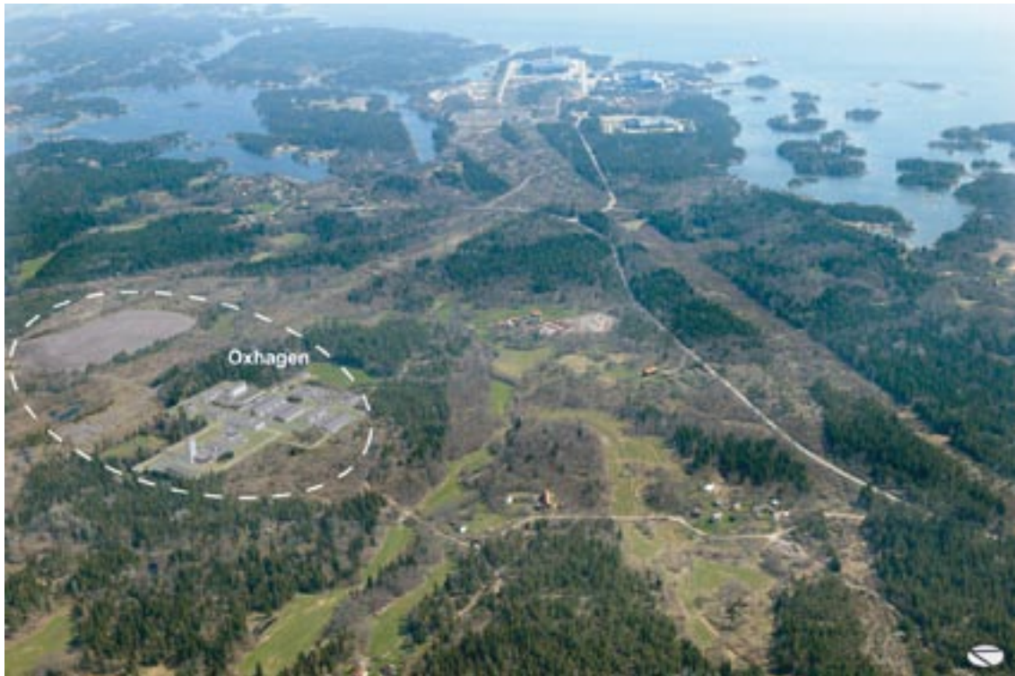
Figure 4-8. View over parts of the Laxemar area with a photomontage of envisioned surface facilities and rock heaps for the final repository at Oxhagen and the Simpevarp Peninsula in the background.
