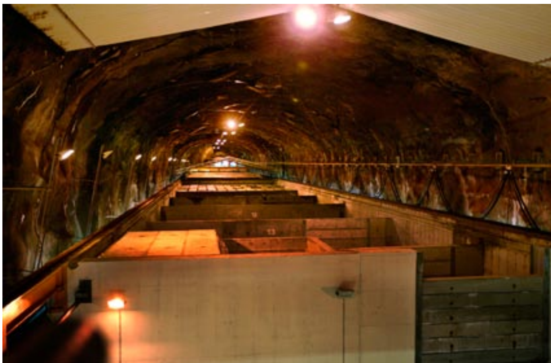
Figure 1-2. Interior from the final repository for low- and intermediate-level operational waste.
