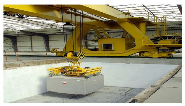
Fig. Disposal of VBK to disposal boxes of the repository in the first double row
