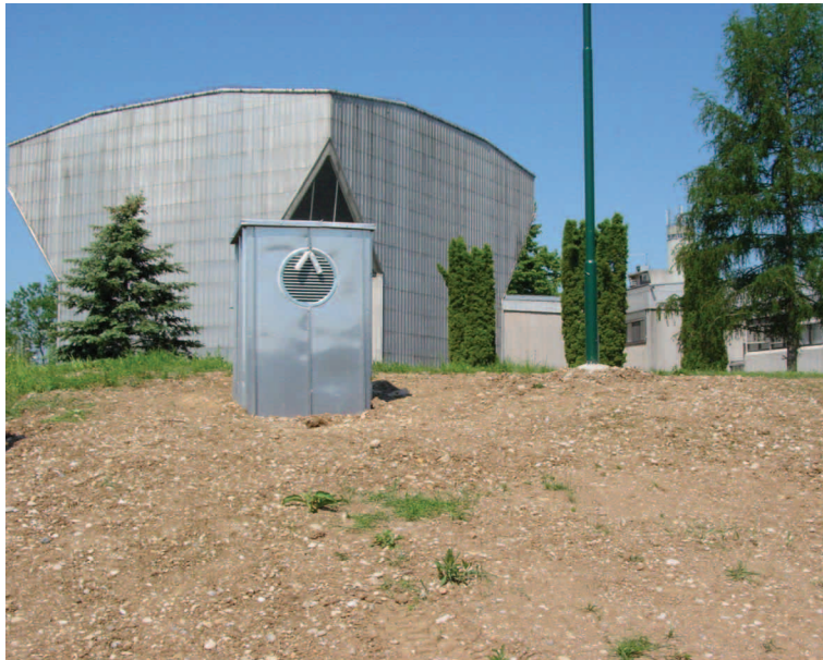
Figure 11: View of the IJS Reactor Infrastructure Centre
