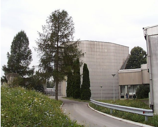
Figure 13: View of the IJS Reactor Infrastructure Centre
