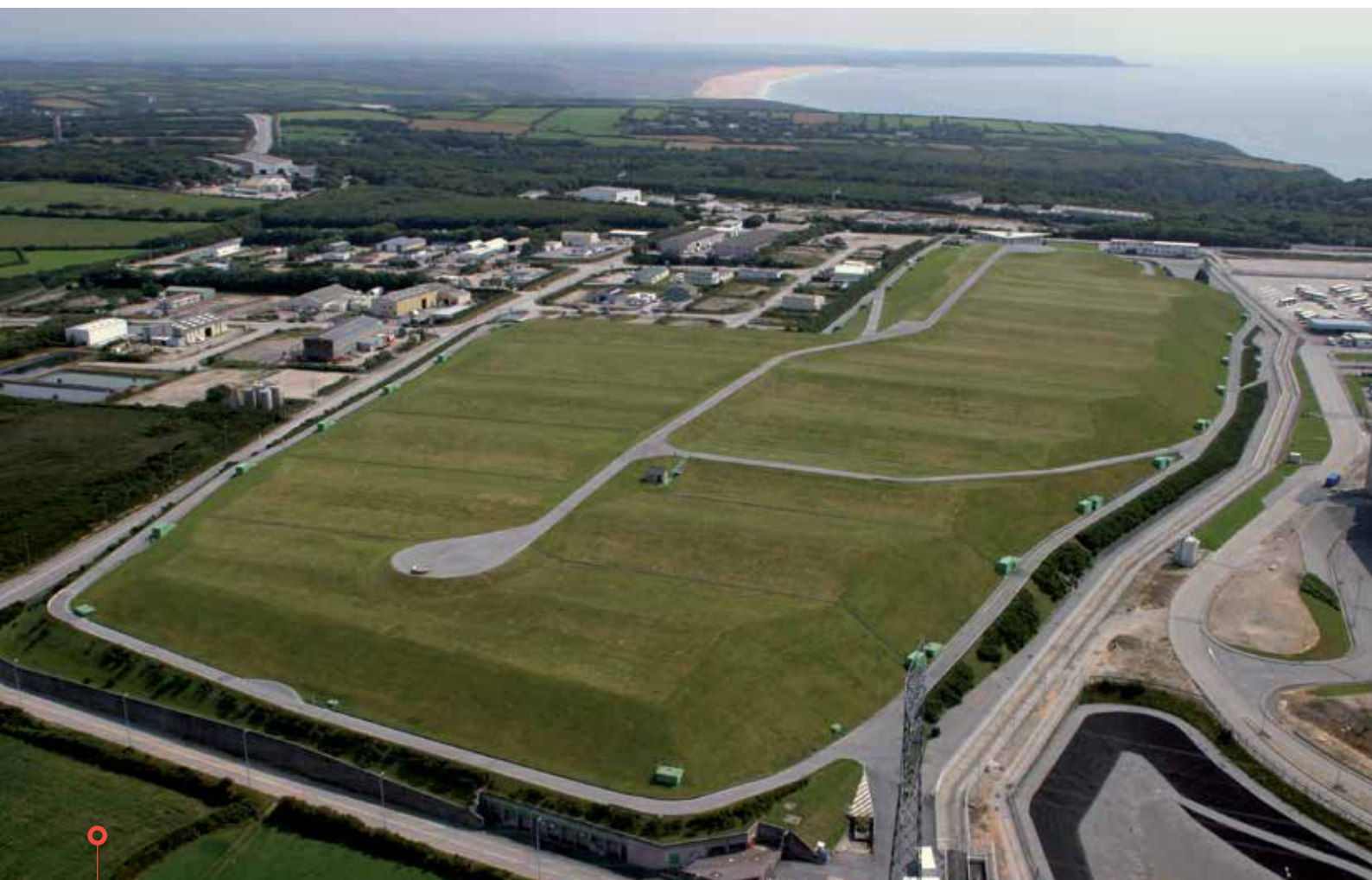
Aerial view of the CSM waste disposal facility.
