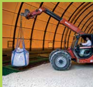
Very-low-level waste disposal
