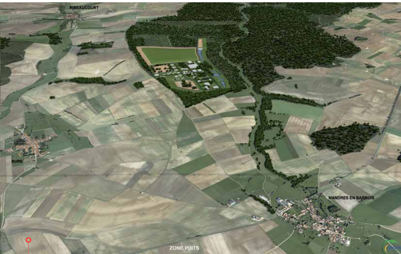
General view of the surface zone set aside for the underground work. Example according to scenario 2 mentioned on page 35.
