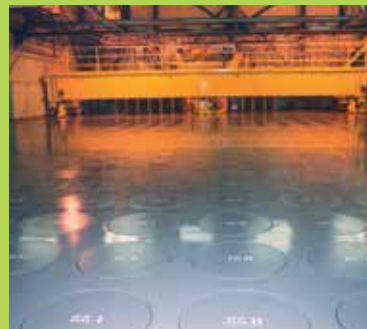
High-level waste storage
