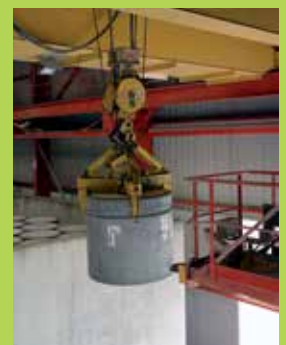
Low- and intermediate-level waste disposal
