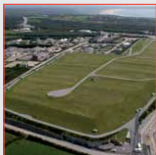
CSM waste disposal facility
