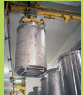
Intermediate-level, long-lived waste storage
