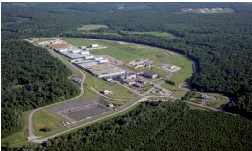
Aerial view of the CSA waste disposal facility
