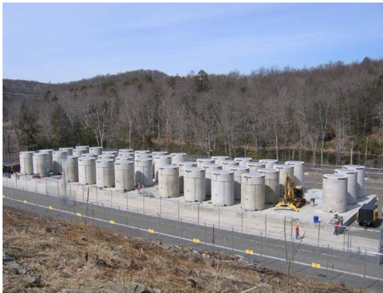
Source: DOE 2008, Connecticut Yankee's Facility
