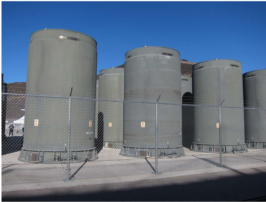
Figure 1. Holtec HI-STORM Dry Cask Storage Systems at Diablo Canyon.
