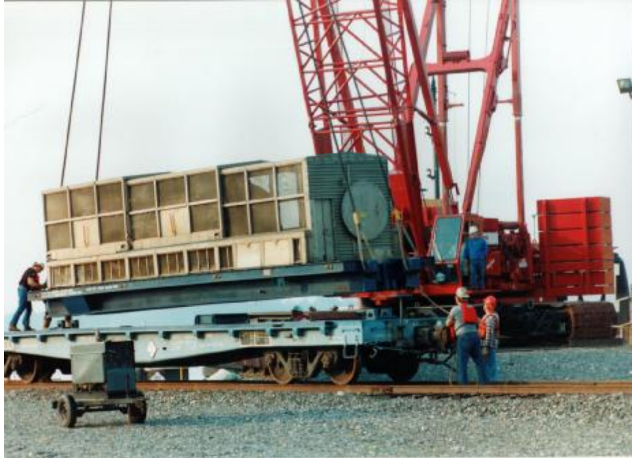
Figure 2.8 Rail-to-Truck Intermodal Transfer Facility, Valognes, France
