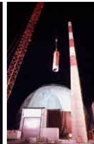
LEFT TO RIGHT: Two cranes loom over Big Rock Point’s stack, prepared for their role in the dismantlement process. A 300-foot crane holds the very top segment of the stack after it was cut free on Oct. 11, 2004. The piece was nearly 24-feet tall and weighed 30,000 pounds. Lights were installed the length of the crane to ensure it was visible to aircraft.
