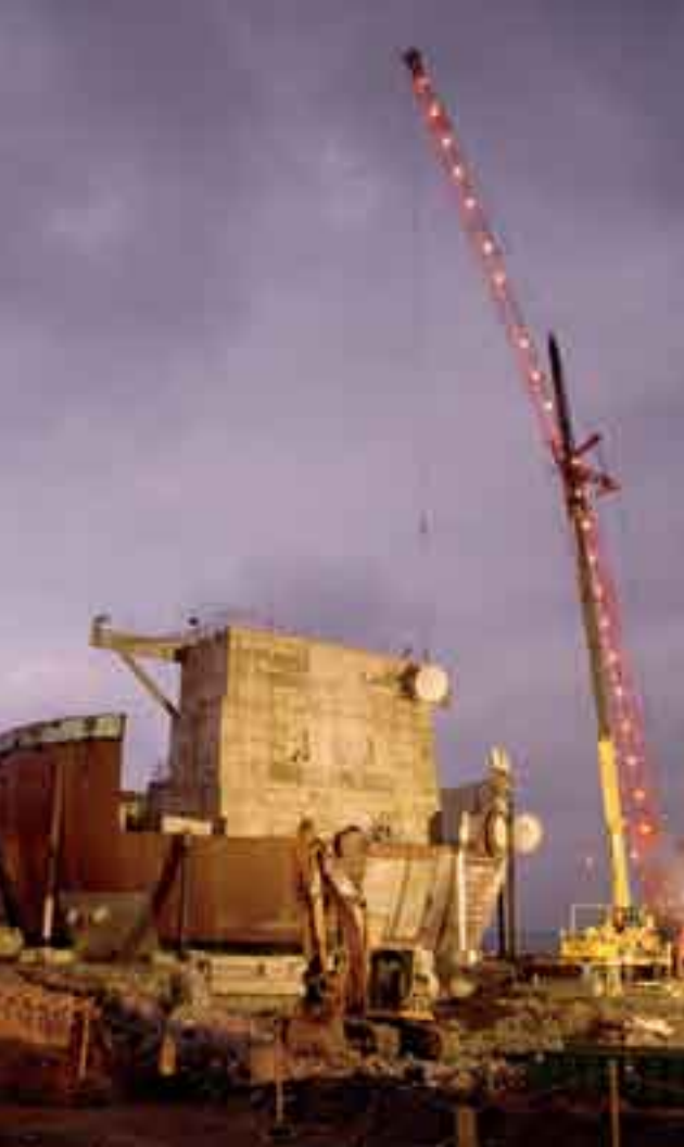
TOP: The 9,000-pound containment sphere cap was the first of 90 pieces to be removed and lowered to the ground in mid-September 2005. Some of the sections weighed up to 20,000 pounds, and the project spanned two months.
