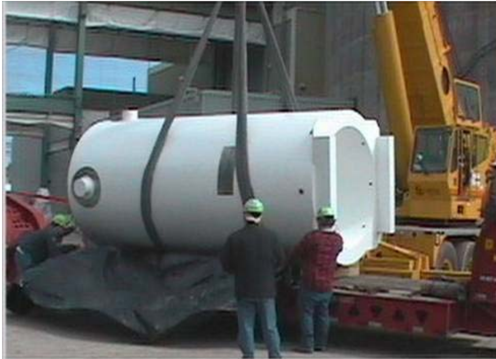
Figure 5-2 NAC Transfer Cask Body (NAC SNFDS Seminar)
