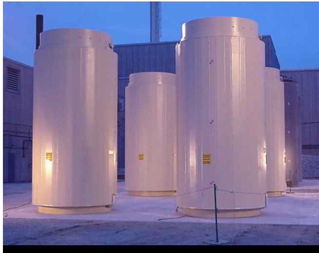
HI-STAR 100 Overpacks in Interim Storage at a Domestic ISFSI
