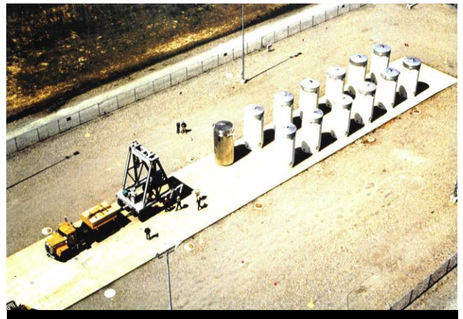
NAC I28 S/T Used Fuel Storage Cask in Place at Surry Nuclear Power Plant ISFSI
