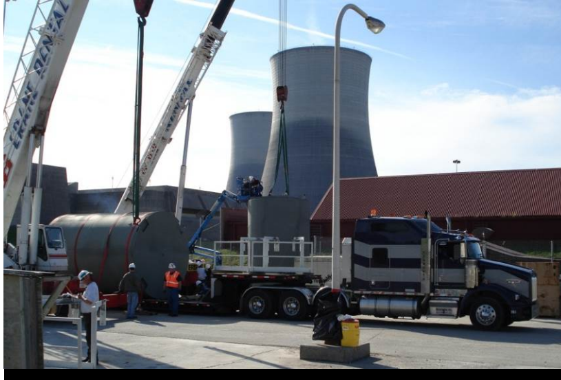
HI-STORM 100 Overpack Delivery to NPP
