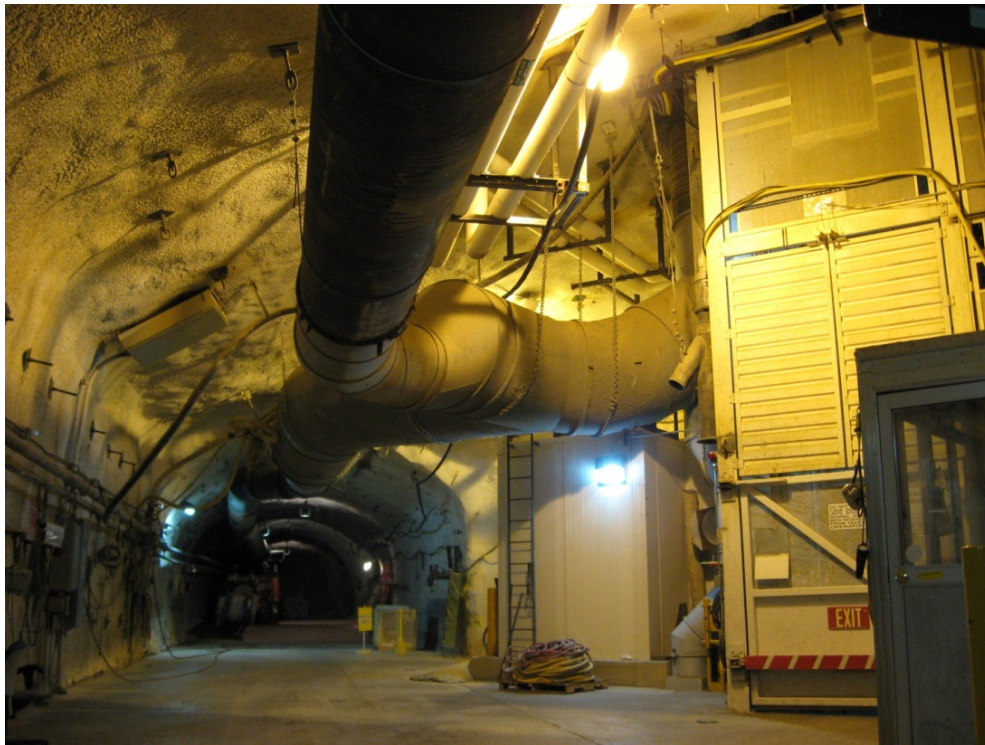
Figure B-1 Shaft Station at the Main Working Level (~300 m depth) in the U1a Underground Facility at the NNSS (photo released for unlimited use)
