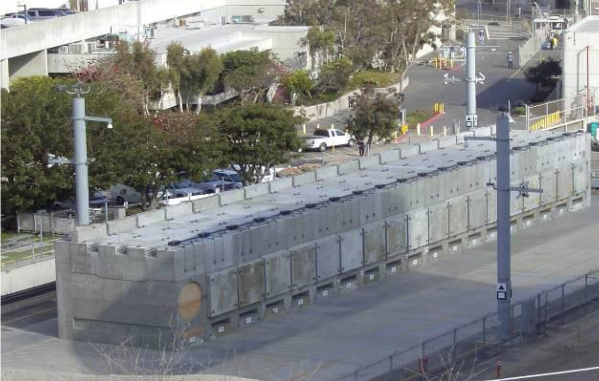
Figure V.1-1: NUHOMS horizontal dry storage systems at San Onofre.
