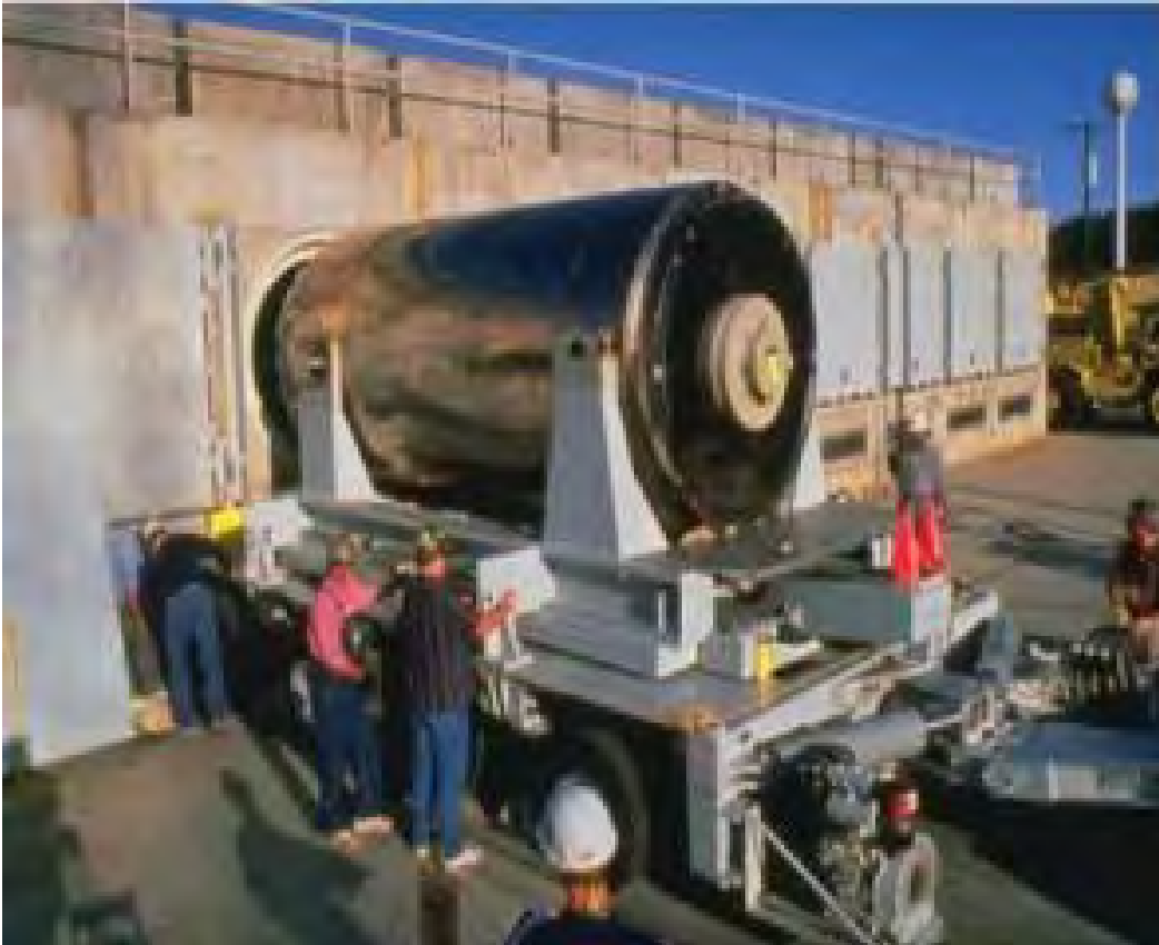
Figure 3.2-25 Transnuclear Advanced NUHOMS Storage System at the San Onofre ISFSI
