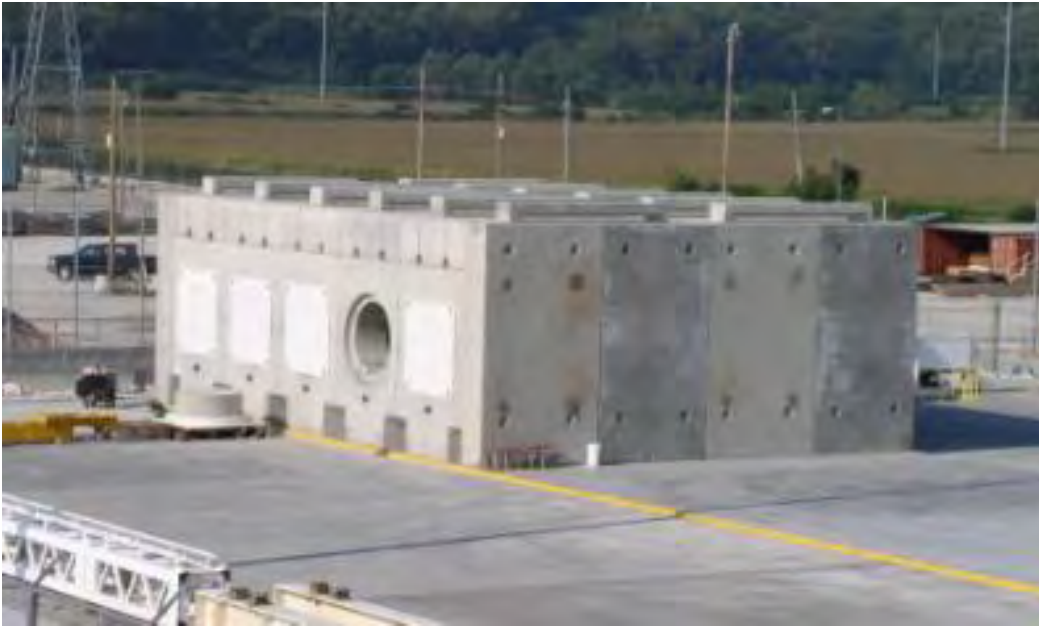
Figure 3.2-24 Transnuclear HD NUHOMS Storage System at the North Anna ISFSI
