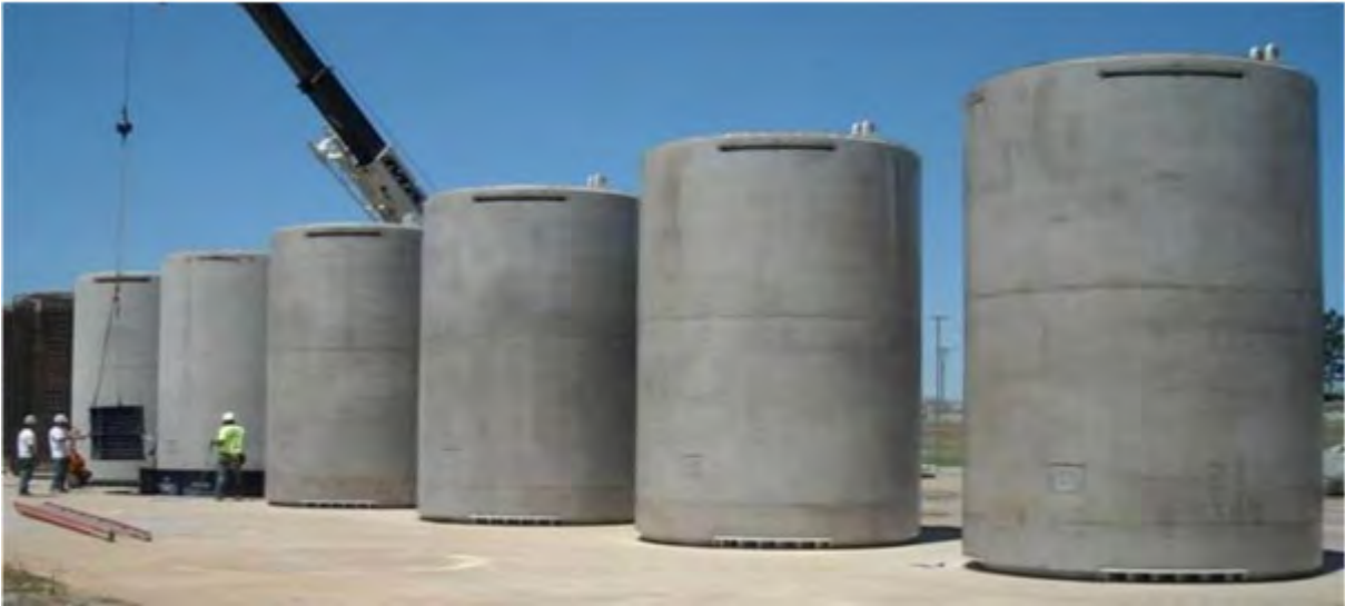
Figure 3.2-7 NAC MAGNASTOR System that will be used at the Zion ISFSI
