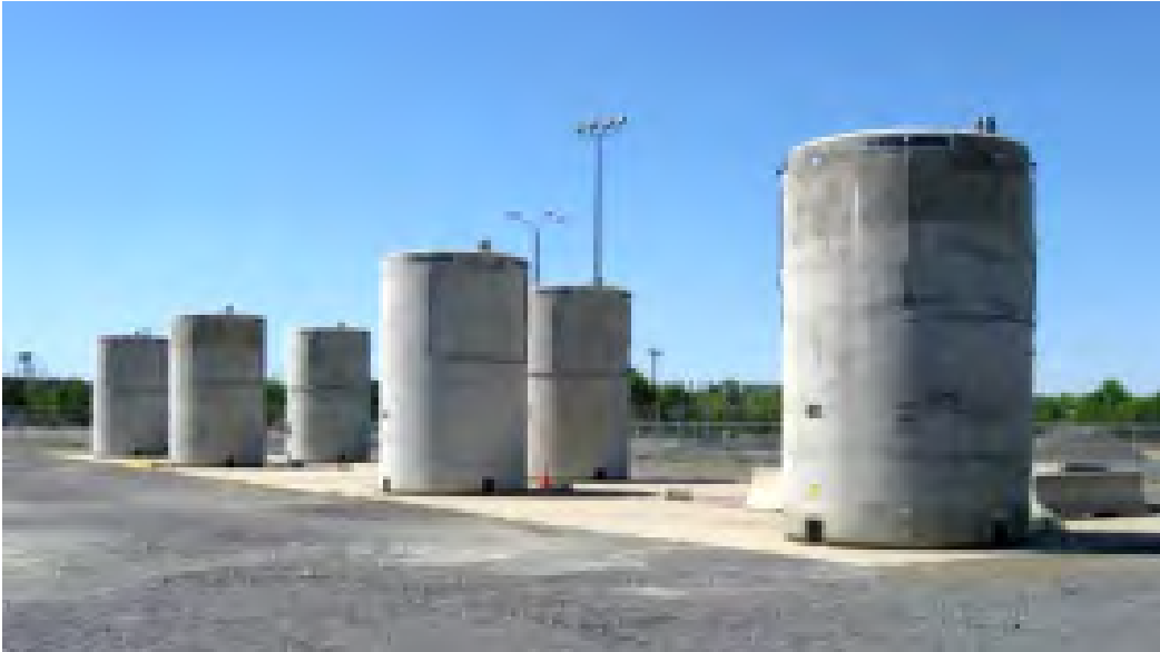
Figure 3.2-22 NAC MAGNASTOR Storage System at the McGuire ISFSI
