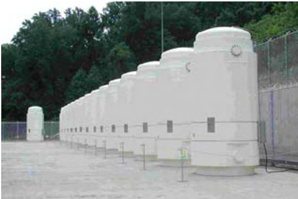
Figure 3.2-35 TN-68 at Peach Bottom
