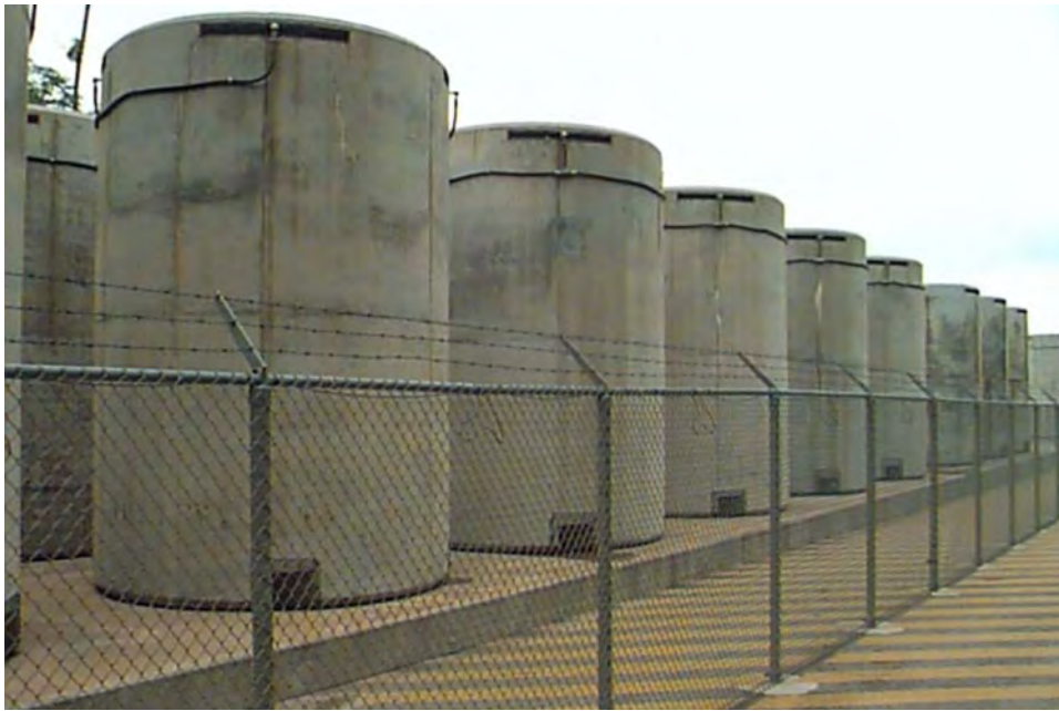
Figure 3.2-46 VSC-24 Non-Transportable Canister DFSS at Palisades
