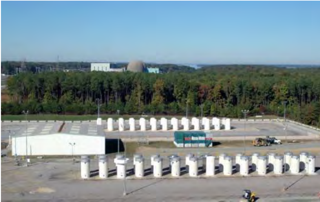
Figure 3.2-43 Castor V/21 and X/33, NAC-I28, and Westinghouse MC-10 at Surry
