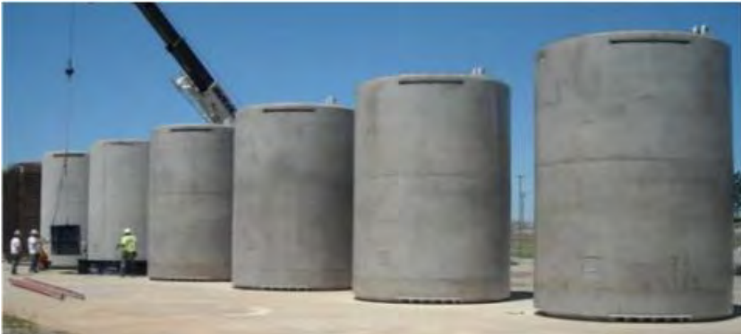
Figure 3.2-22 NAC MAGNASTOR Storage System at the McGuire ISFSI
