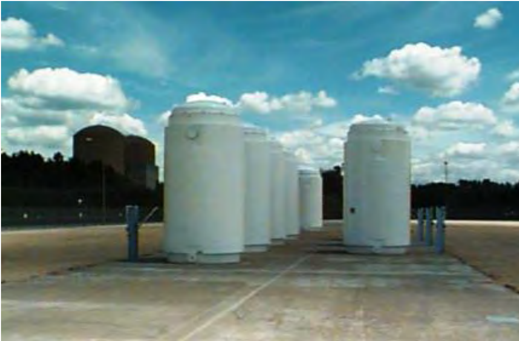
Figure 3.2-35 TN-68 at Peach Bottom
