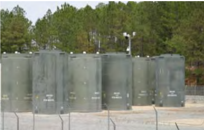
Figure 3.2-20 Holtec HI-STORM 100 Storage System at the Hatch ISFSI
