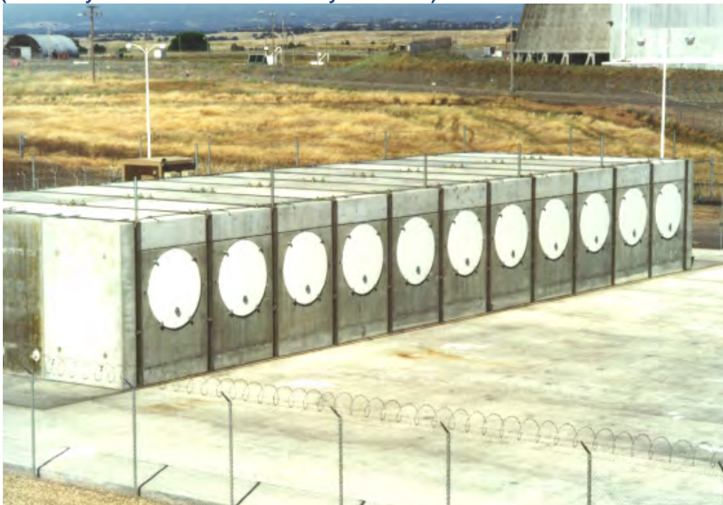
Figure 3.2-5 Transnuclear NUHOMS System at the Rancho Seco ISFSI (Similar systems at Kewaunee and Oyster Creek)
