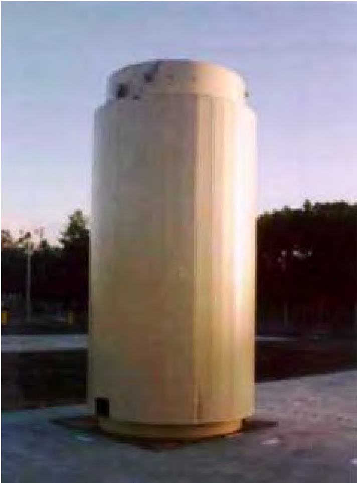
Figure 3.2-20 Holtec HI-STORM 100 Storage System at the Hatch ISFSI
