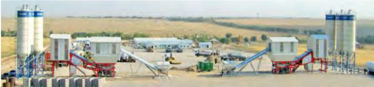
Figure 3.2-28 Typical Dual-Batch Plant Arrangement
