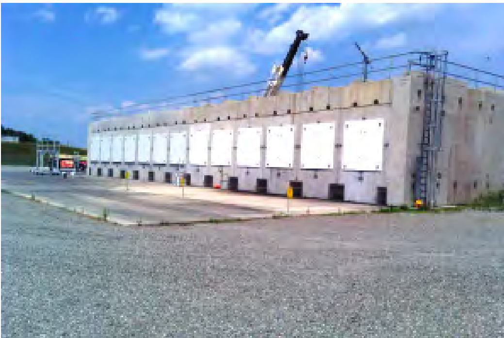
Figure 3.2-24 Transnuclear HD NUHOMS Storage System at the North Anna ISFSI
