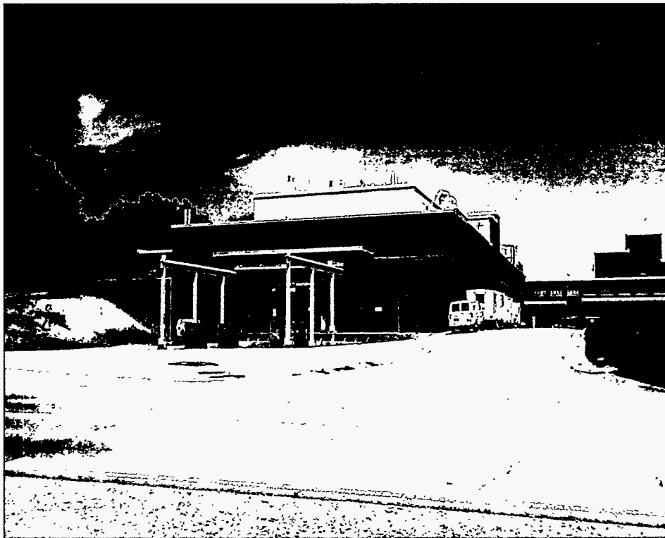
FIGURE 2.1 Photograph of M-Wing, Building 200 (17551 K)
