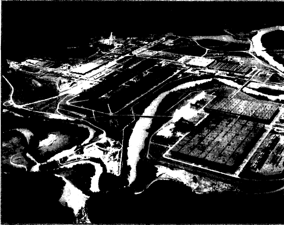
The Oak Ridge Gaseous Diffusion Plant was the first gaseous diffusion plant to produce HEU. Ultimately, there were five process buildings at the plant that were interconnected to form one long, continuous cascade.
