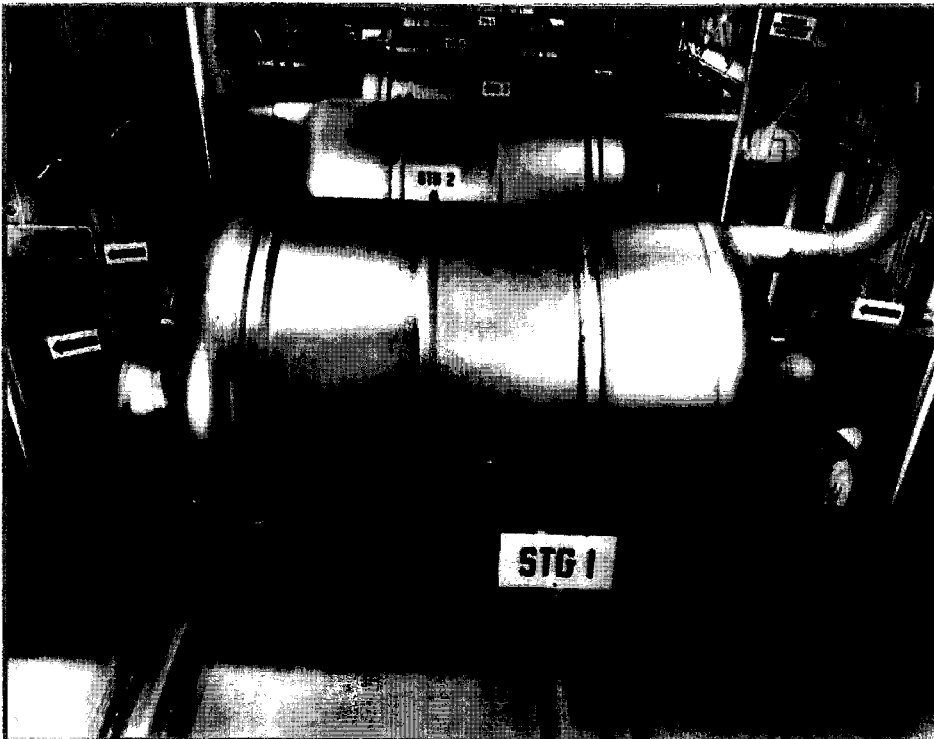
To enrich uranium using the gaseous diffusion process, uranium hexafluoride gas must be cycled and recycled through various stages of equipment, such as the arrangement at the Oak Ridge Gaseous Diffusion Plant (ORGDP). By the mid-1950s, the ORGDP had approximately 5,000 stages capable of furnishing a top product of 93 percent uranium-235.
