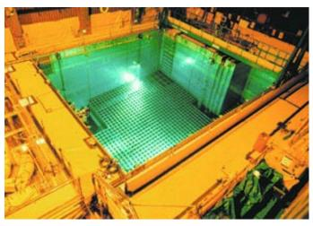
Figure 2. Typical Used-Fuel Storage Pool
