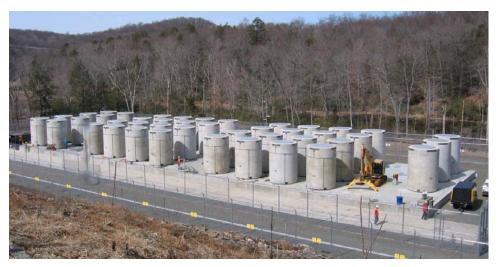
Figure 3. Independent Spent-Fuel Storage Installation
