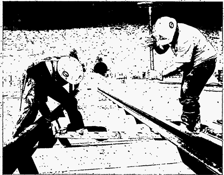
Layin' 'em in and tyin' 'em down... Workers run a track for muck cars into the TBM starter tunnel. Current TBM technology is a combination of the latest developments and standards such as railroad tracks, which are used when appropriate.
