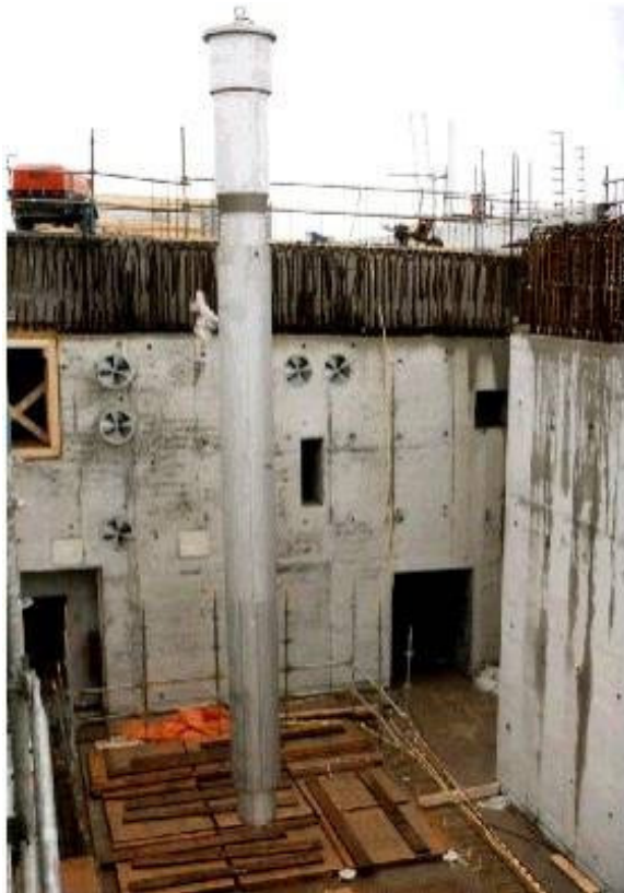
Figure A.4. Placement of the wells during construction
