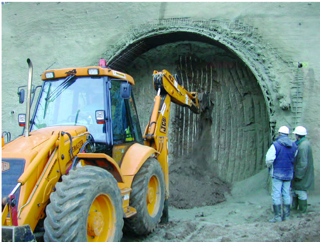
Figure 11.3. Excavation of the double incline
