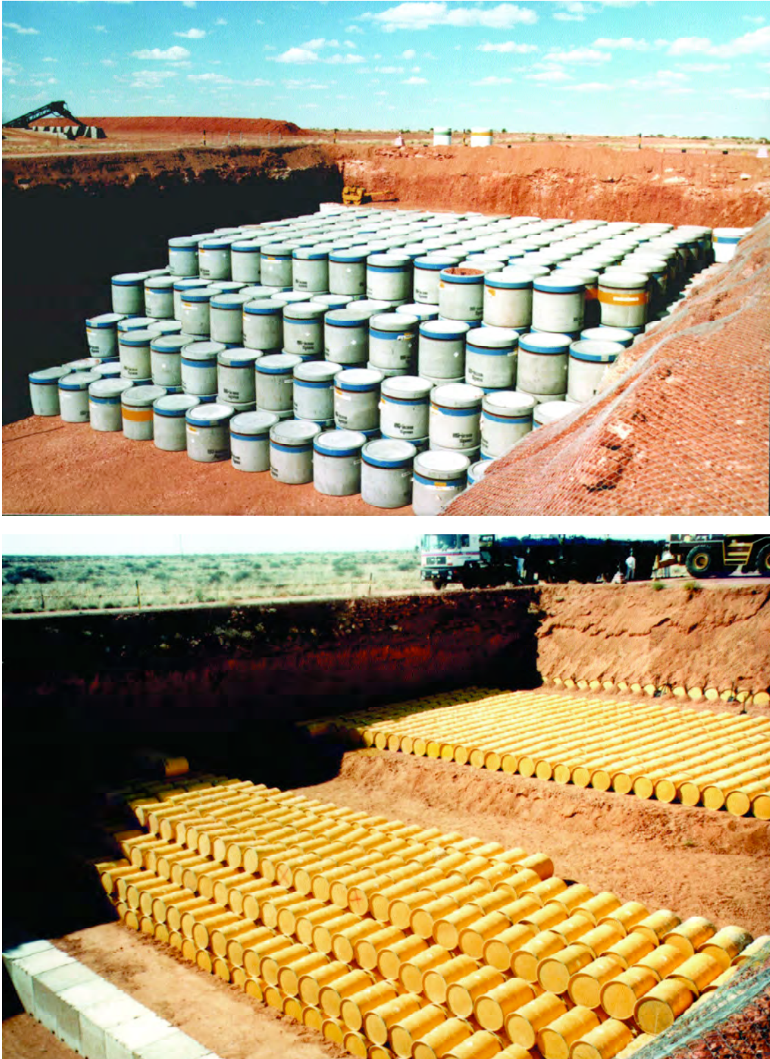
Figure 20.4. Waste disposal practices at Vaalputs: the intermediate (top) and low-level waste (bottom) trenches at Vaalputs before their filling and planned closure in 2005
