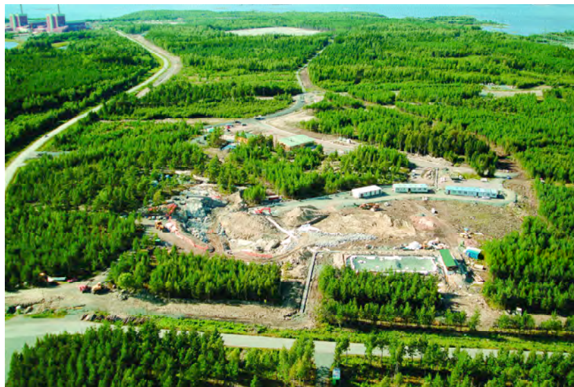
Figure 8.4. A general view of the ONKALO site in March 2005
