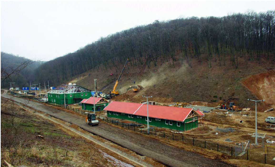
Figure 11.2. Preparations for the underground explorations
