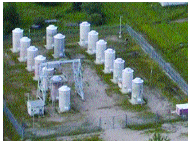
Figure 5.6. Concrete silos at the Whiteshell Laboratory in Manitoba
