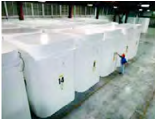
Figure 5.5. Dry storage container at the Pickering Waste Management Facility in Ontario
